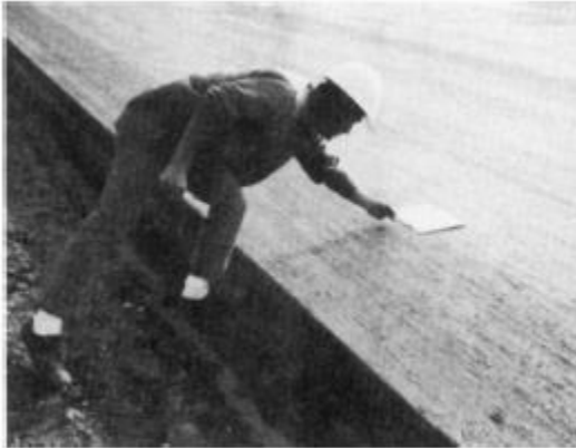
Figure A.9: CT535 Absorbent Pad Placement (CalTrans 2014).
