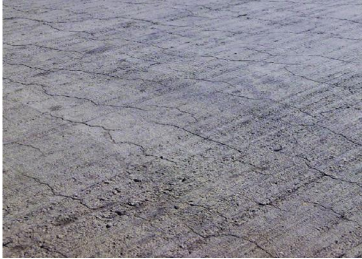
Figure A.1: Pavement plastic shrinkage cracks (Sayahi, 2019)
