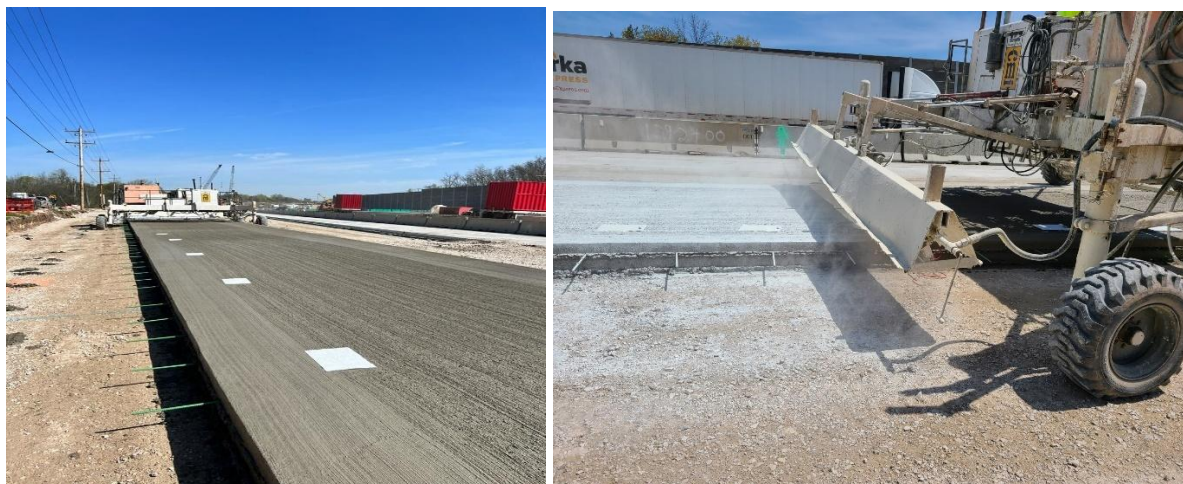
Figure 16. Caltrans CT 535 set-up. (Left) absorbent pads before curing compound application (Right): Absorbent pads after curing compound application.
