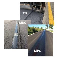
membrane; Methods and Materials Post-Construction (MPC) includes processes and materials used immediately following construction, before joint deterioration requires extensive structural repair or replacement, such as fog sealing and spraying penetrating asphalt emulsions on the joint following construction.
