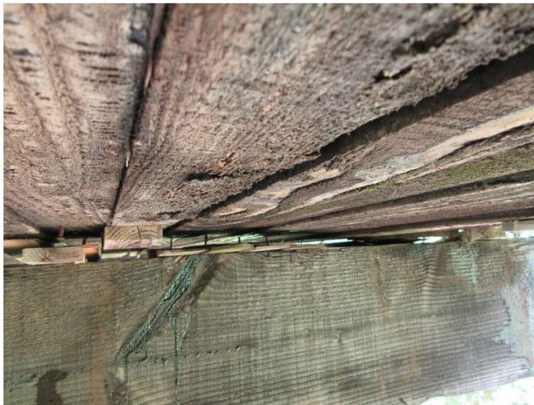
**Figure 4-52 Missing shims or gapping between spreader beam and bottom side of deck (La Crosse Co. P320083)**
