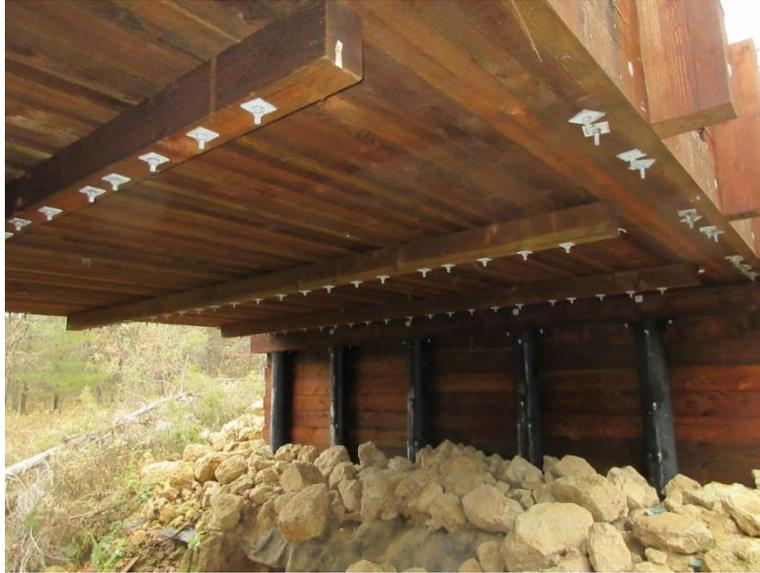
**Figure 4-48 Monroe County Bridge B410315 Spreader Beams**
