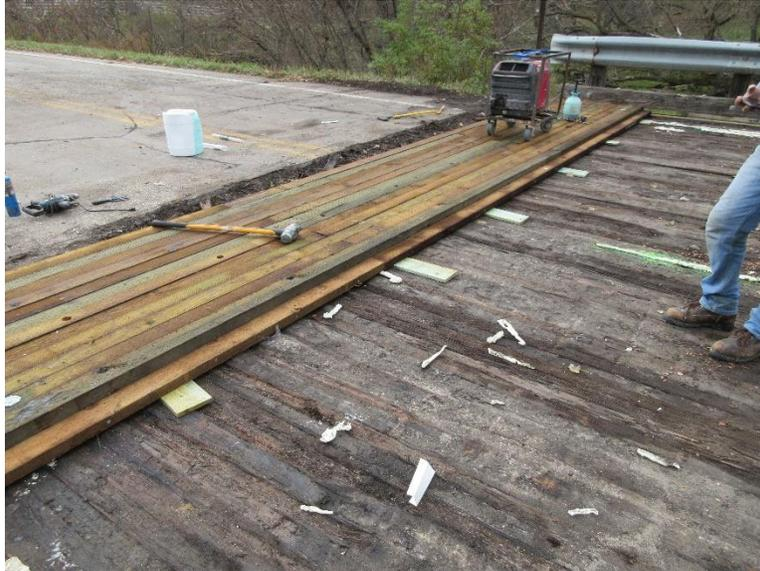
**Figure 4-35 Transverse Timber Slab Retrofit under Construction**
