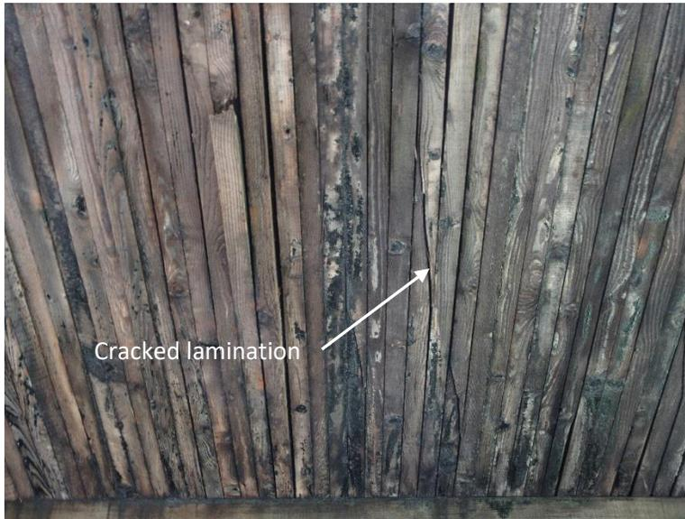
**Figure 4-54 Cracked Lamination (La Crosse Co. P320083)**
