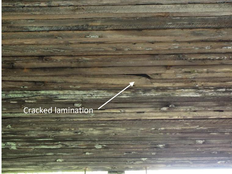
**Figure 4-53 Cracked Lamination (La Crosse Co. P320083)**
