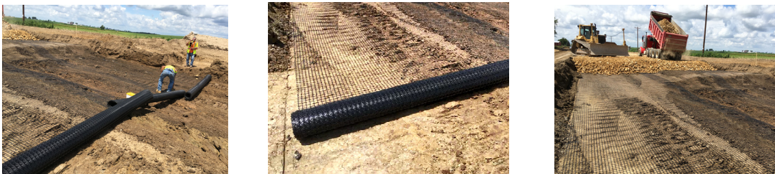
Figure 1.1: Use of geogrid in Wisconsin pavements – STH 33 between Cashton and La Crosse, WI (Pictures by Titi, 2016)
