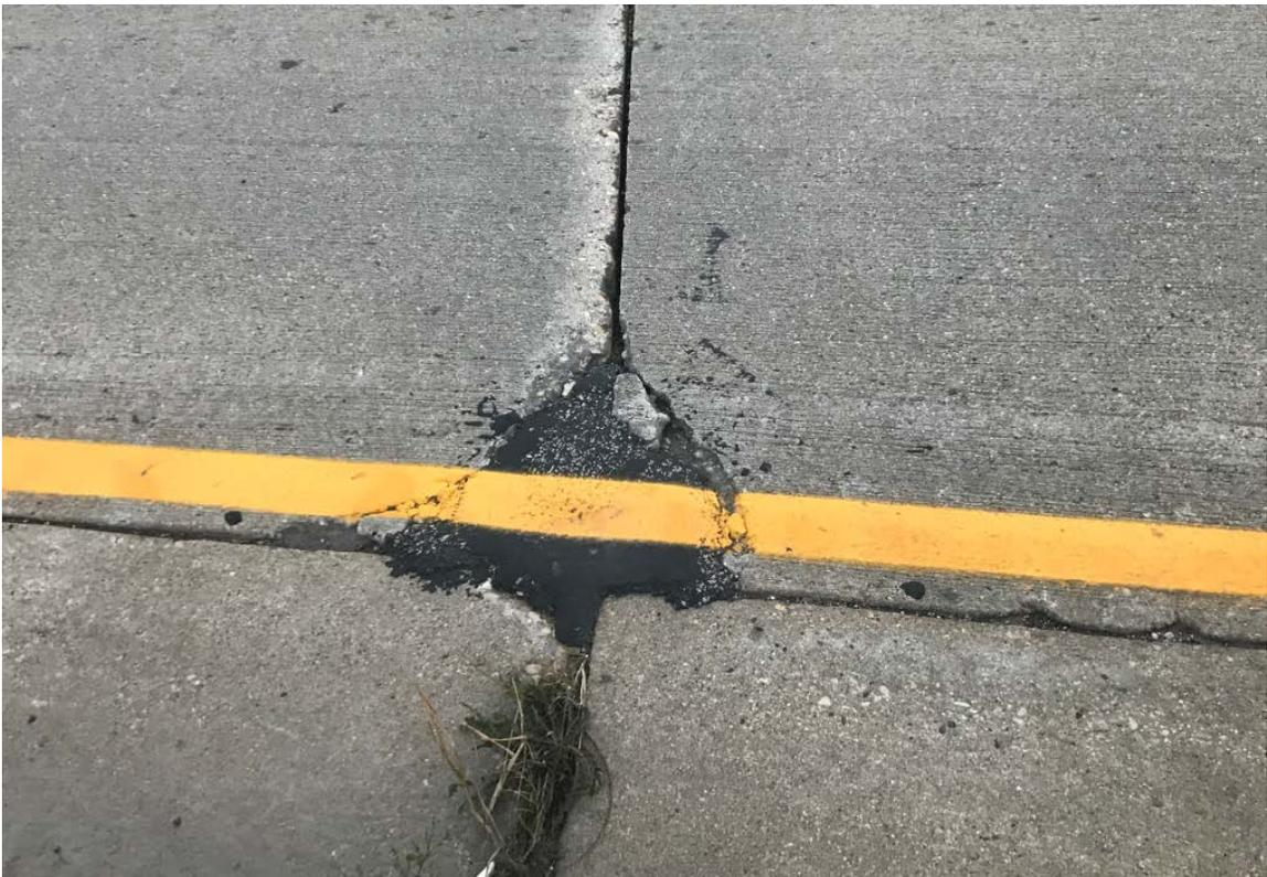
Figure F-7. Existing pavement deteriorating around PDR
