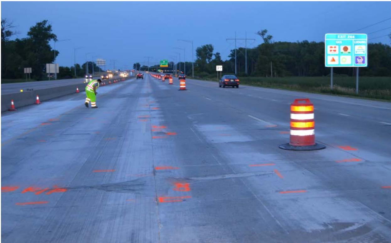
Figure B-11. Workzone—areas being marked for full-depth repairs
