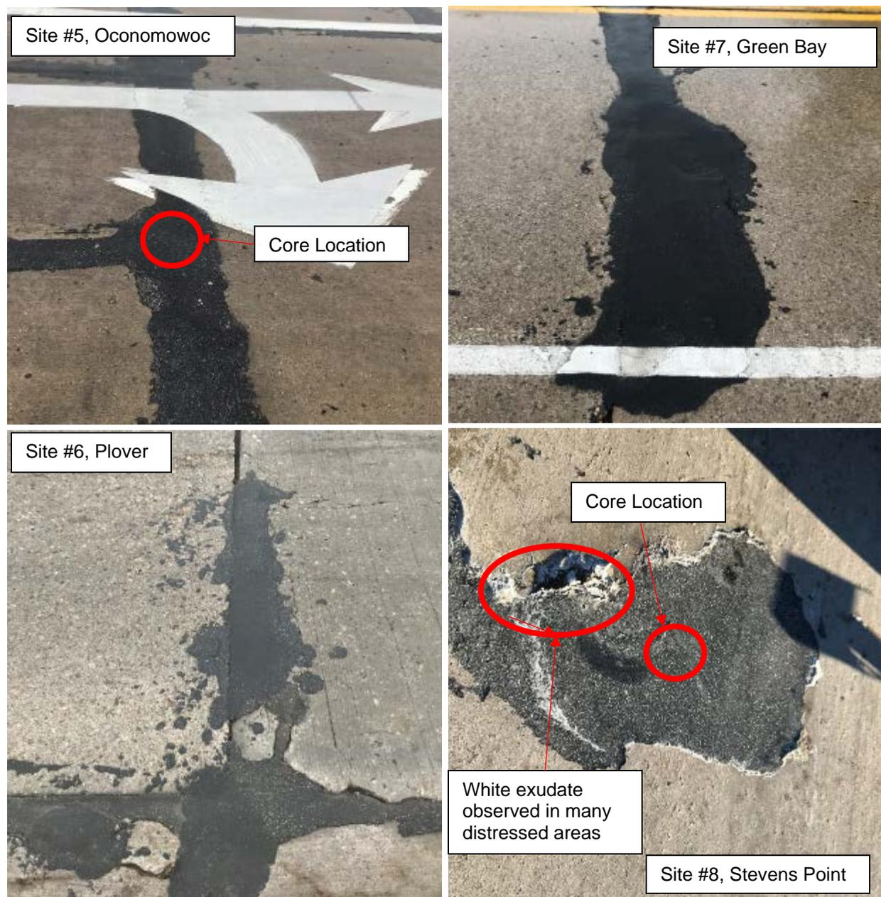
Figure 3-13. RM-3 used in concrete pavement PDR applications.
