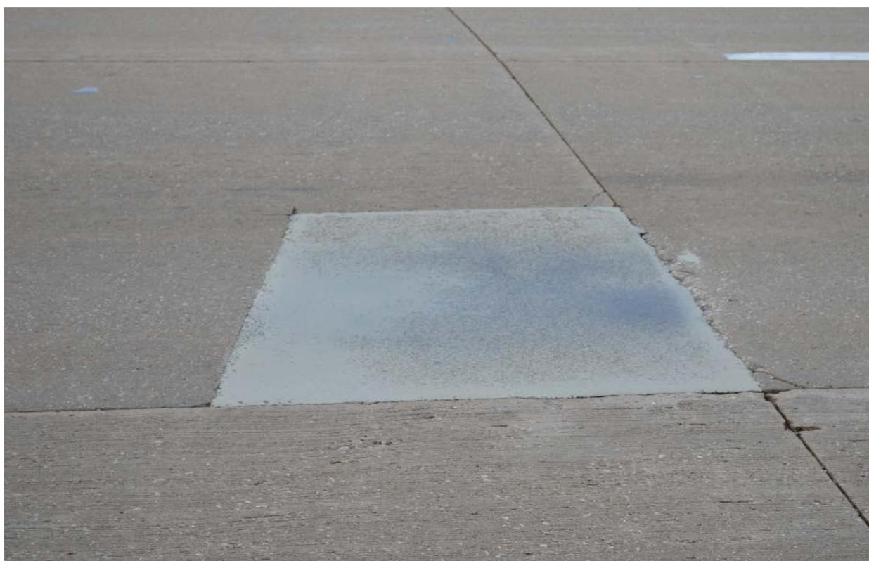
Figure E-27. PDR to address an isolated area of distress in an otherwise distress free pavement (Site #17, W. Johnson St., Fond du Lac).
