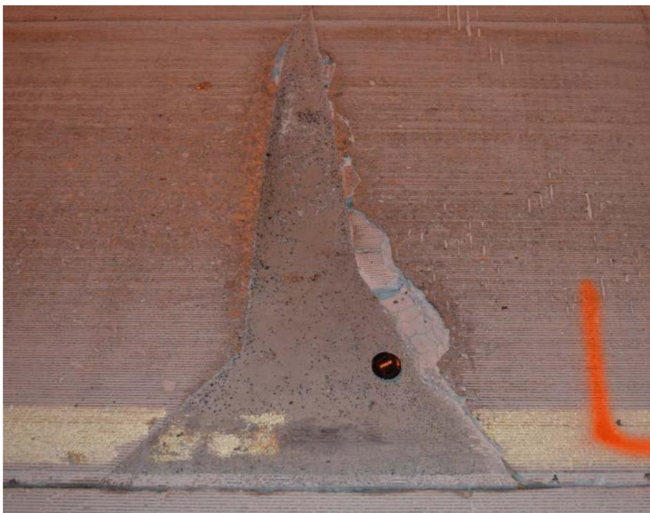
Figure B-6. RM-1 PDR (6)—deterioration along patch edges
