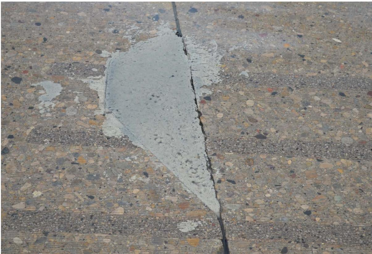
Figure E-15. PDR to address spalling at a transverse joint (Site #12, US 41, Marinette).
