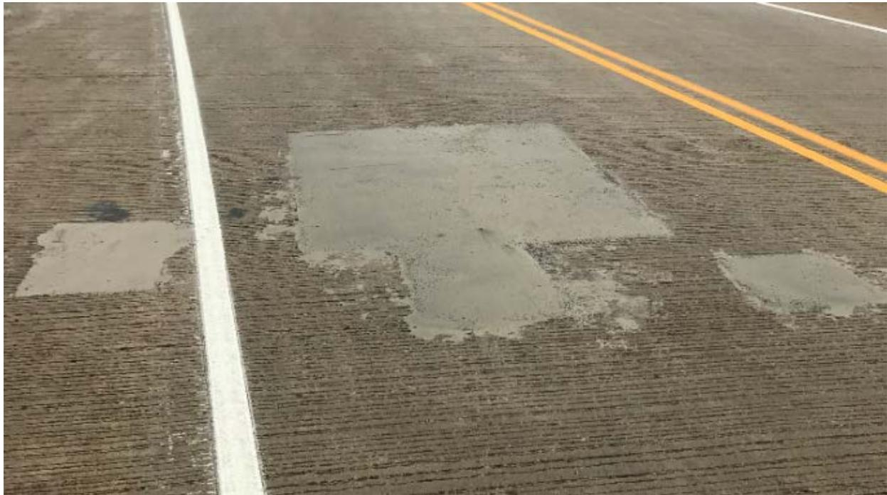
Figure E-18. PDRs on bridge deck (1)
