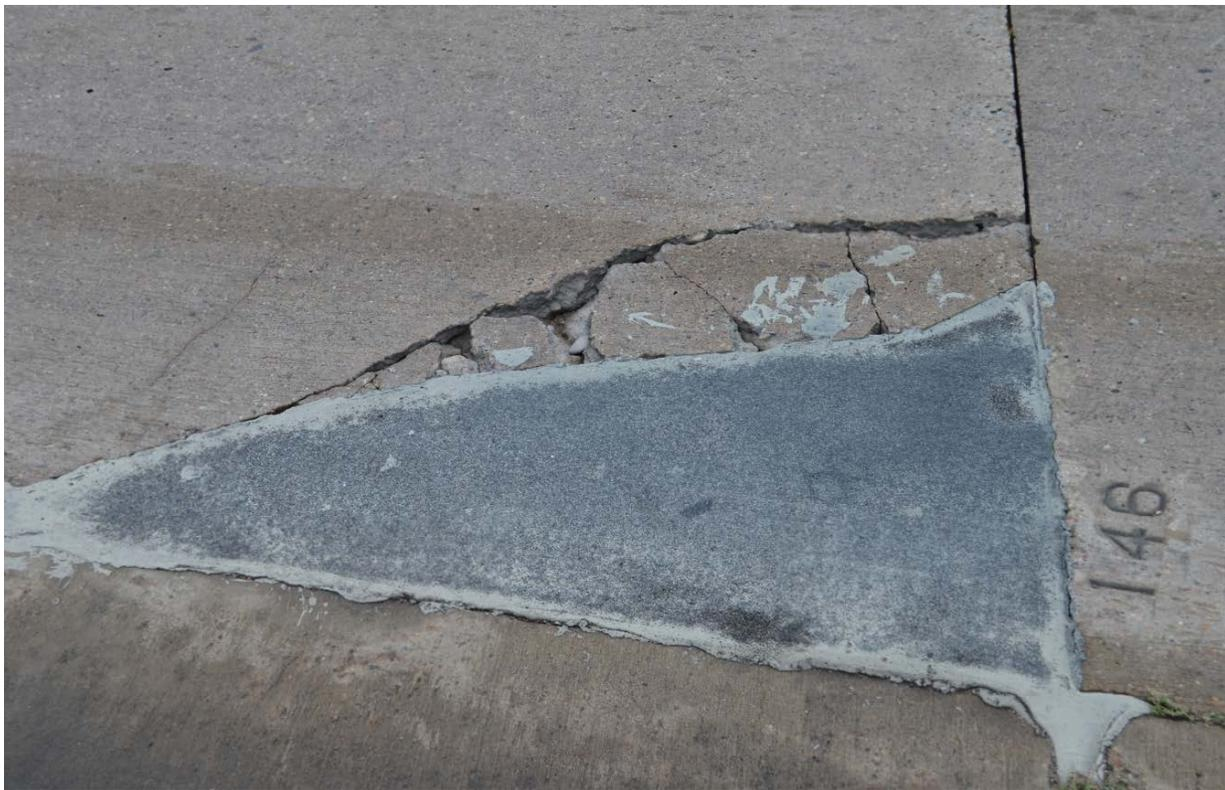
Figure E-8. Concrete pavement deterioration around PDR
