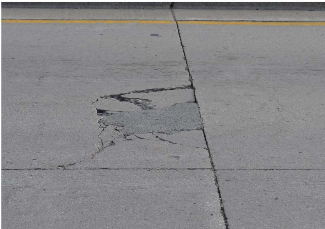
Figure E-6. Concrete pavement deterioration around PDR
