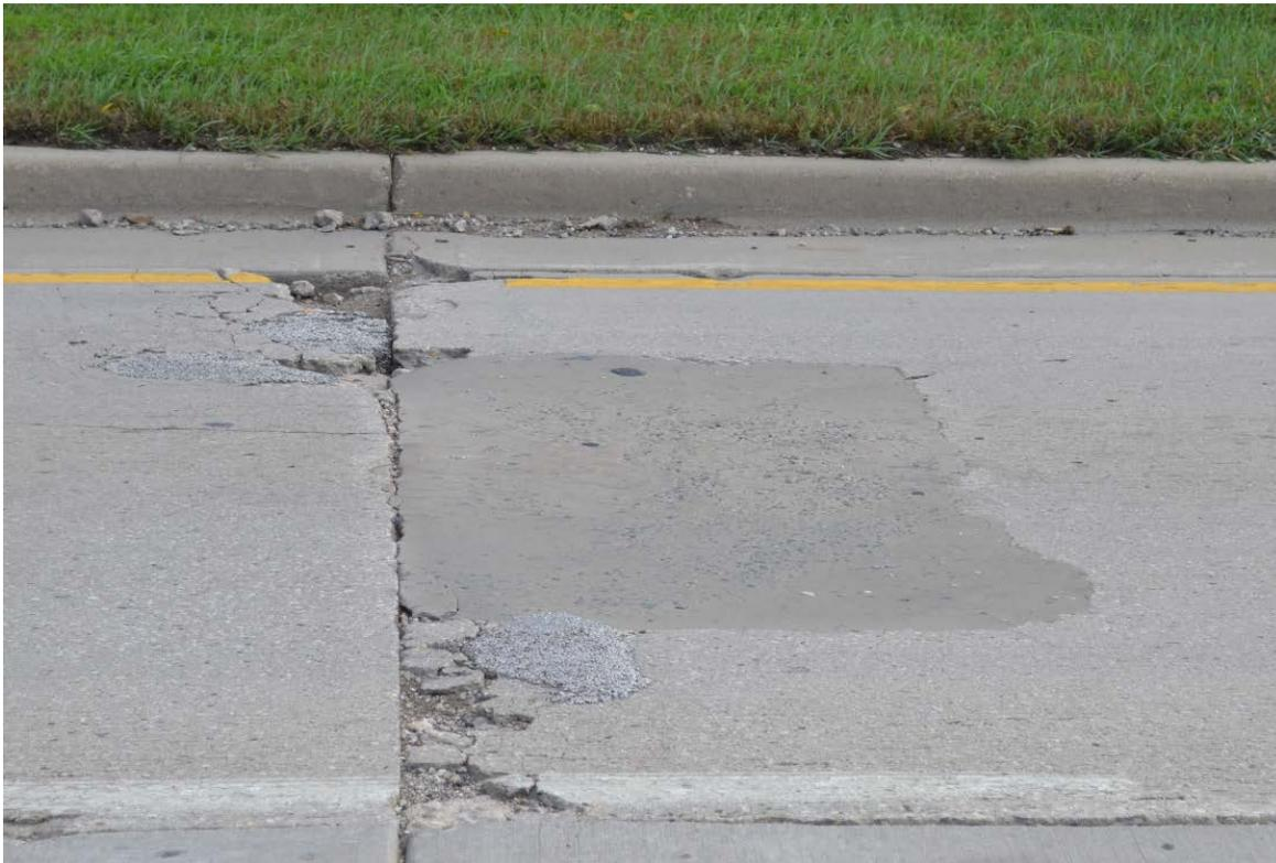
Figure E-5. Concrete pavement deterioration adjacent to PDR
