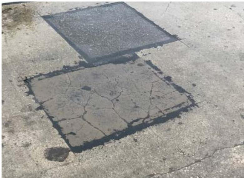
Figure 3-21. Surface map cracking pattern observed on some RM-4 PDRs on Site #16.
