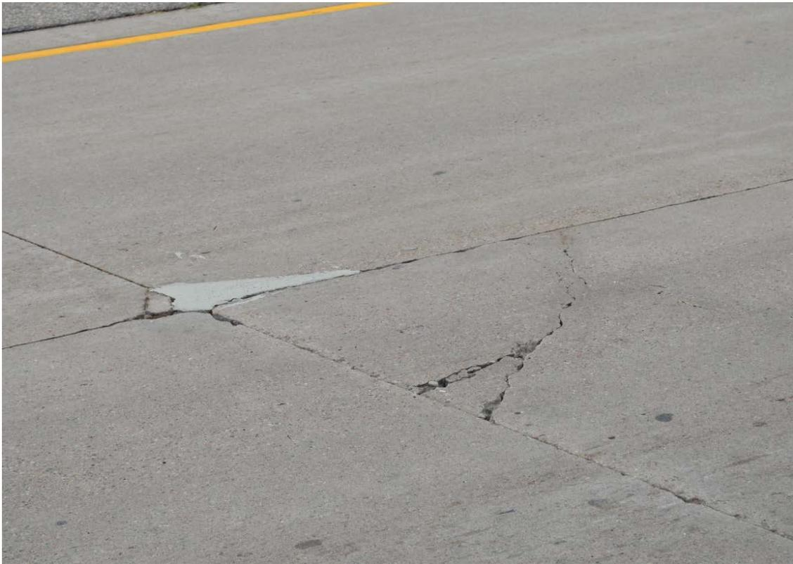
Figure E-12. Corner break in existing concrete pavement (Site #11, US 10, Stevens Point).
