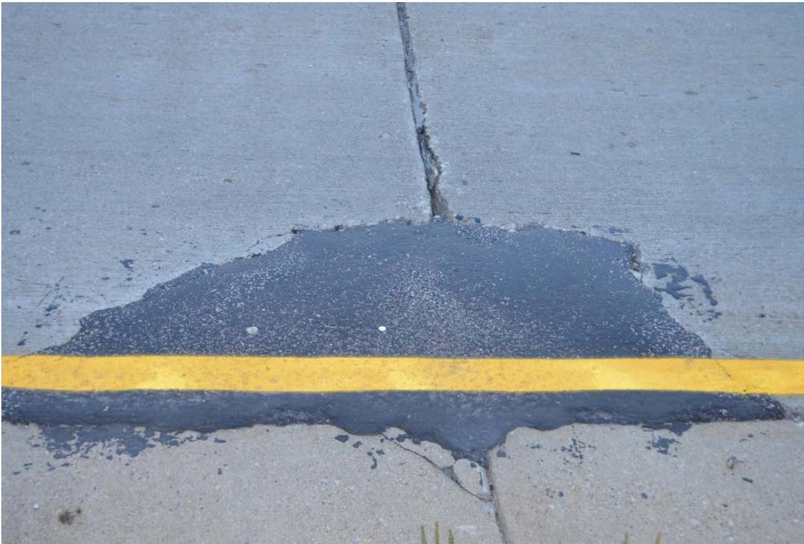
Figure F-6. PDR to address corner spalling
