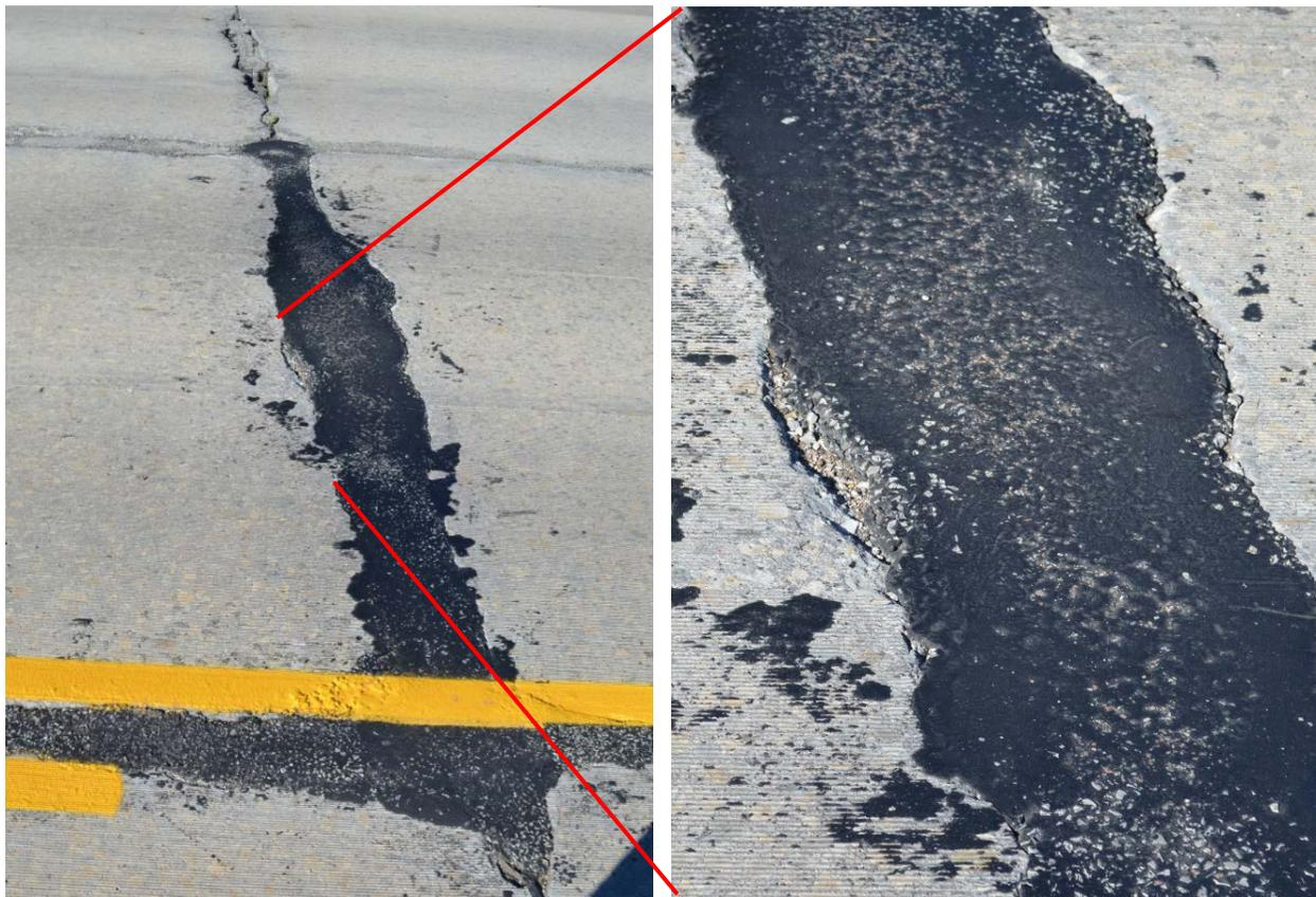
Figure F-9. PDR to address deteriorated joint (left) and existing pavement deteriorating around PDR (right) (Site #22, N. Ballard Rd., Appleton).
