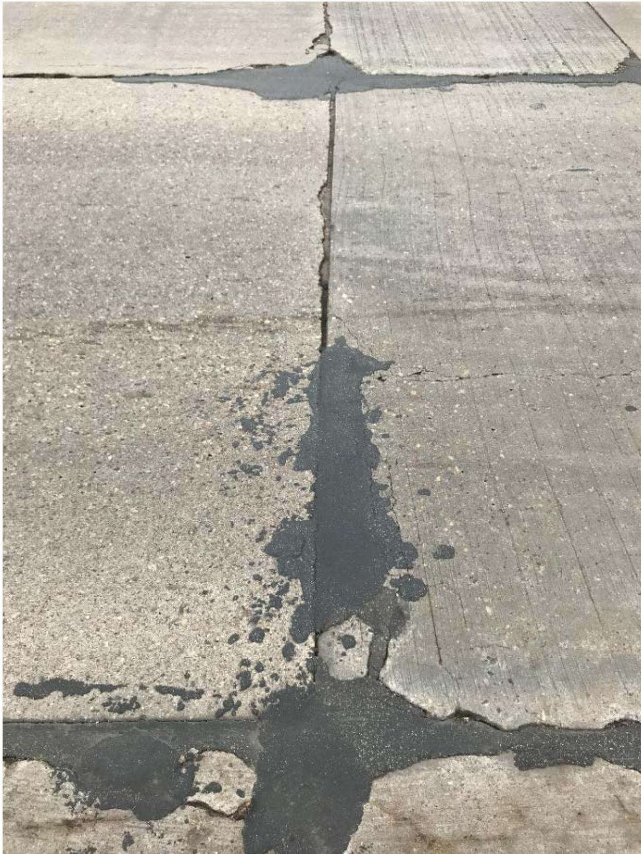
Figure D-2. PDRs to address spalling and deteriorated joints (P Site #6, lower Rd., Plover).
