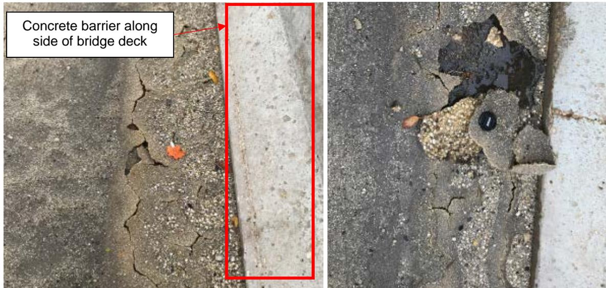
Figure 3-12. Top one-third of the RM-2 overlay peeling off along the deck edge (Site #3).
