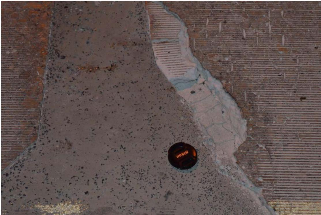
Figure B-7. RM-1 PDR (6)—close-up of deterioration along patch edge (Site #1, US 12/18, Madison Beltline).
