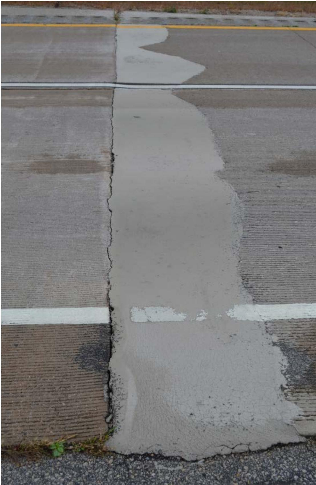
Figure E-21. PDR on bridge deck approach slabs, surface map cracking in shoulder area (Site #14, US 141, Pound).
