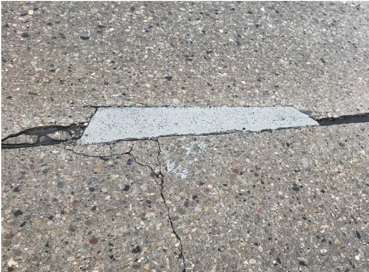
Figure E-16. Concrete pavement deteriorating around the PDR
