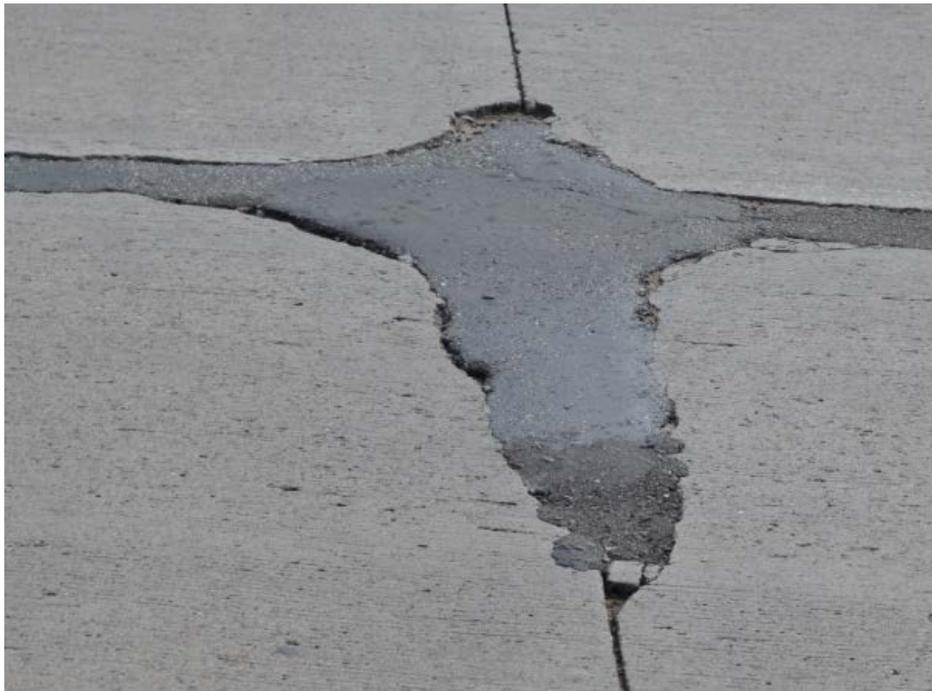
Figure F-13. PDR to address joint deterioration (Site #23, W. Kemp St., Rhinelander).
