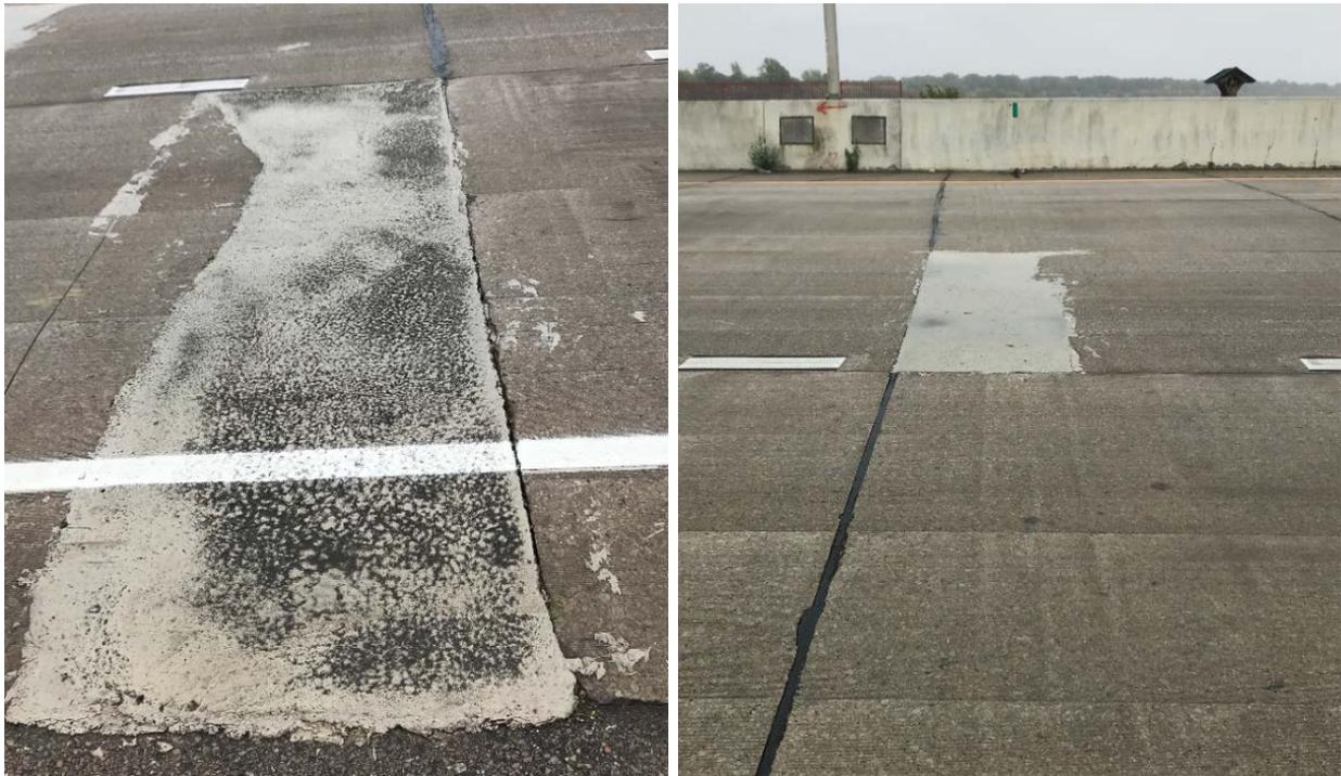
Figure E-28. PDR to address deterioration along transverse joints
