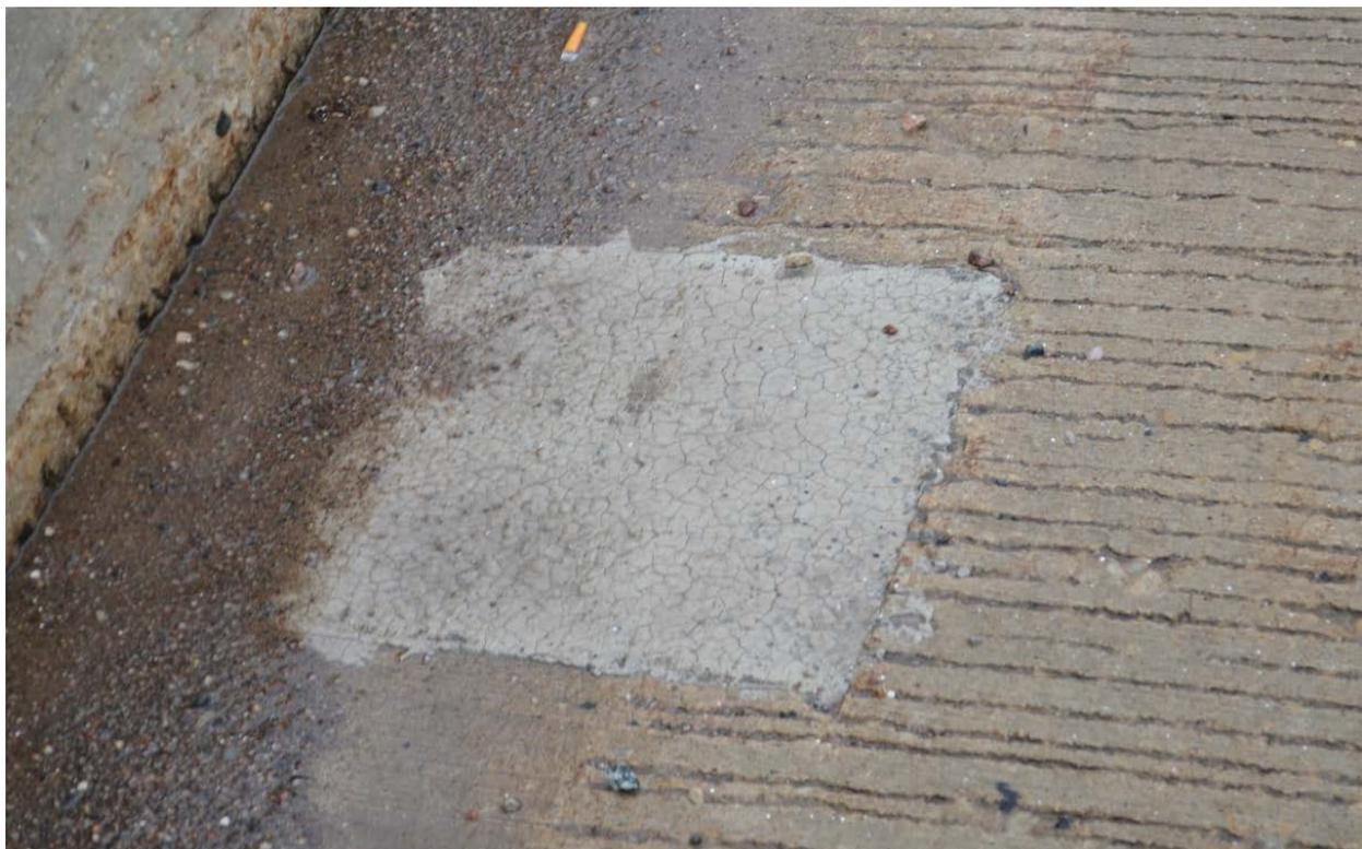
Figure E-19. Map cracking pattern on PDR surface
