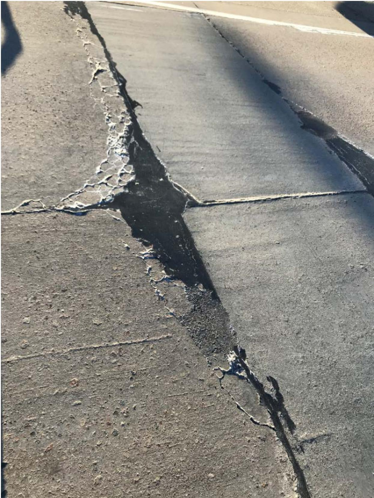
Figure D-8. D Cracking and full-depth repairs in existing concrete pavement (Site #8, State Road 66, Stevens Point).
