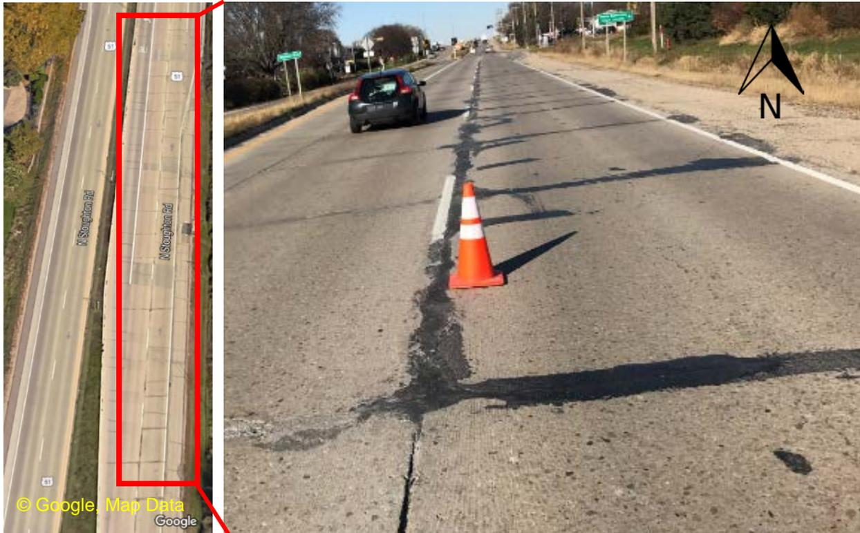
Figure 3-23. Overview of US 51/N. Stoughton Rd northbound lanes(top) and satellite imagery showing severely distressed condition of the north bound lanes.
