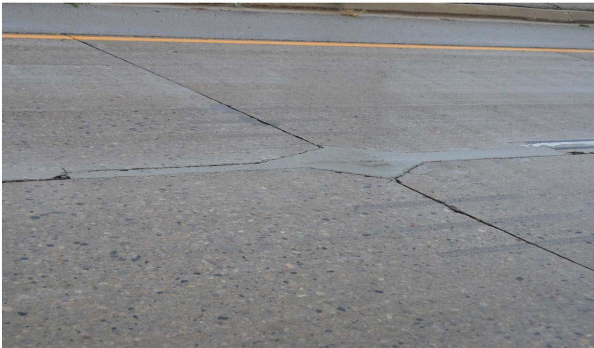
Figure E-17. PDR used to address deteriorated longitudinal joint
