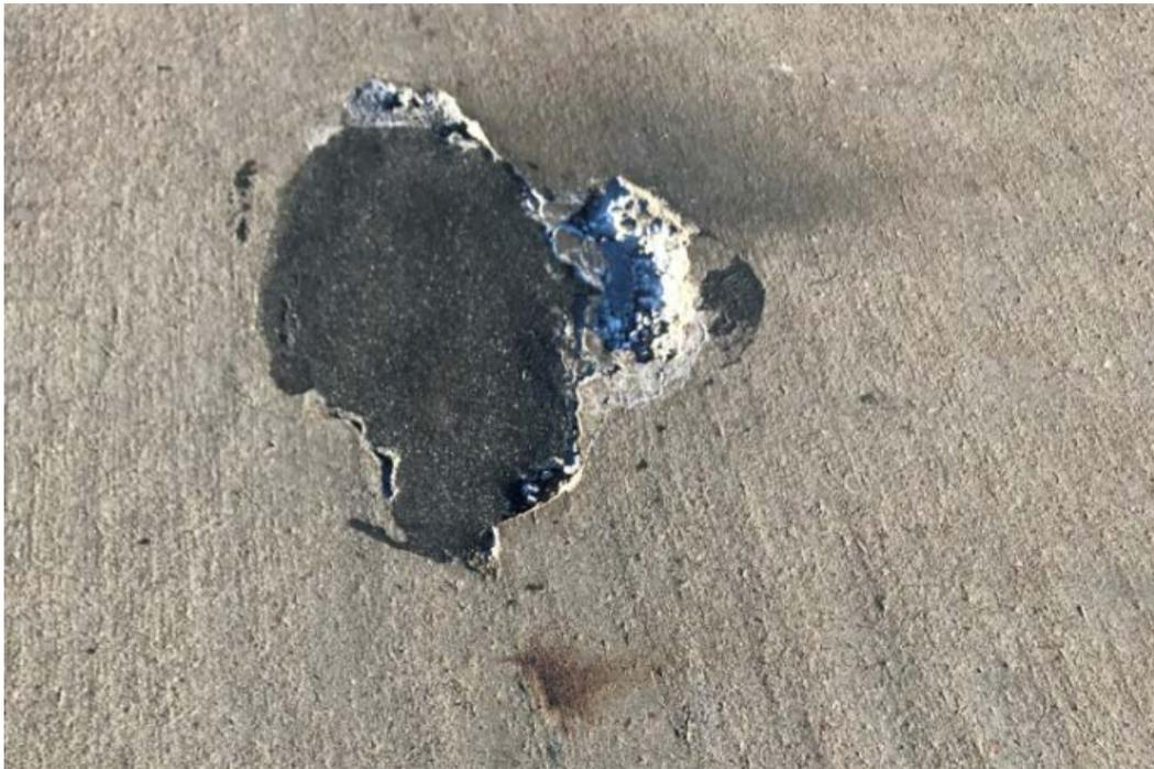
Figure D-9. Small spot repairs in slab interior
