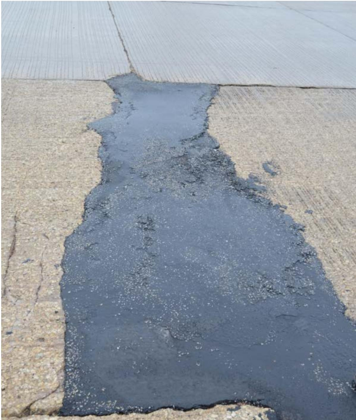
Figure F-1. PDR to address deterioration along transverse joint (Site #19, State Road 93, Eau Claire).
