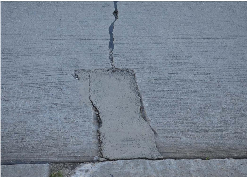
Figure E-4. Material loss along edges of a small PDR
