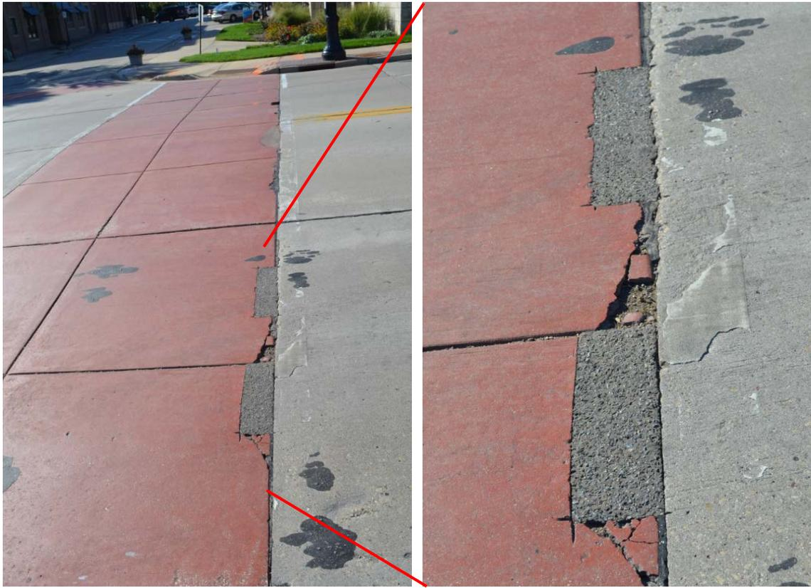
Figure E-1. PDRs along transverse joint
