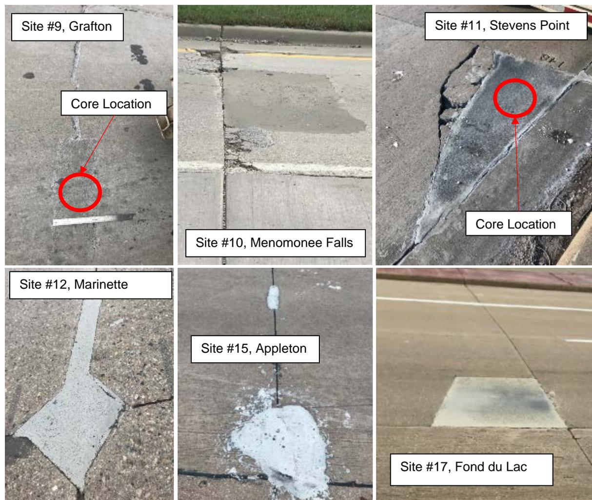
Figure 3-16. RM-4 used in concrete pavement PDR applications.
