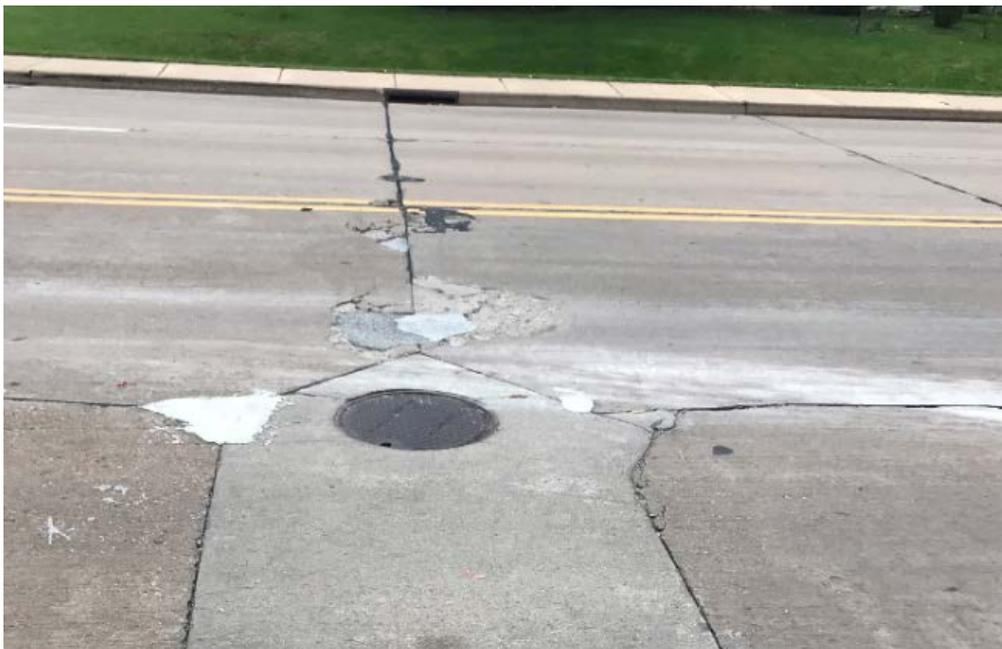
Figure E-23. Existing concrete pavement deteriorating around PDRs (Site #15, Calumet St., Appleton).
