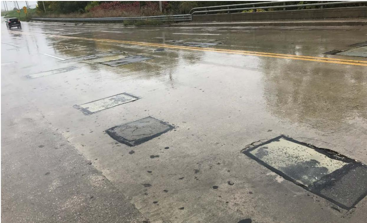
Figure E-24. PDRs on bridge deck
