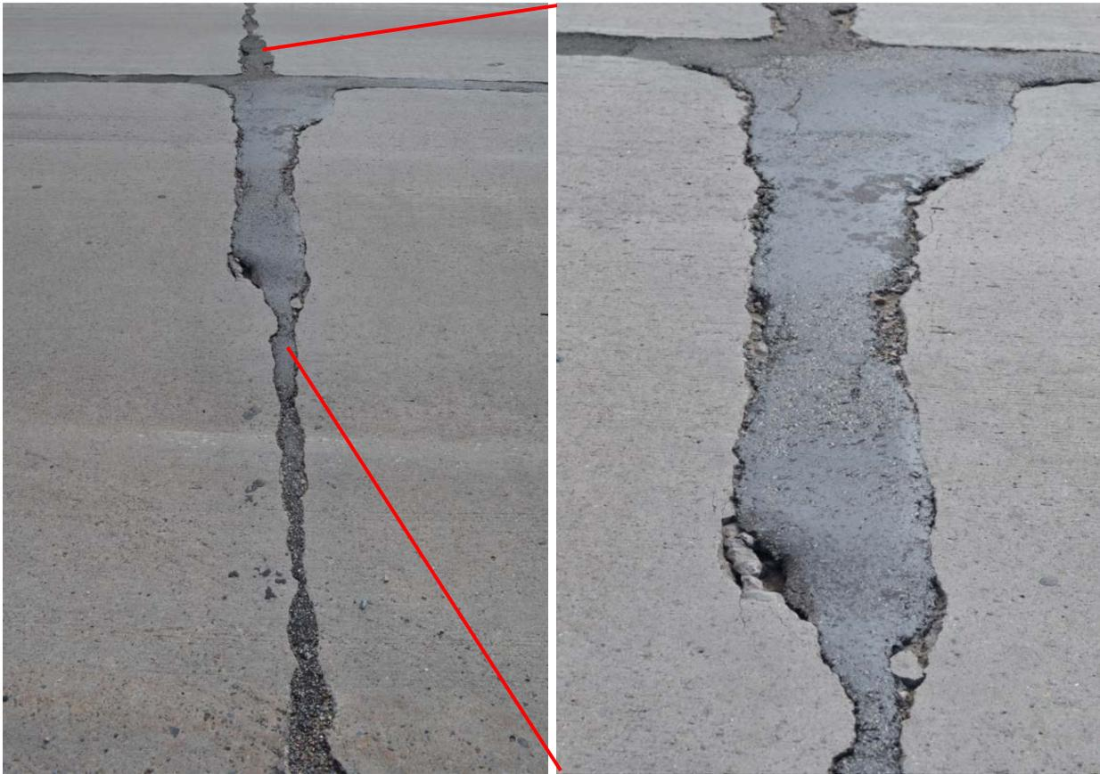
Figure F-12. PDR to address transverse joint deterioration (left) and surrounding concrete pavement deteriorating around PDR (Site #23, W. Kemp St., Rhinelander).
