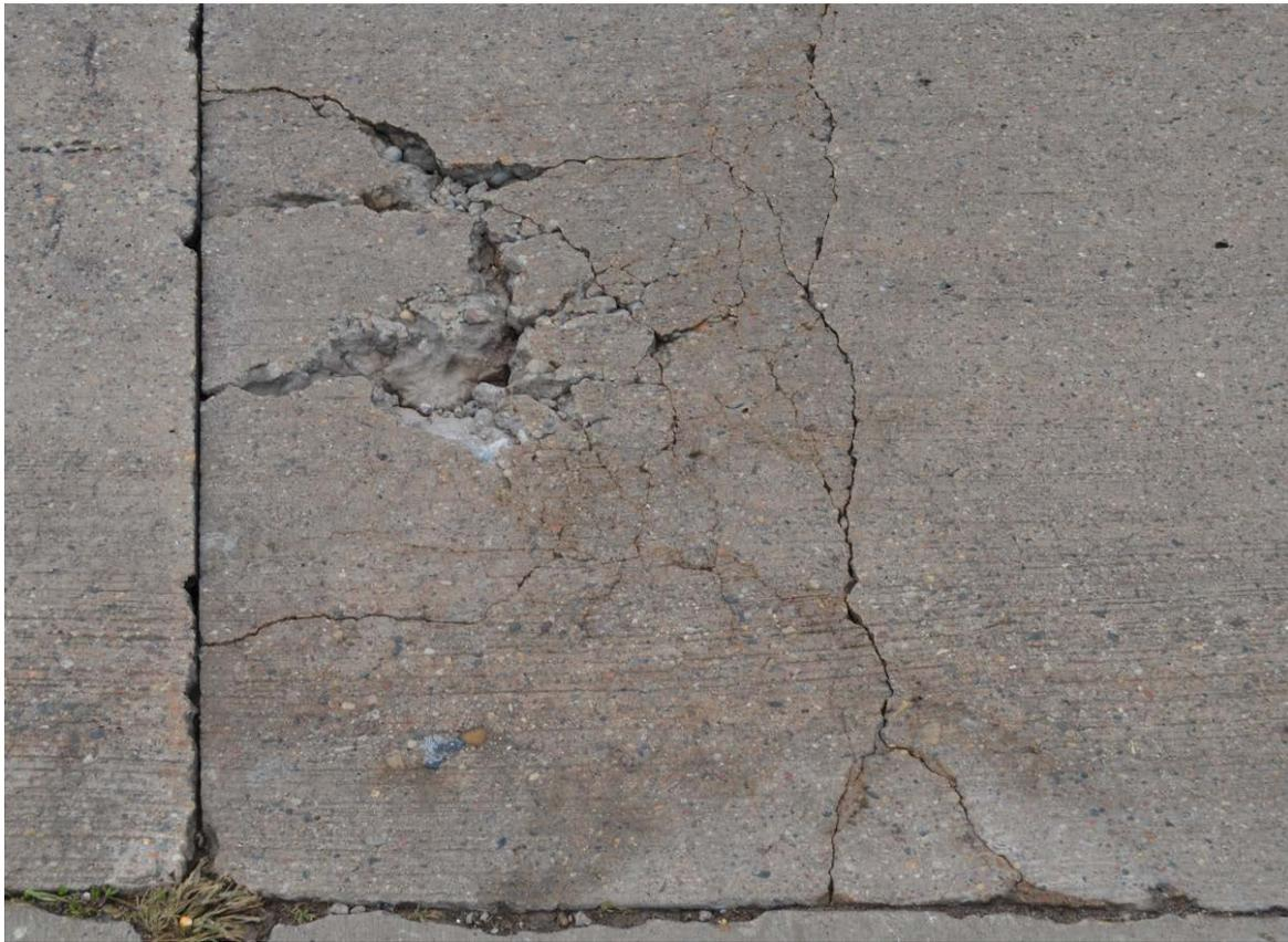
Figure E-10. Severely deteriorated areas in existing concrete pavement (Site #11, US 10, Stevens Point).
