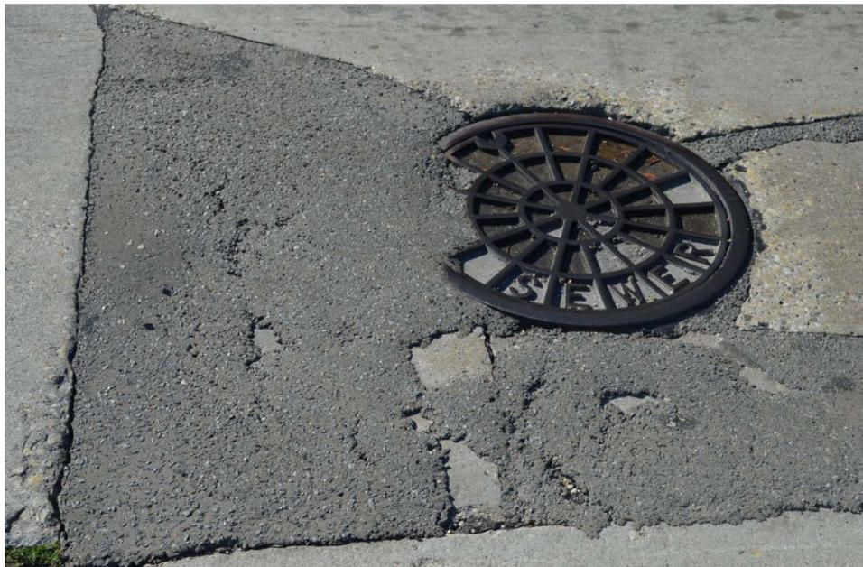
Figure E-2. PDRs to address deteriorated areas around utility hole
