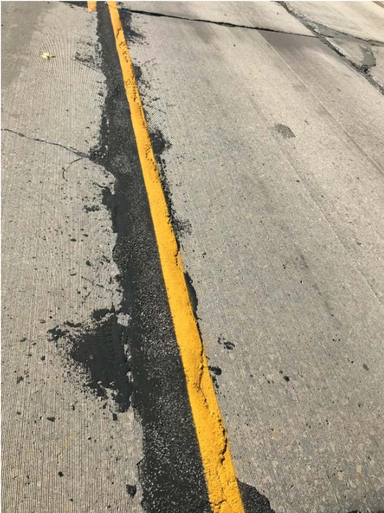
Figure F-10. PDR to address longitudinal joint deterioration
