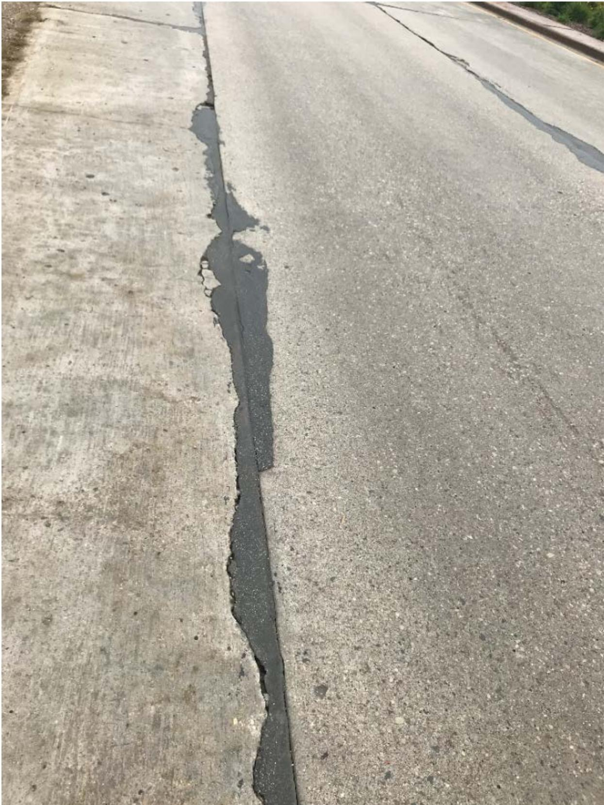
Figure D-3. PDRs to address spalling along lane-shoulder joint (Site #6, Plover Rd., Plover).
