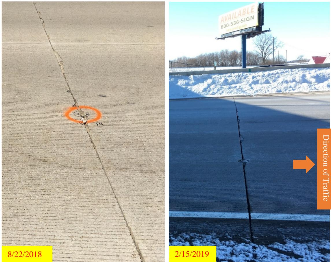
**Figure 3.10 Picture Taken from Shoulder of Core #14 Joint on I-41**
