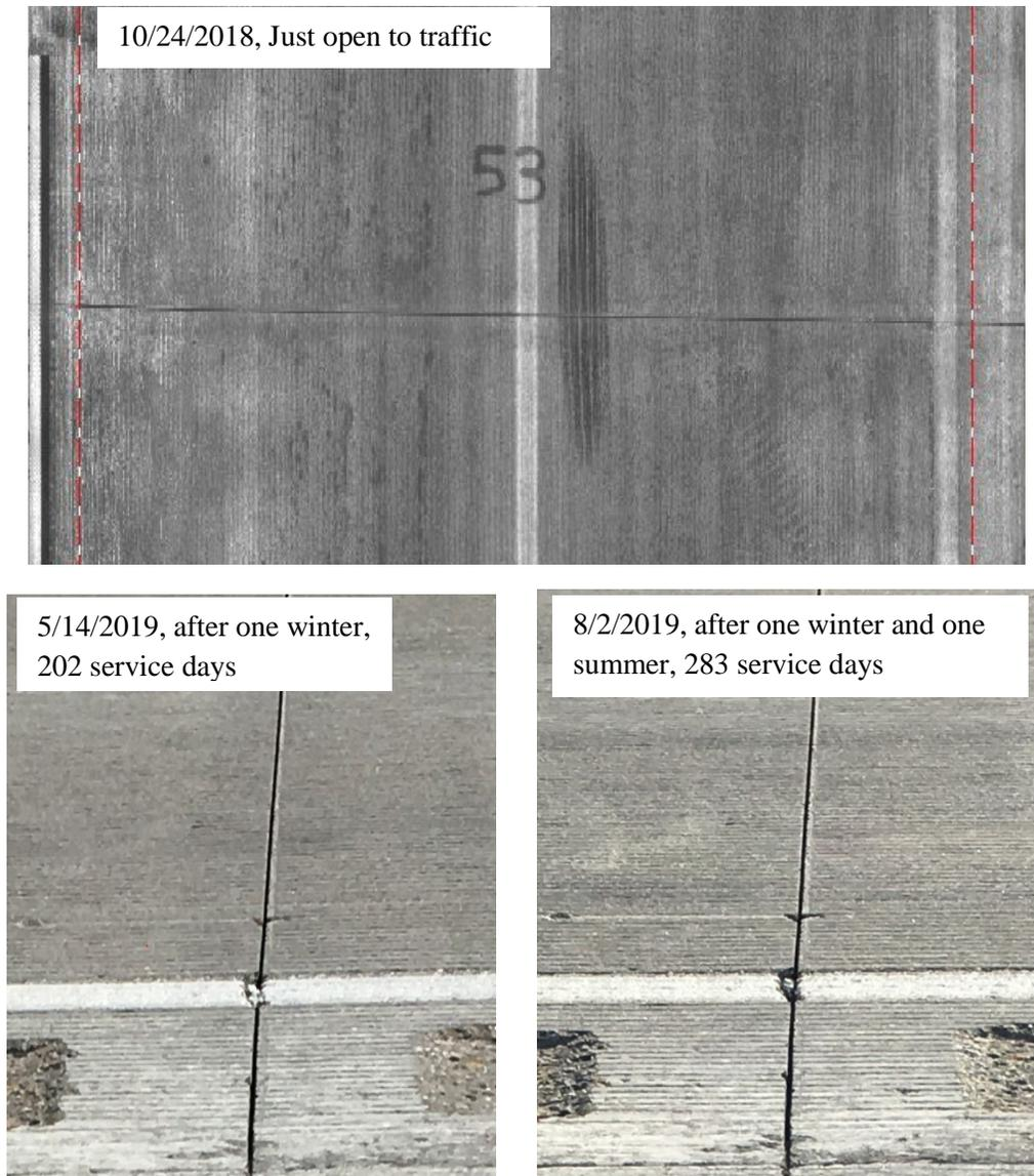
**Figure 5.3 Field Performance of Joint #53**
