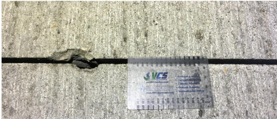
**Figure 5.5 Close-up of small spalling at Joint #104**
