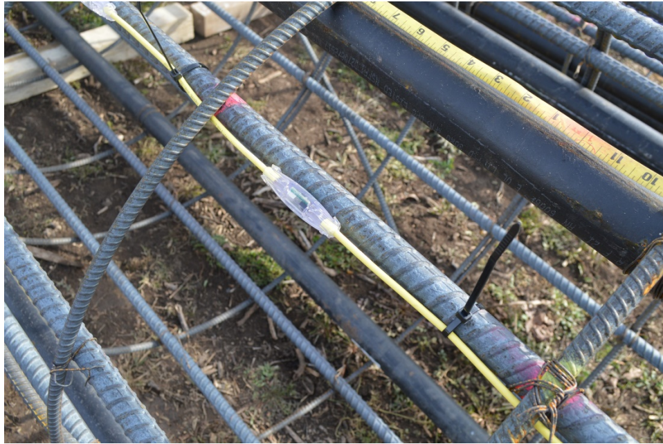
Figure 36: Close view of a TIP wire with sensor.
