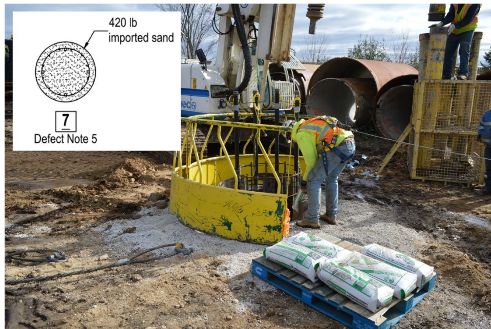
Figure 32: After placing the reinforcing cage but prior to placing concrete for Test Shaft 2, 420 lbs of sand was poured into the bottom of the excavated shaft to simulate a soft bottom for Defect 7.
