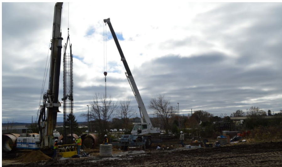
Figure 28: Reinforcing cage is lowered into the hole for Test Shaft 2. Sandbags for Defect 9 are visible near the cage mid-height.
