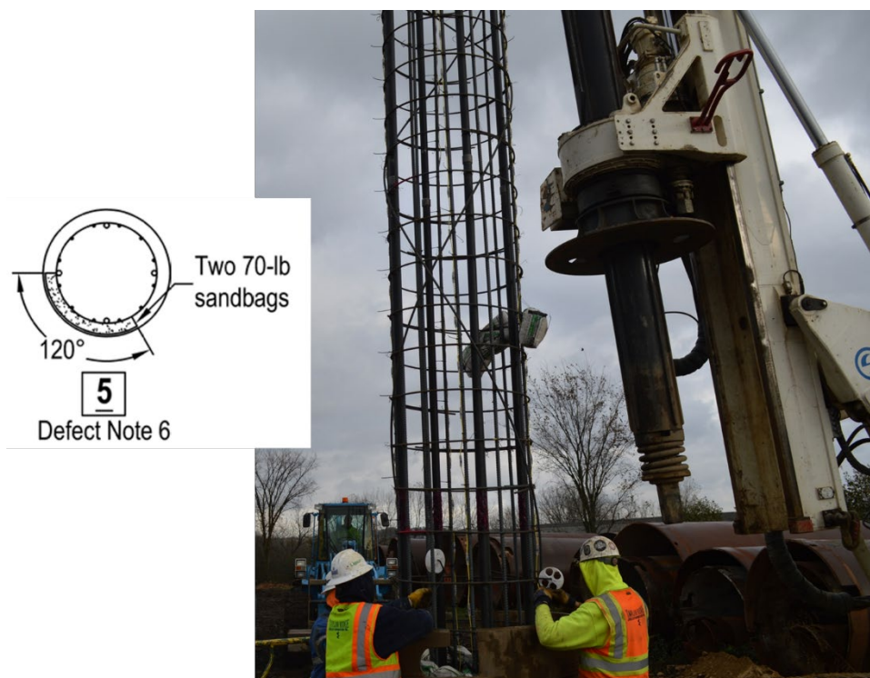
Figure 26: Defect 5 consisted of two 70 lb sandbags outside one side of the reinforcing cage for Test Shaft 1 at a depth of 12 ft.
