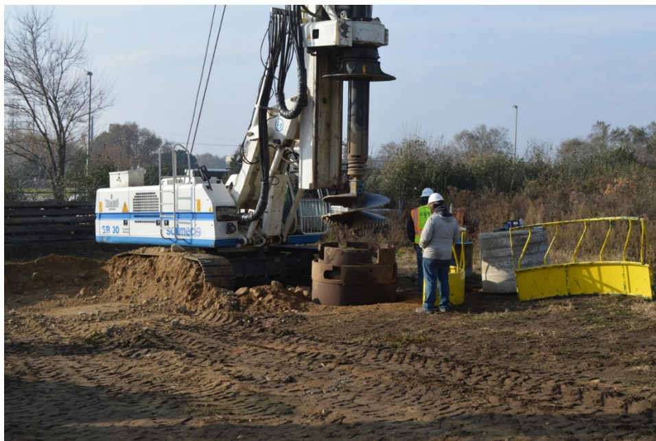
Figure 20: Excavation of shaft with 48 in. auger through telescoping casing.
