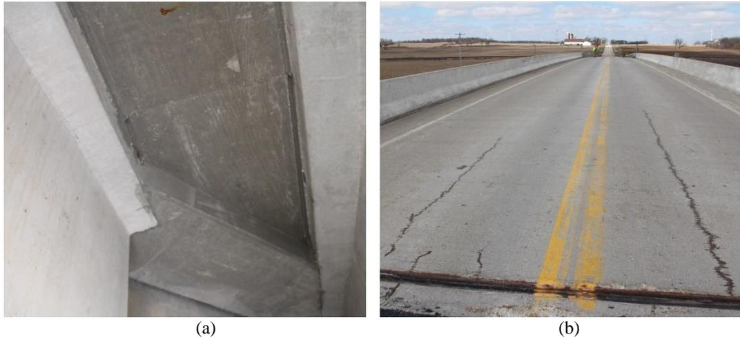
Figure 3.1. (a) Lack of cracking on deck bottom surface for 52° skew, and (b) longitudinal cracks for 0° skew near the abutment.
