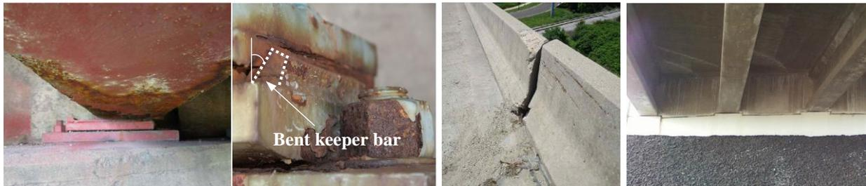
*Figure A. Misaligned girder (left), bent keeper bar (middle, left) misaligned parapet wall and closed expansion joint (middle, right), diagonal acute corner deck cracks (right). [1]*
