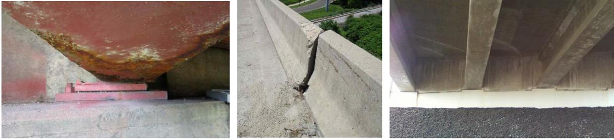
Figure 1.2. Misaligned girder (left), misaligned parapet wall and closed expansion joint (middle) of B-13-228, diagonal acute corner deck cracks (right) of B-09-212. [1]
