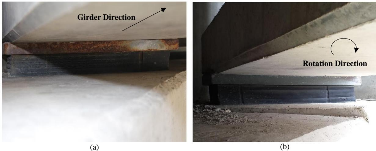
Figure 3.4. (a) Lateral displacement, and (b) rotation of the bearing for 52° skew.
