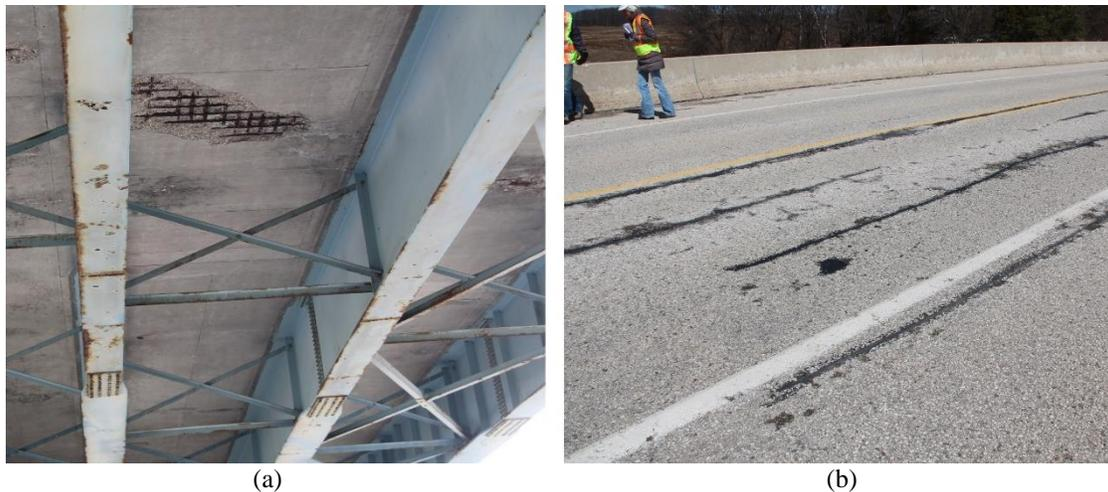
Figure 3.2. (a) Concrete spalling on deck bottom surface for 30° skew, and (b) longitudinal sealed cracks on deck top surface for 3° skew.
