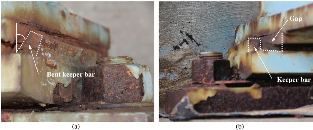
Figure 3.5. (a) Bent interior keeper bar and (b) gap between bearing and exterior keeper bar of obtuse corner bearing at north bridge end for 30° skew.
