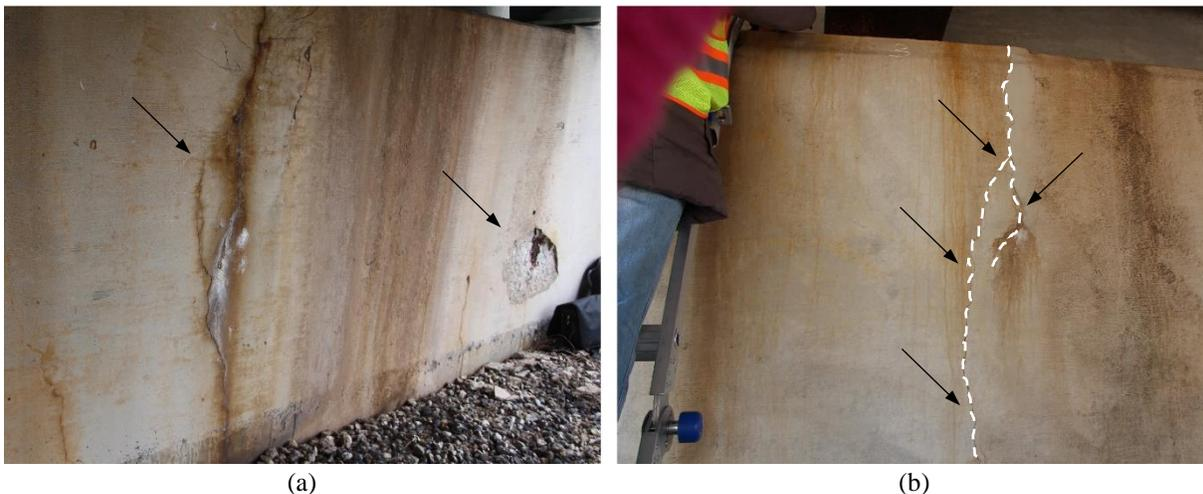
Figure 3.7. Vertical cracks on the abutments of bridges with (a) 30° skew, and (b) 3° skew.
