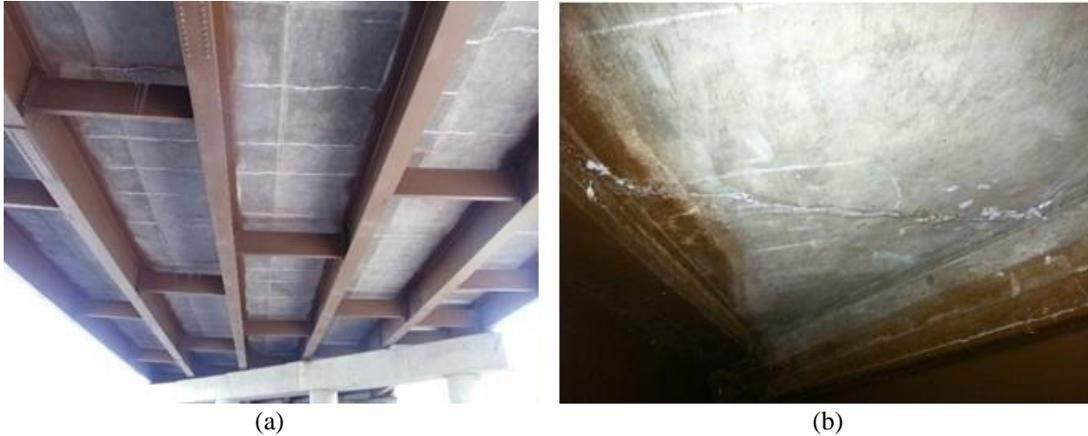
*Figure 3.9. Deck bottom face: (a) transverse cracking on west span, and (b) typical acute corner cracking at bridge ends of the load tested steel bridge.*
