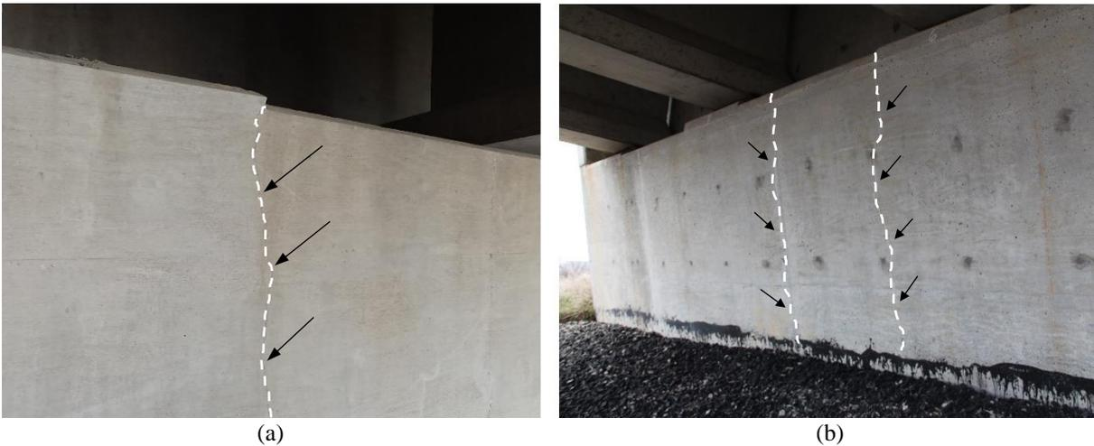
Figure 3.6. Vertical abutment cracks for bridges with (a) 52° skew, and (b) 0° skew.
