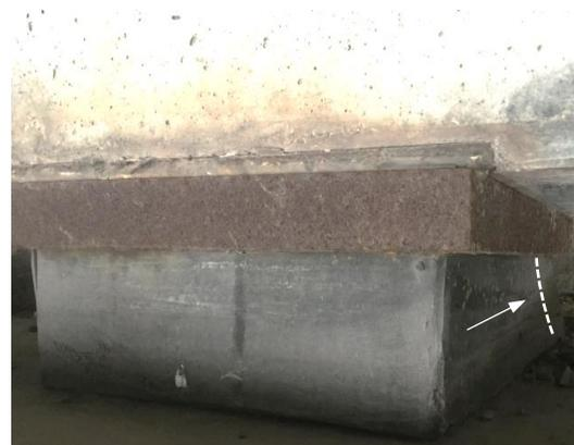
Figure 2.6. Bearing rotation at the obtuse corner. [1]
