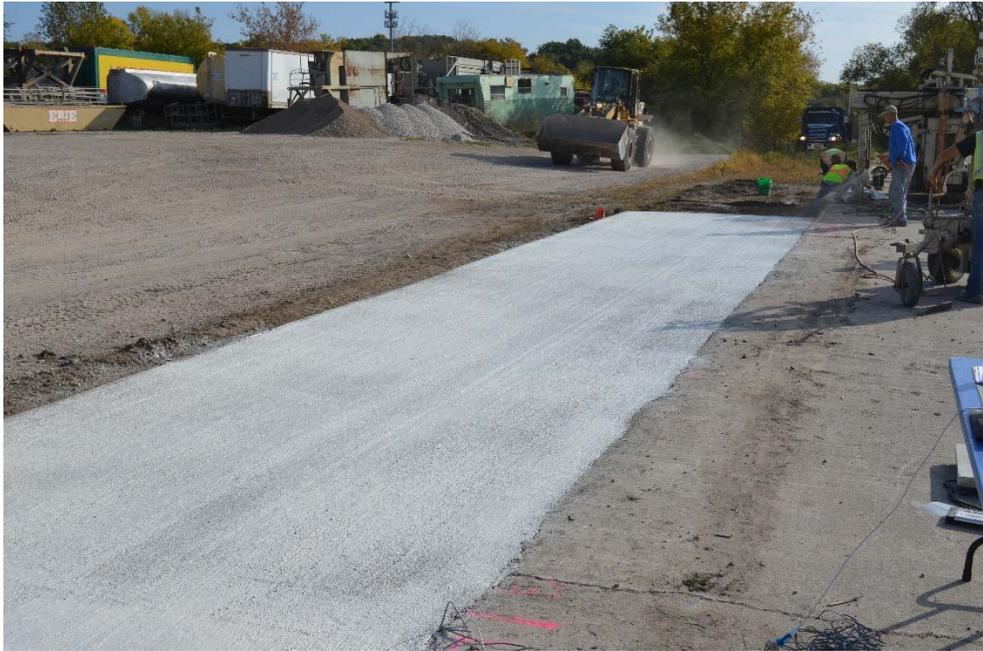
**Figure 2.5.6. Application of Curing Compound Over Gravel Mixture**
