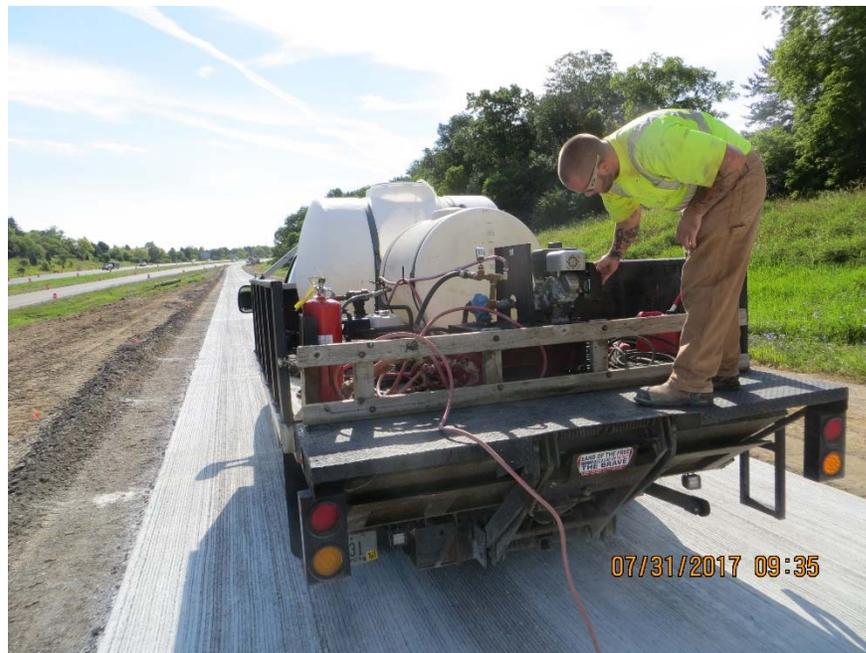
**Figure 2.10.15. Truck-Mounted Joint Sealing Equipment**
