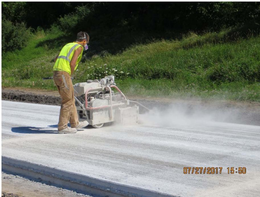
**Figure 2.10.14. Husqvarna SOFF-CUT Model 4000 Early Entry Sawing Operations**
