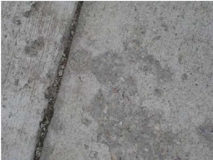
**Figure 1.8.1. Salt Scaled Concrete Surface (Zhang, 2013)**
