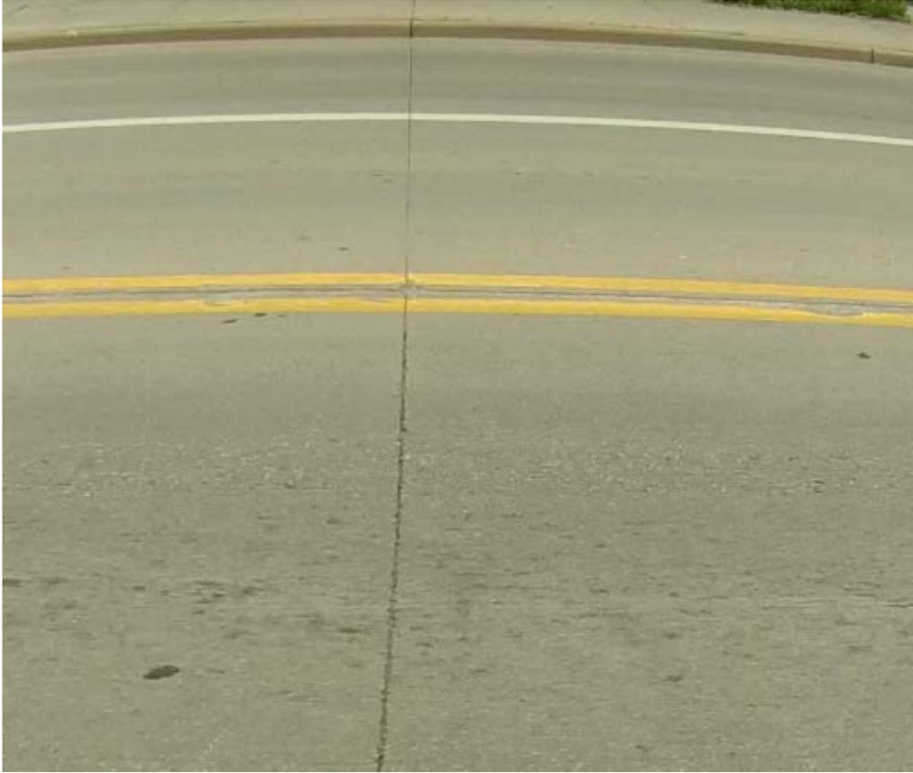
**Figure 5.3.1. Typical Joint Condition Along Birch Street, May 2015**
