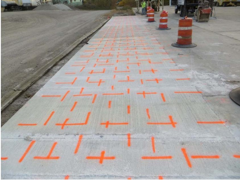
**Figure 2.6.2. Layout Markings For Full-Depth Sawing**
