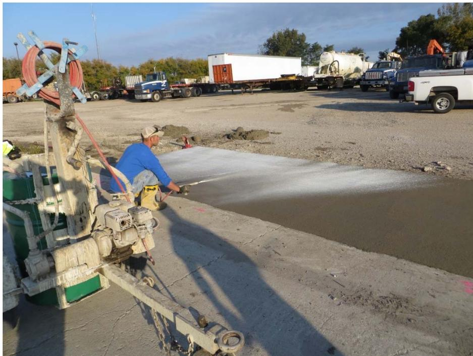
**Figure 2.5.4. Application of Curing Compound Over Limestone Mixture**
