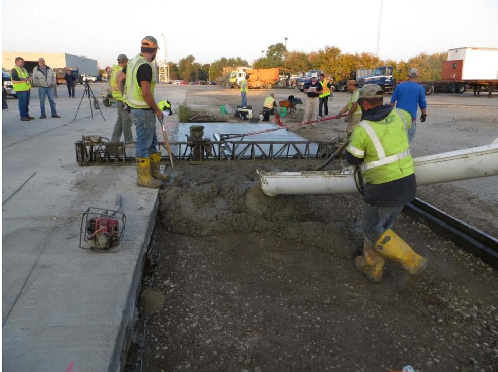
**Figure 2.5.3. Paving Operations Within Limestone Mixture**
