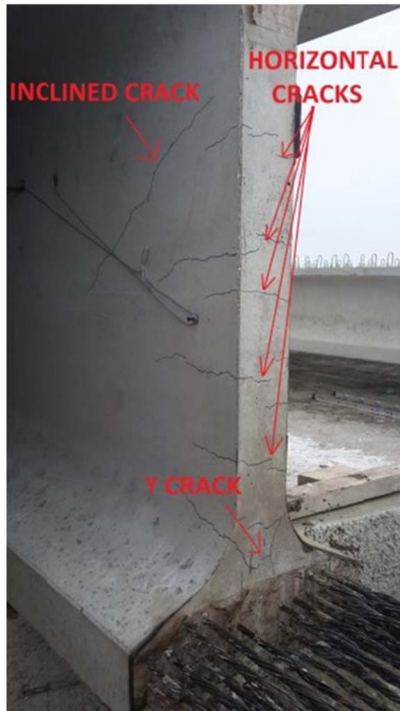
Figure 3-3. Inclined, Horizontal Web, and Y cracks shown on 72W girder.
