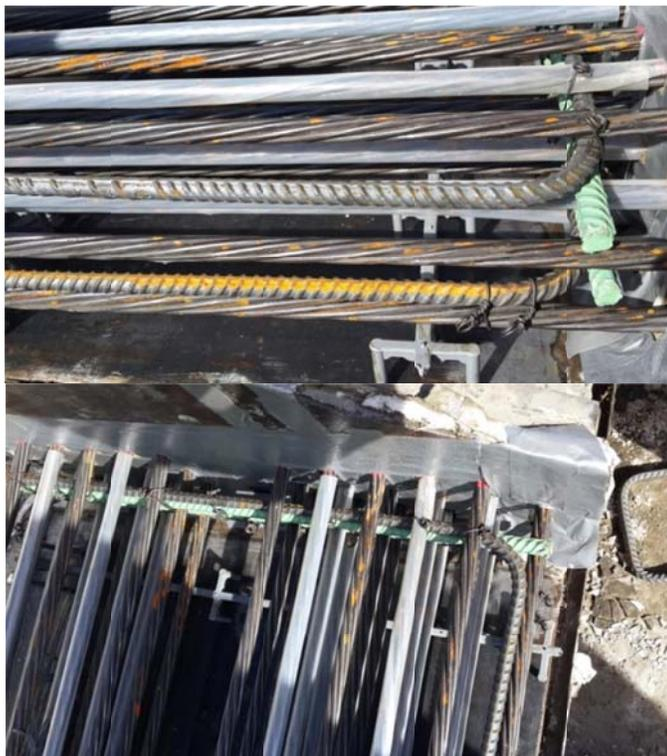
Figure 6-27. U bars beneath the top row of strands and above the bottom row of strands in side view (top) and in top view (bottom).
