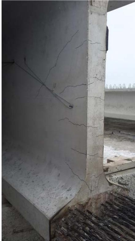
Figure 1-1. Cracks at the end of a Wisconsin 72W girder.
