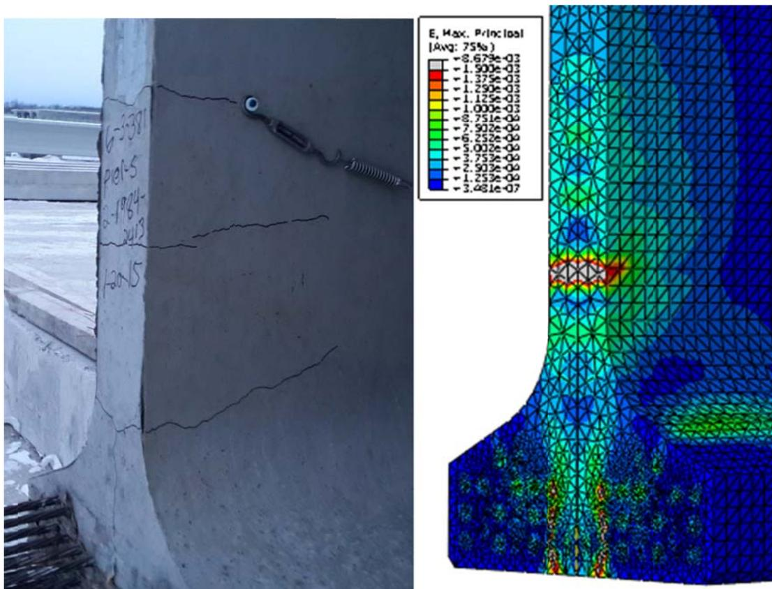
Figure 5-32. The comparison of actual girder end cracking with Abaqus model strains for the de-bonded girder.
