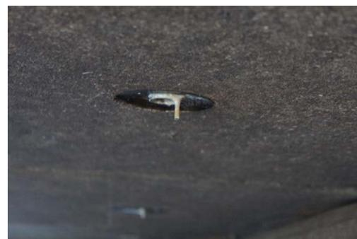
(b) Drains with moisture and efflorescence
