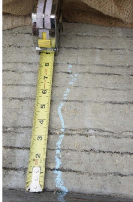
(b) Crack propagation along deck
