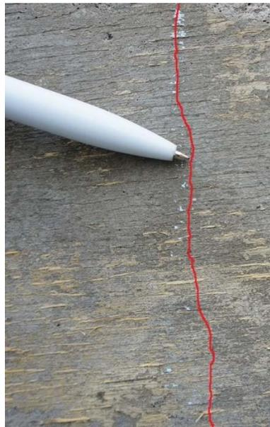
**Figure 5-7. Crack over beam 2**
