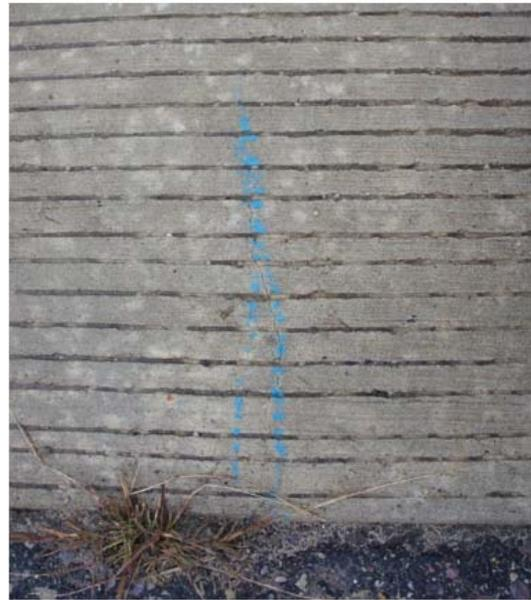
(b) A short crack over the abutment and above a shear key
