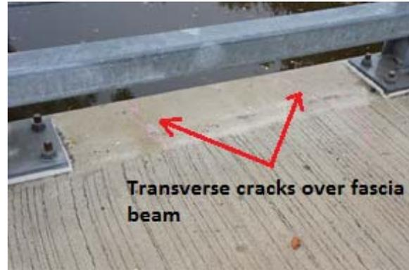
(ii) Transverse cracks over the fascia beam
