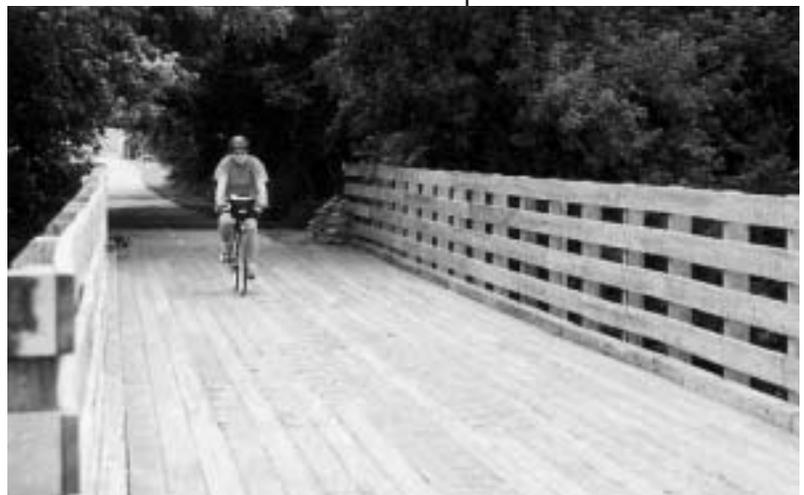
Widths less than 12 feet should apply under less demanding conditions (low pedestrian and bicycle use, a relatively flat or short bridge deck, or bicyclists are permitted to use the motor vehicle
