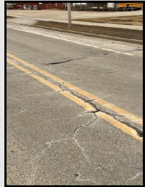
Example of pavement deterioration
