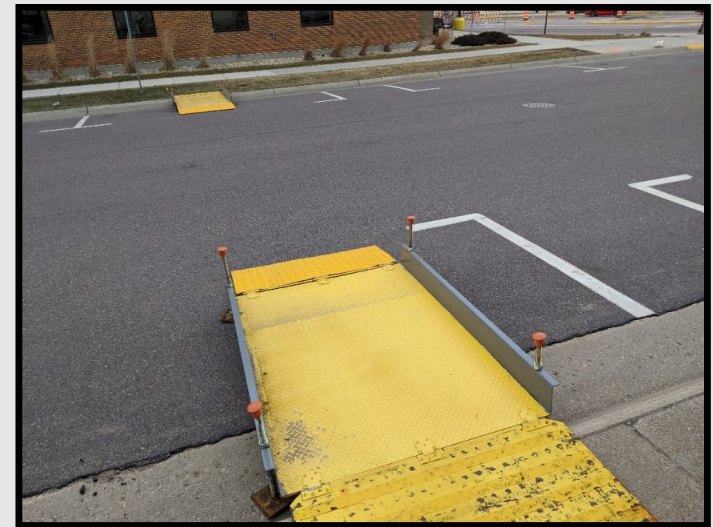
Example of temporary pedestrian curb ramp to be used during construction.
