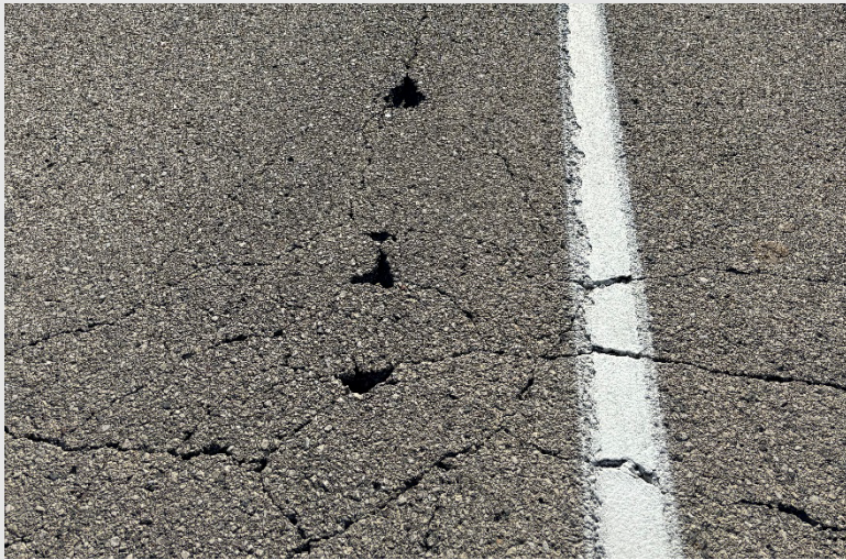
Cracking
