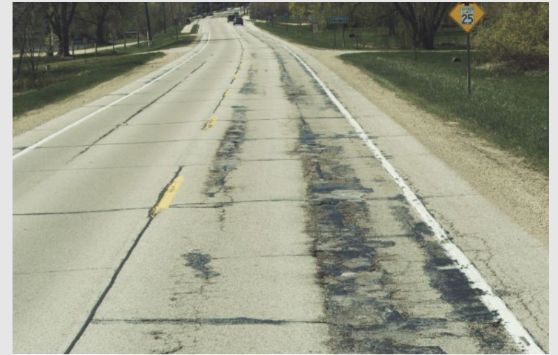
Cracking & Patching
