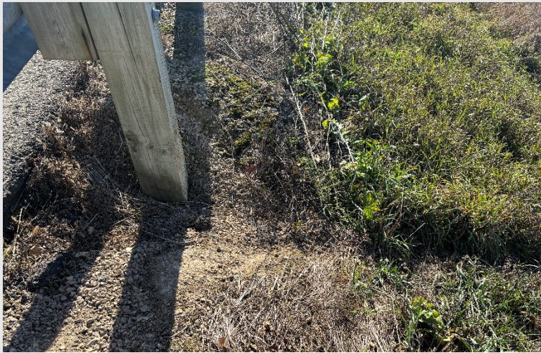
Erosion around posts
