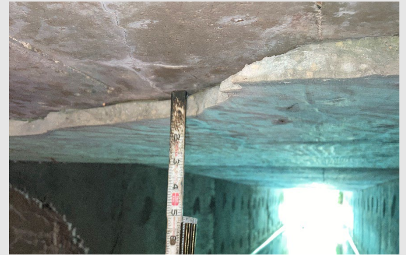
Cracking & Settling
