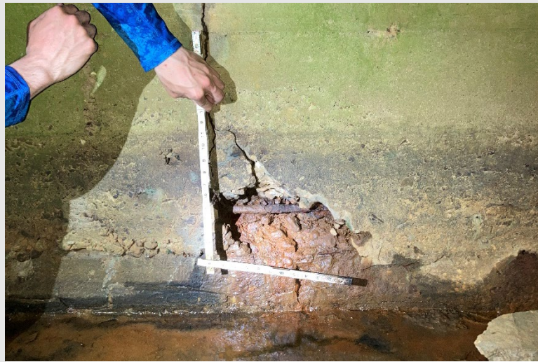
Cracking & Chipping
