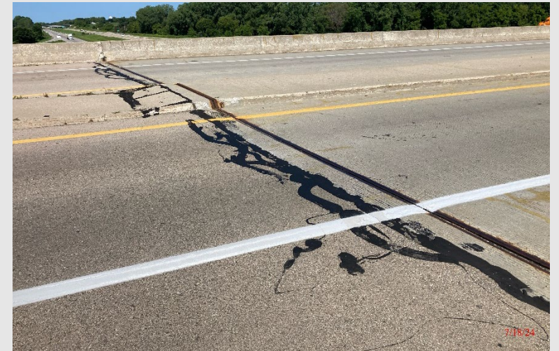
Crack Repairs
