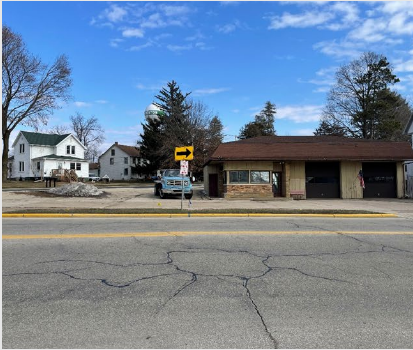
Pavement deterioration
