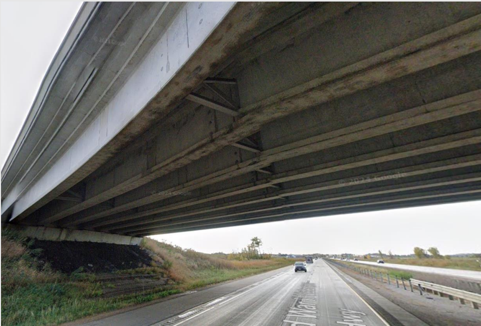
WIS 49 over I-41(B-14-0115) – spalling between girders and deteriorating bridge deck
