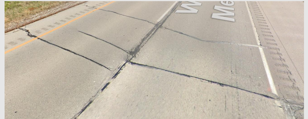
Deteriorating pavement; cracking and rutting, guardrail deficiencies, deteriorating guardrail
