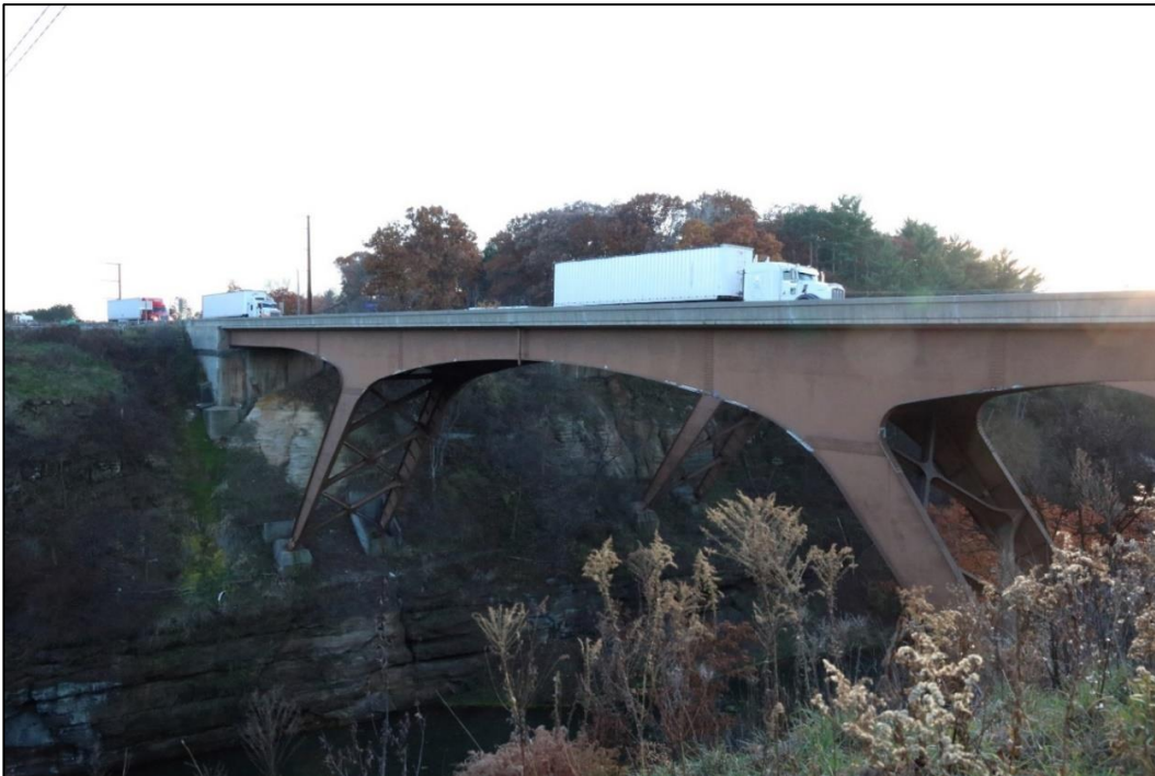
Figure 3-36: View of I-90/94 Bridge over Mirror Lake
