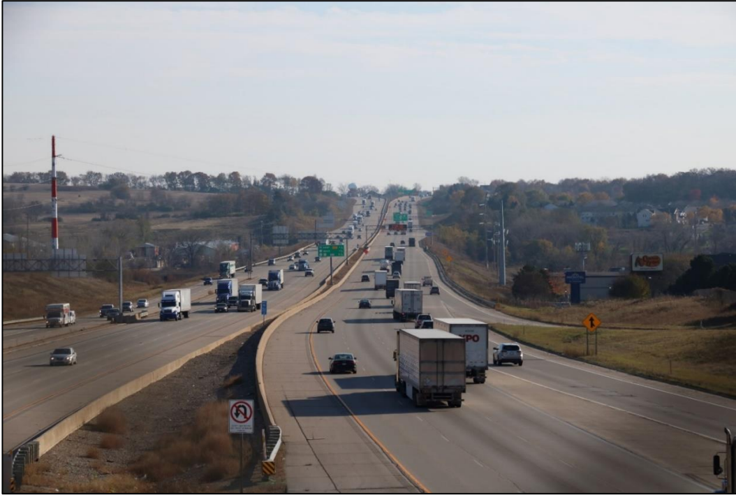
Figure 3-29: View of I-39/90/94 from High Crossing Boulevard
