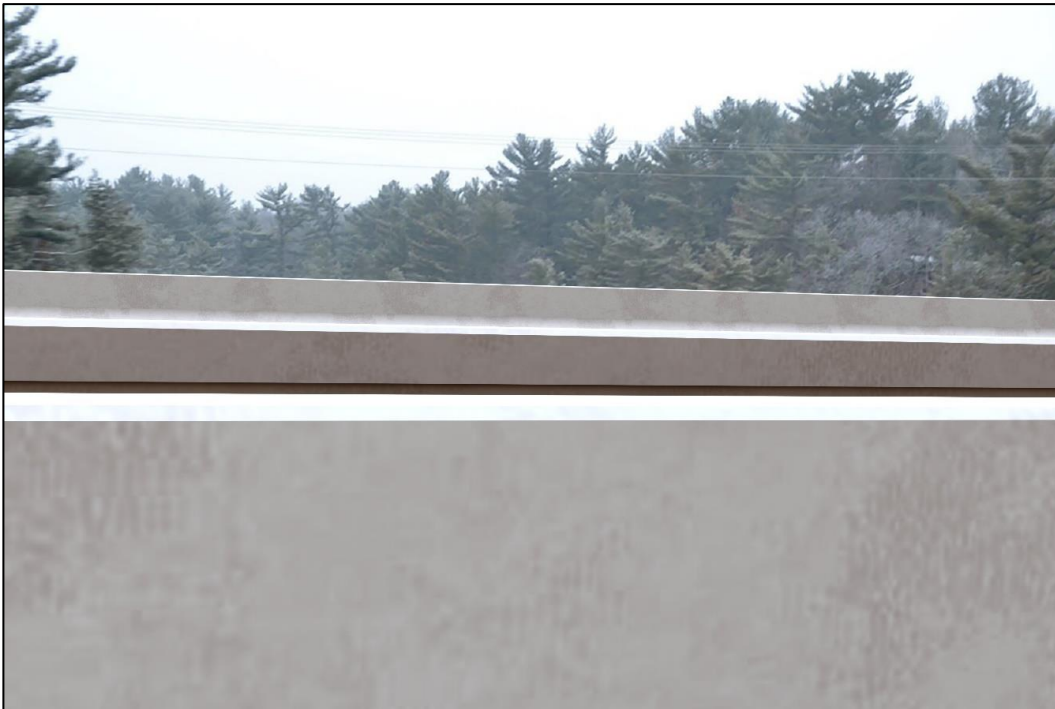
Figure 3-42: View for Northbound Travelers Looking West, Bridge Replaced
