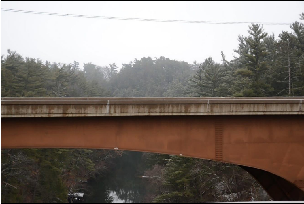
Figure 3-43: View for Southbound Travelers Looking East, Existing Conditions
