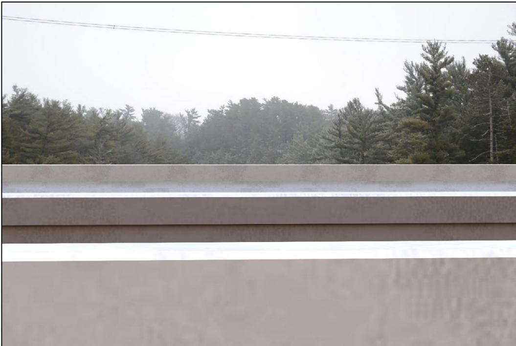
Figure 3-44: View for Southbound Travelers Looking East, Bridge Replaced
