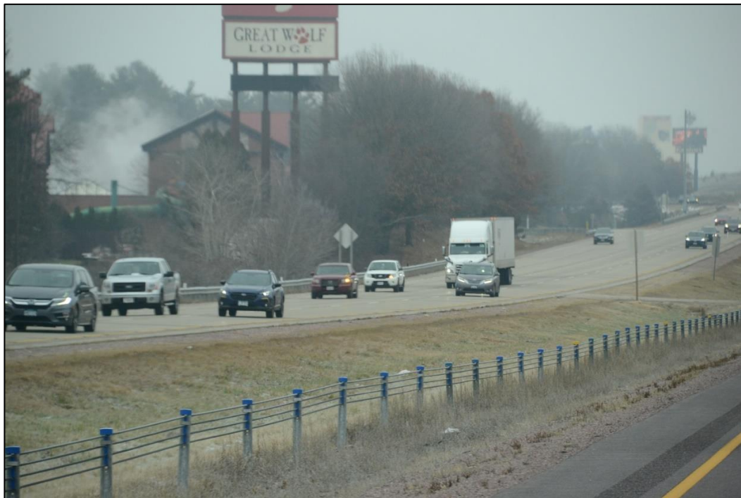
Figure 3-34: View of I-90/94 in the Wisconsin Dells
