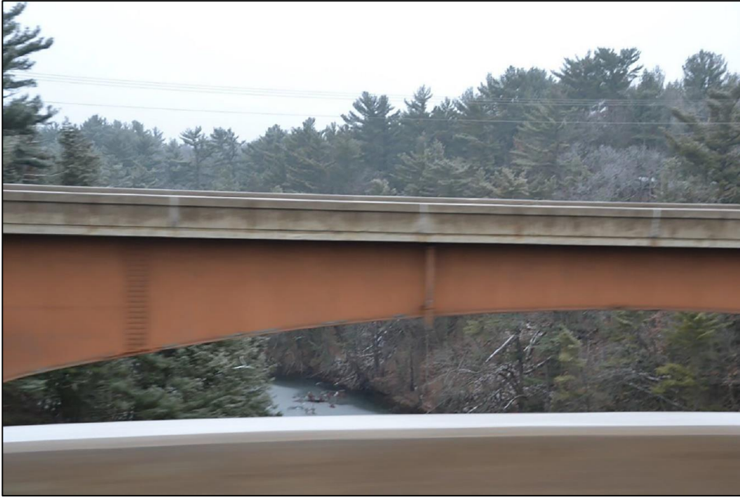
Figure 3-41: View for Northbound Travelers Looking West, Existing Conditions
