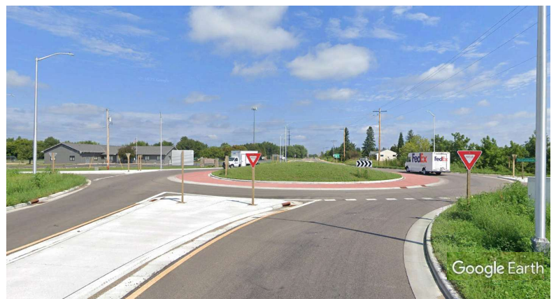
Single-lane Roundabout Example
