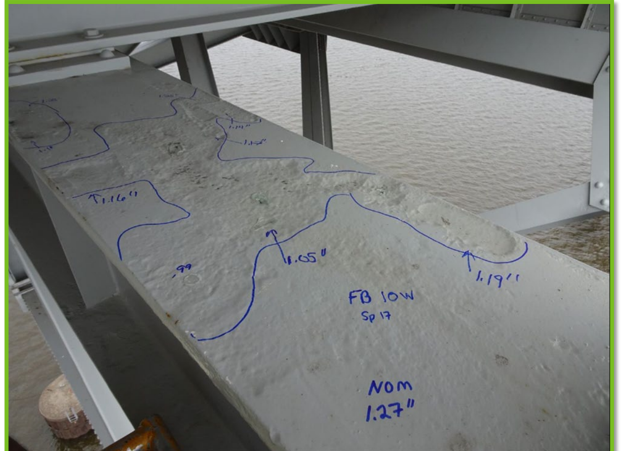
ST035 9030_2020 Span 17 Floorbeam 10 West Side Top FFlange Losses
