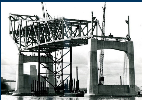
1960: The steel framework of the High Bridge rises above the St. Louis Bay.
