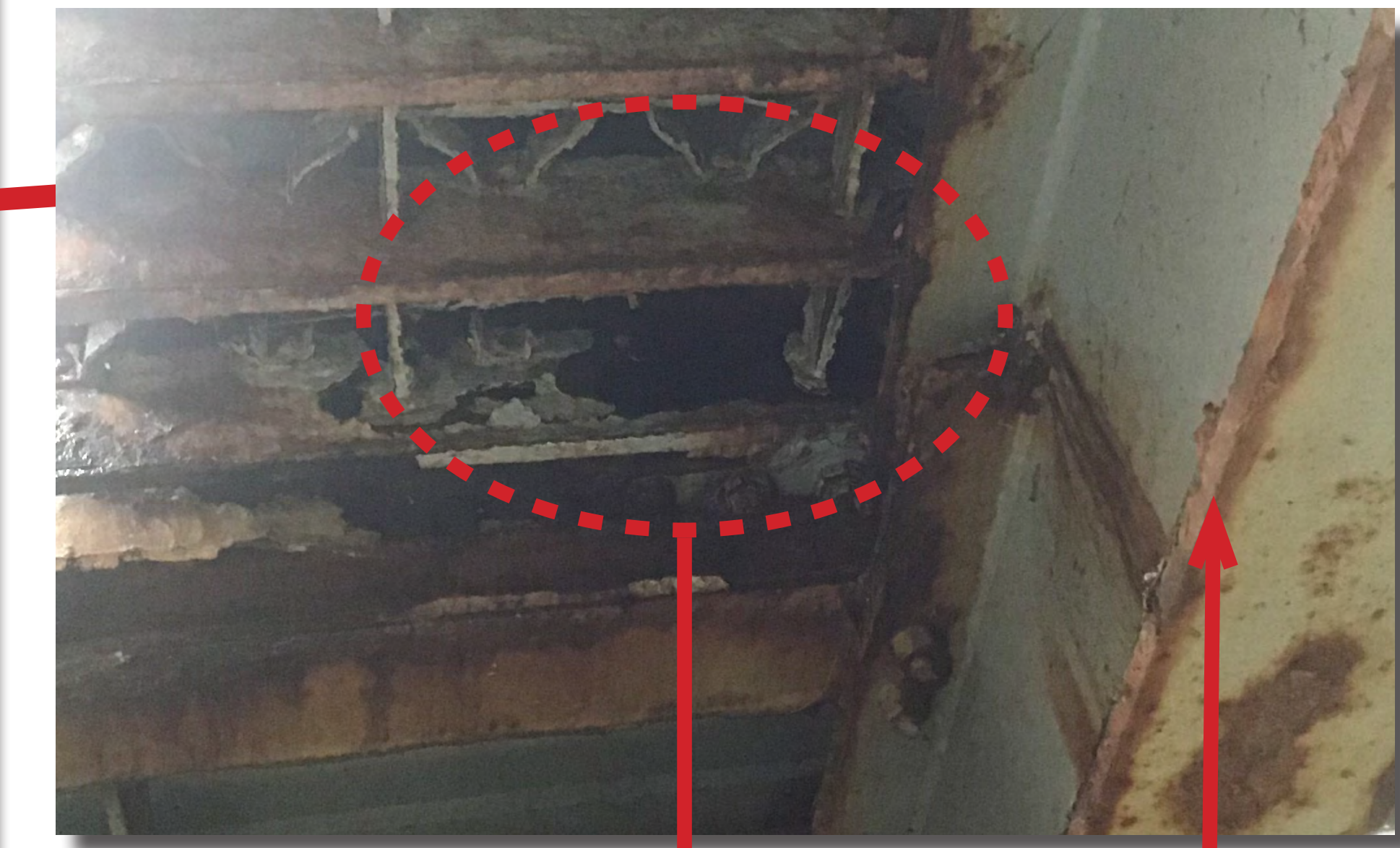
Replace Median Barrier and Stringers
