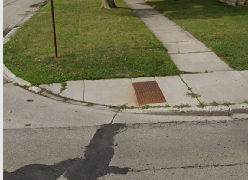
Multi-modal Accommodations/Curb Ramps
