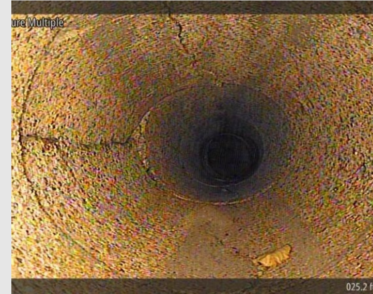
Storm Sewer Condition
