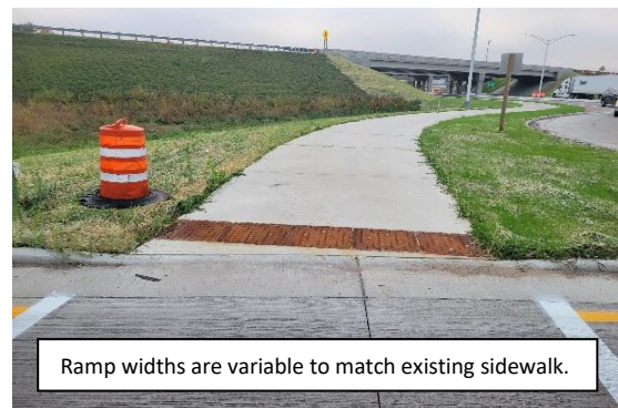
Compliant curb ramp
