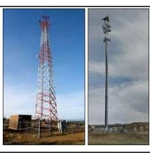
Macro cells may be installed on rooftops, building facades, monopoles and other steel structures. These cells provide coverage over a broad area (up to several miles). When on monopoles, they are typically over 50 feet in height.
