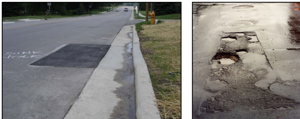
Figure 5: Both patches improperly backfilled/compacted, and not patched to nearest joint or seam
