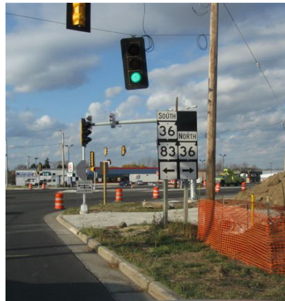
Figure 6: Temporary driveway within the functional area of an intersection
