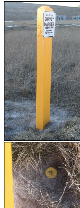
Figure 4. ROW monument with yellow cap and yellow plastic post with sign nearby. Posts may be metal too.
