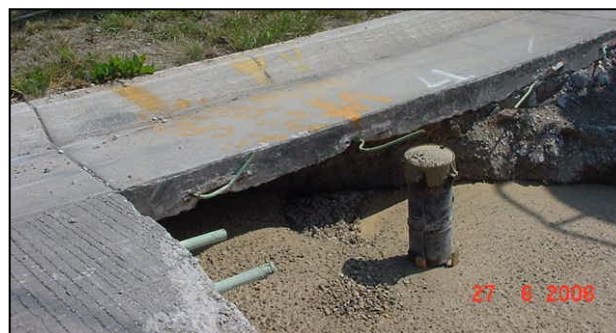
Figure 2: Concrete pavement repair without sawcut. Note top of pavement edge and missing dowel bar. In lower picture, dowel bars in gutter are bent and not ready to accept slurry.
