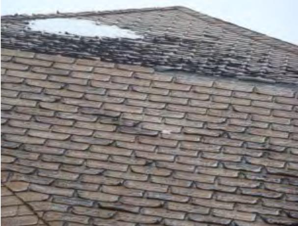
Weathered shingles-curling/missing (Poor - 40 total points)
