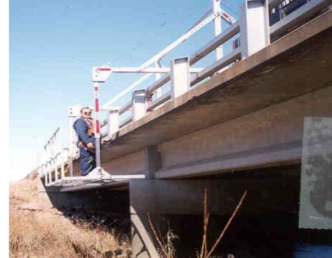
Class 9118 Scaffolding w/ electric hoist
