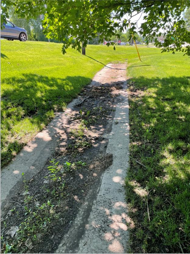
Concrete Channel Containing Sediment
