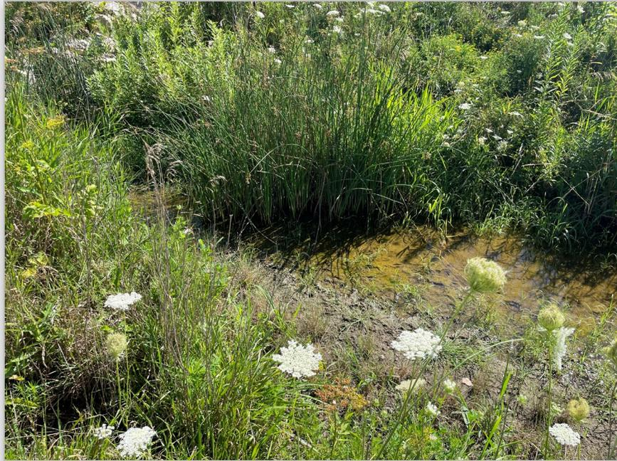
Pooling Water in Bioretention Basin
