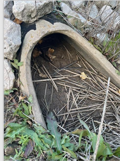
Sediment in Drainage Pipe
