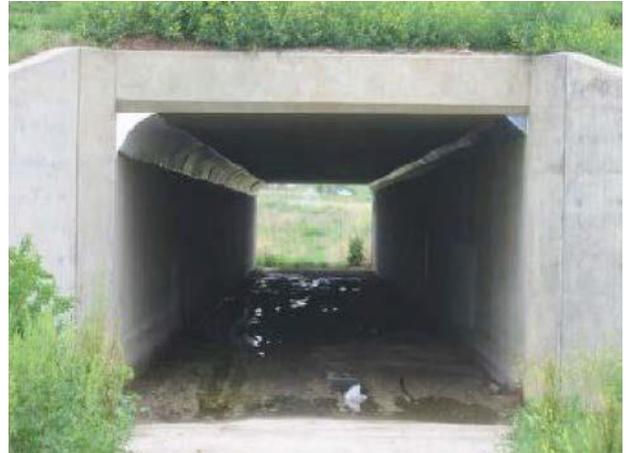
Properly installed corner slopes on a box culvert (GDOT)
