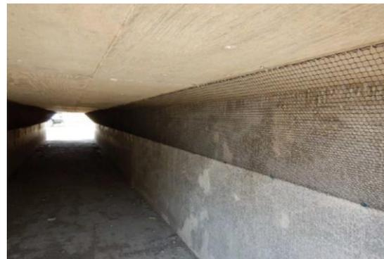
Properly installed culvert corner netting (TxDOT)
