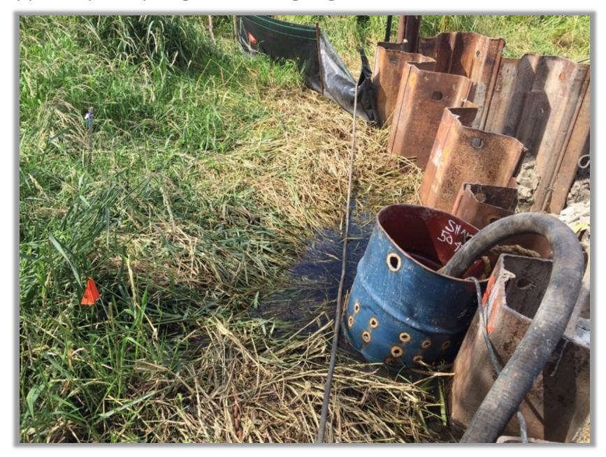
Good example: Managing pump intake water to prevent sediment being introduced to operation
