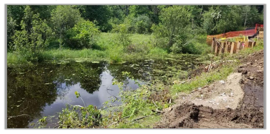
Issue: the downstream water has visible plume of discolored water when comparing to upstream water quality – therefore issue with dewatering operation that needs attention.
