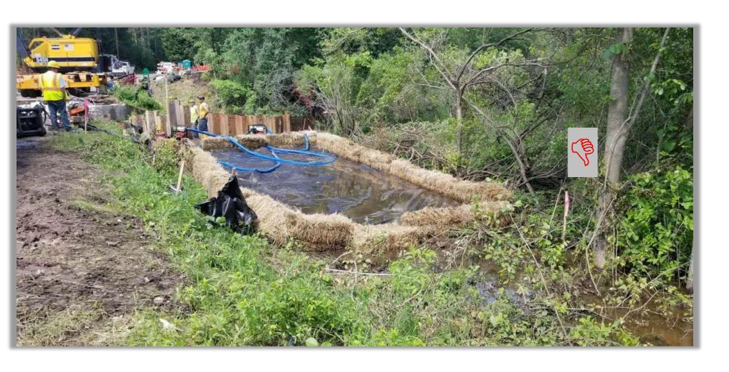
Issue: End of pump hose not connected to filter bag (lower right corner of picture)
