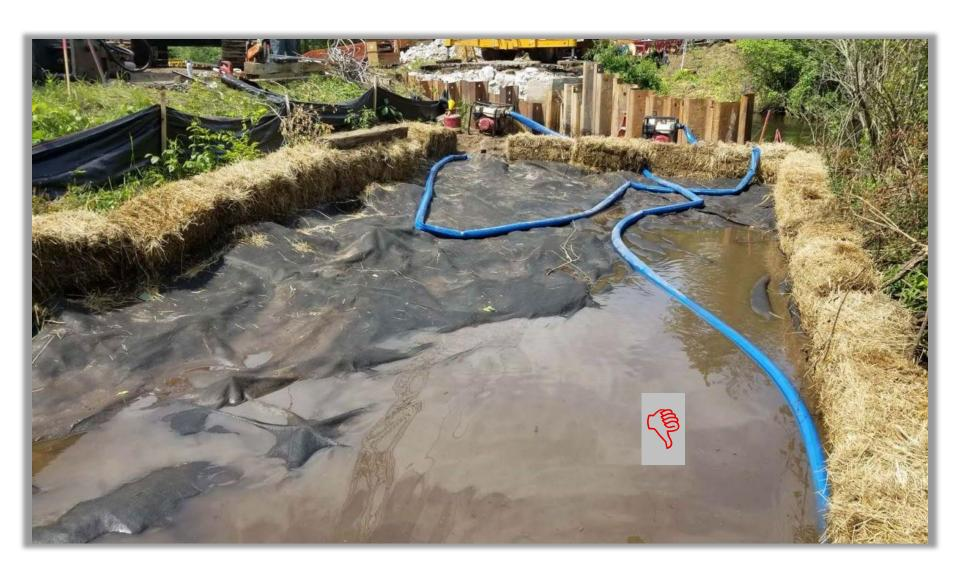
Issue: Large amount of sediment present in water because not filtered by bag
