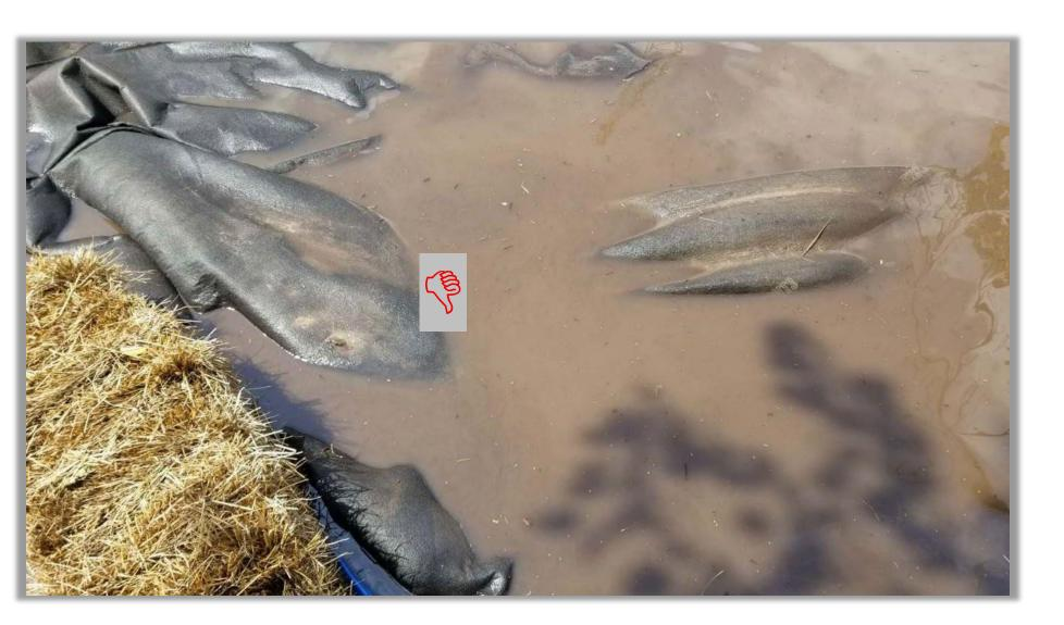
To determine if dewatering operation is adding turbidity, look upstream of operation. In this example, the upstream water showed no turbidity.
