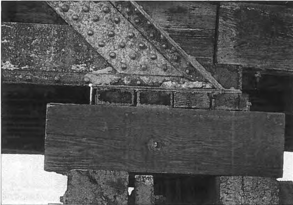
Chicago and Northwestern Bridge No. 2476 (P-14-125), Town of Lebanon, Dodge County Bearing block, northwest end - Source: J.A. Hess, 1986
