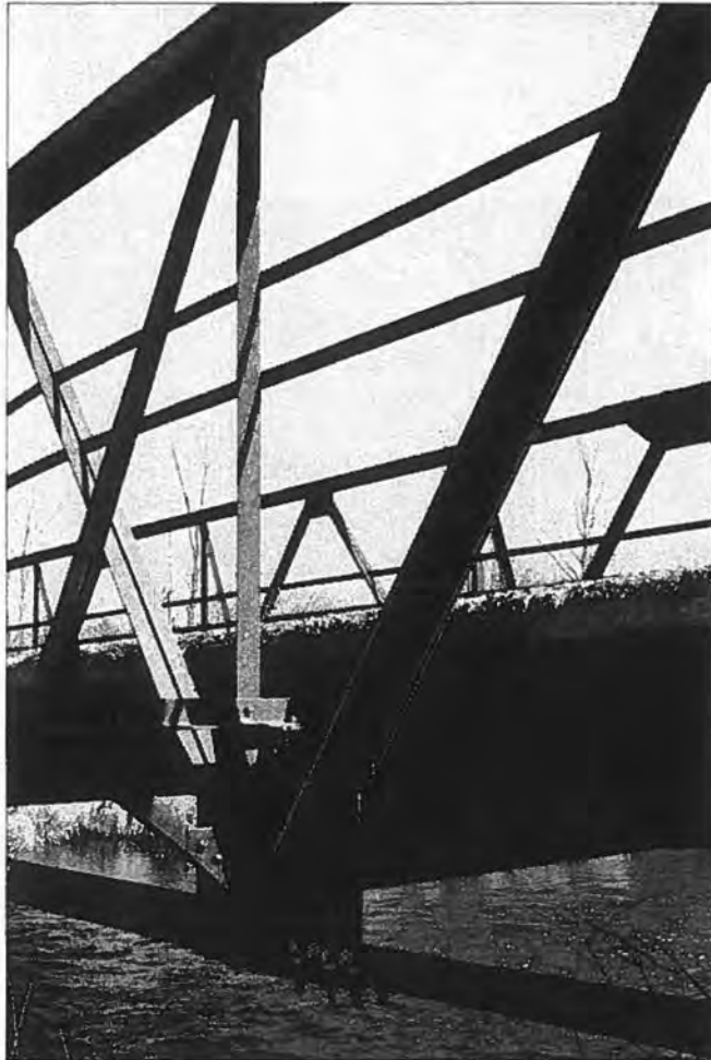
River Road Bridge (P-34-067), Town of Ackley, Langlade County Detail of post and hanger - Source: J.A. Hess, 1986
