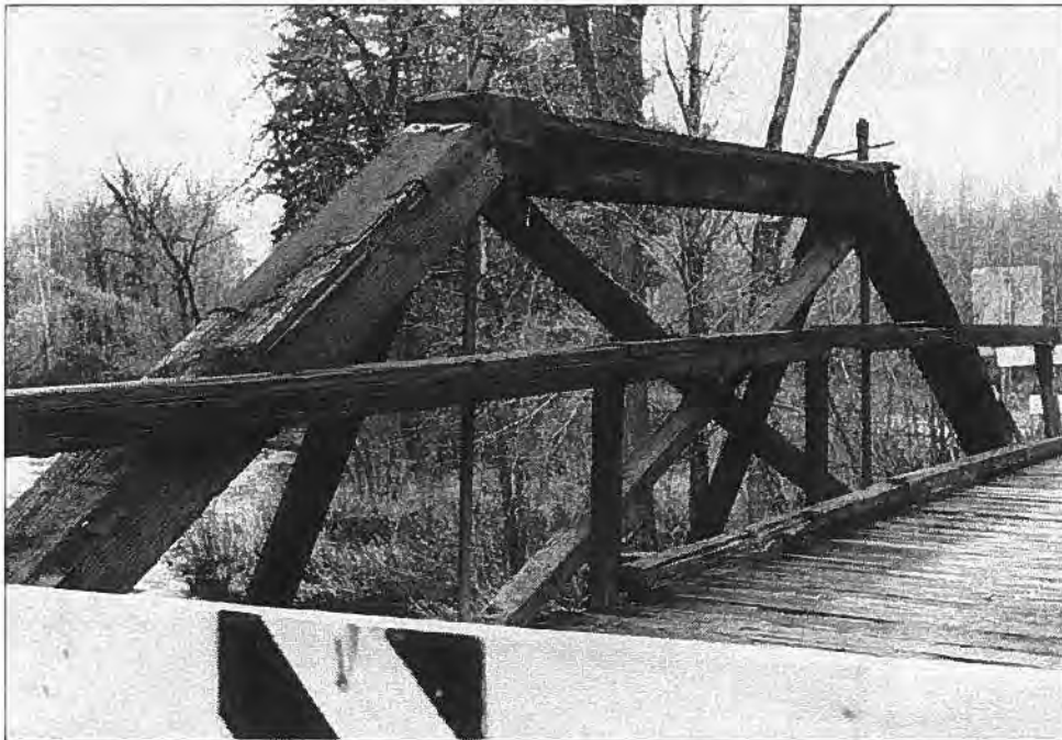
Taylor Bridge (P-16-097), Town of Amnicon, Douglas County Detail of timber truss members - Source: Wisconsin Department of Transportation
