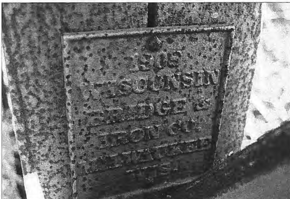
River Road Bridge (P-34-067), Town of Ackley, Langlade County South approach, detail of builder's plate - Source: J.A. Hess, 1986
