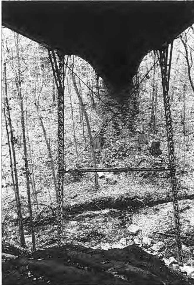
Bridge Of Pines (P-09-718), Town of Tilden, Chippewa County Looking underneath deck at center-span support columns with sway bracing - Source: J.A. Hess, 1986
