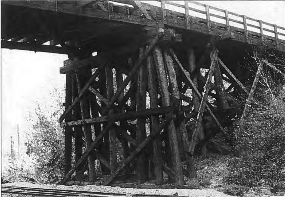
Old Wells Road Bridge (P-18-720), City of Eau Claire, Eau Claire County Top: West elevation - Source: J.A. Hess, 1986 Bottom: Trestle work, south approach span - Source: J.A. Hess, 1986
