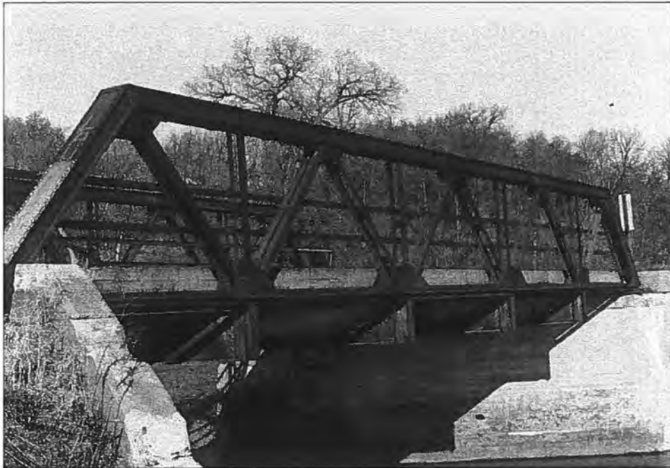
Coltman Bridge (P-33-217), Towns of New Diggings and Benton, Lafayette County Detail of side elevation and abutments- Source: Wisconsin Department of Transportation
