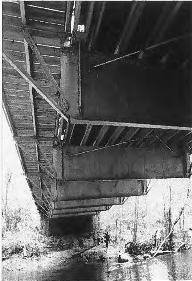
Irvine Park Main Bridge (P-09-709), City of Chippewa Falls, Chippewa County Detail of deck girders and cantilevering for sidewalk, west elevation - Source: J.A. Hess, 1986
