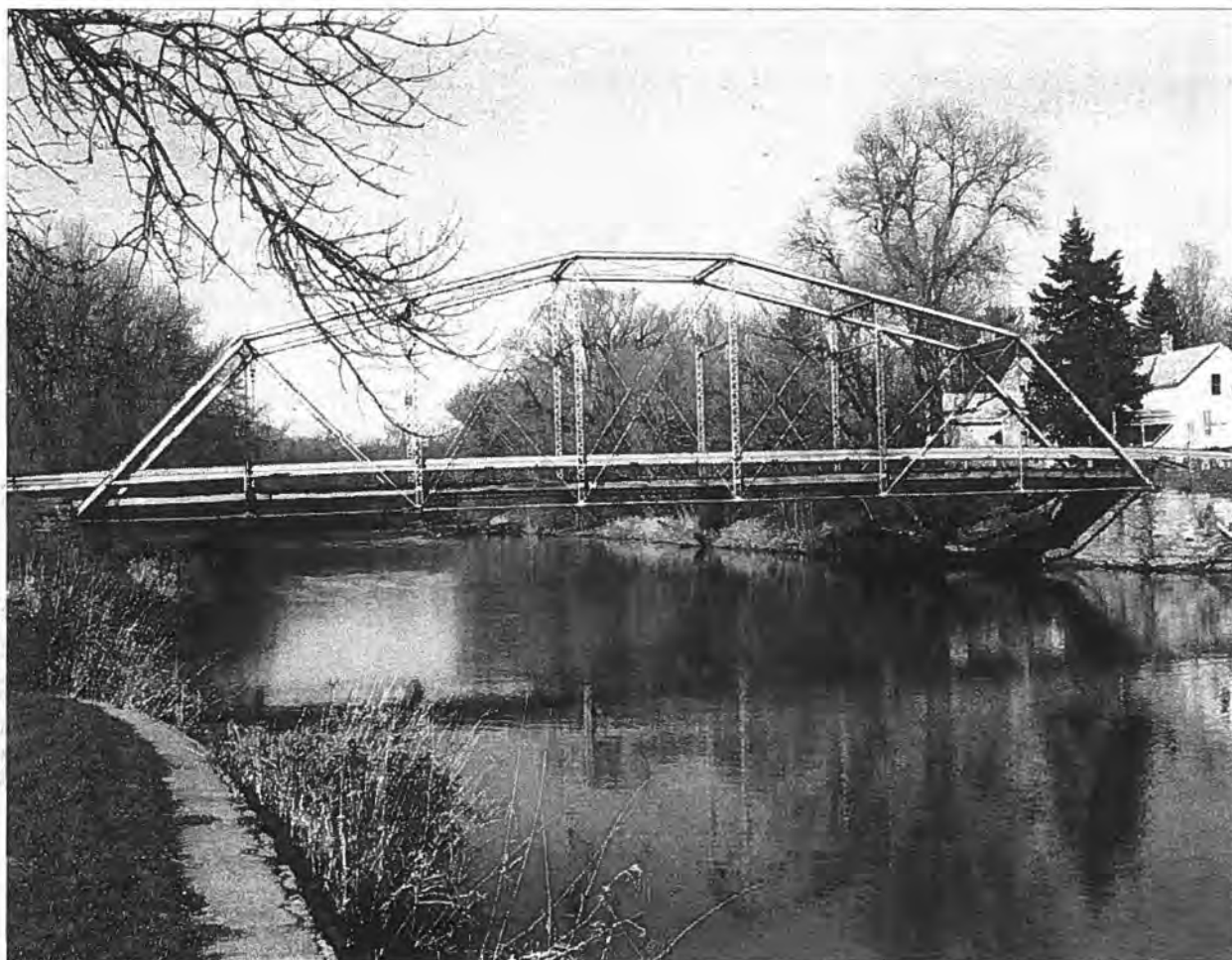
Figure 22: Manchester Street Bridge (P-56-713), Baraboo, Sauk County. Erected by the Milwaukee Bridge and Iron Works in 1884, this camelback truss was moved to a city park in 1987. (Source: Robert M. Frame III, Field Inventory Photograph, 1986).
