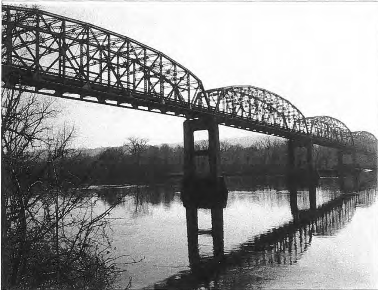
Figure 31: Bridgeport Bridge (B-12/22-850), Town of Wyalusing, Grant County; seven-span Pennsylvania truss, erected 1931. (Source: Robert M. Frame III, Field Inventory Photograph, 1986).
