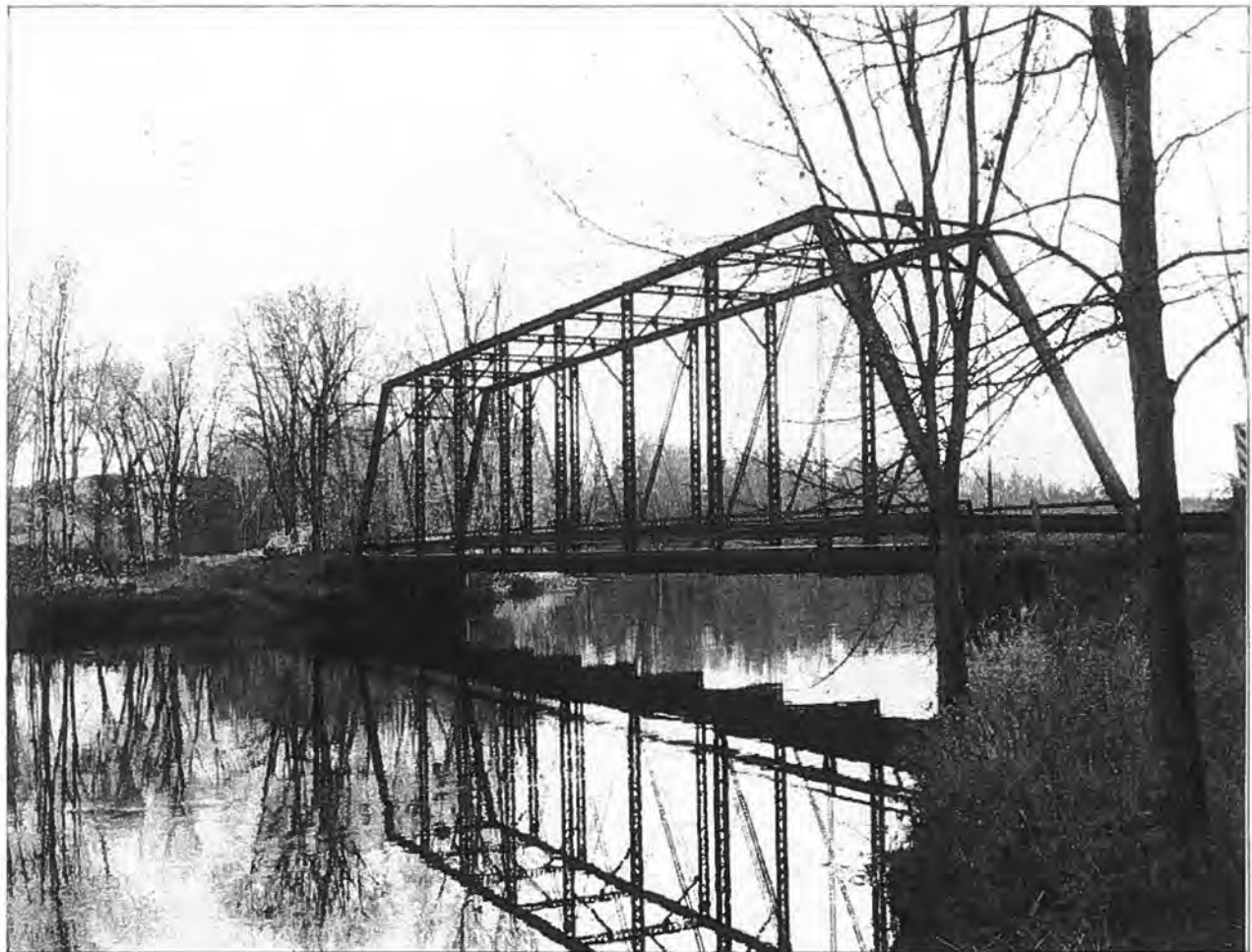
Figure 30: Ferndale Road Bridge (P-38-096), Towns of Lake and Grover, Marinette County; overhead Pratt truss, erected 1910 by Elkhart Bridge and Iron Company. (Source: Robert M. Frame III, Field inventory photograph, 1986).
