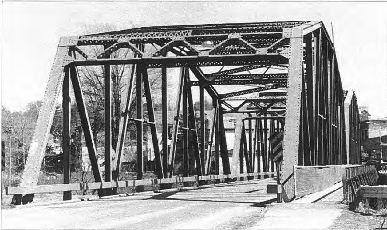
Figure 67: The STH 78/81 (Argyle) Bridge (P-33-088) displays the clean look of the SHC's Warren overhead standard plan. (Source: WisDOT).
