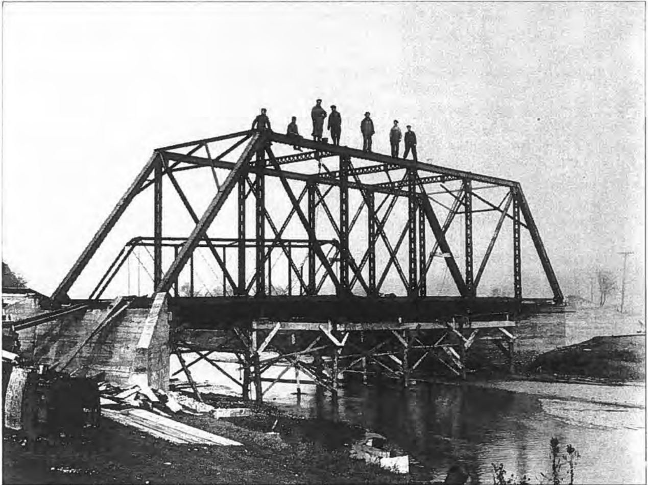
Figure 36: Wausau Iron Works crew erecting a riveted, overhead Pratt truss, New Diggings, Lafayette County, c. 1920. (Source: State Historical Society of Wisconsin, WHi(X3)38359).
