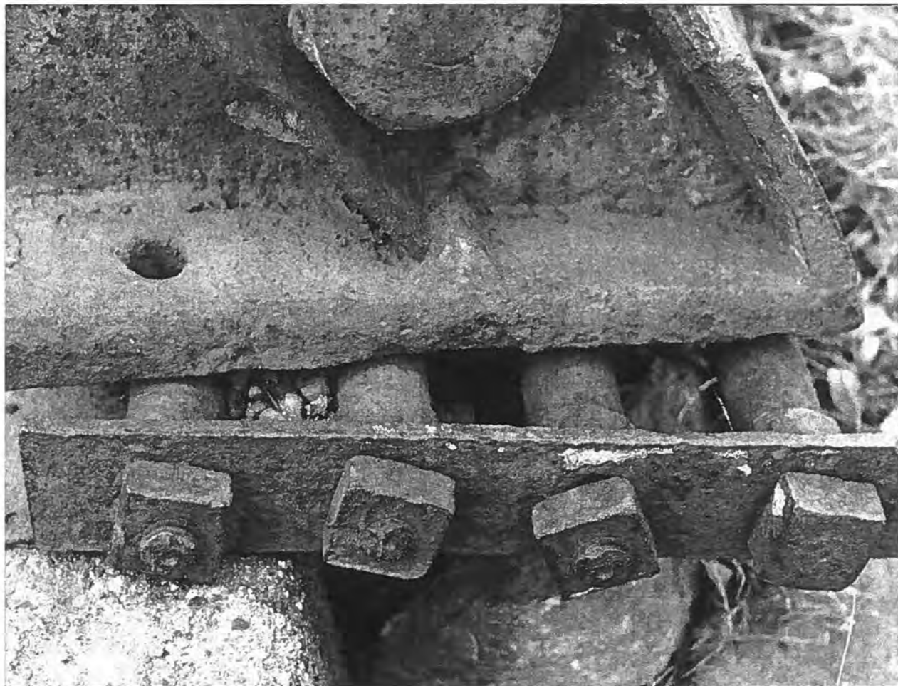
Figure 33: Detail of roller nest expansion bearing, White River Bridge, Burlington, Racine County; erected 1877. (Source: HAER No. WI-16).
