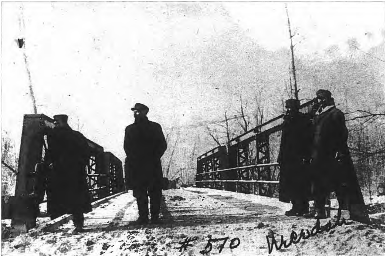
Figure 3: A typical highway, pony truss: Sprague Bridge (P-29-092) in the Towns of Armenia and Necedah, Juneau County; built in 1913 by Elkhart Bridge and Iron Company. (Source: W.E. Gifford, Sr.).
