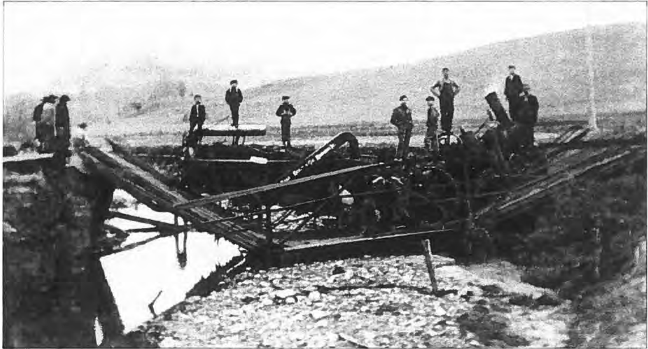
Figure 49: This photograph appeared in an early publication of the Wisconsin Highway Division. Noting that the structure had "failed under a load that should be safe on any bridge built hereafter in the state," the original caption asked the reader to compare "the light flimsy trusses" with bridge "built on plans of the Highway Division." (Source: W.O. Hotchkiss, First Biennial Report of the Highway Division [Madison, 1909], p. 39).
