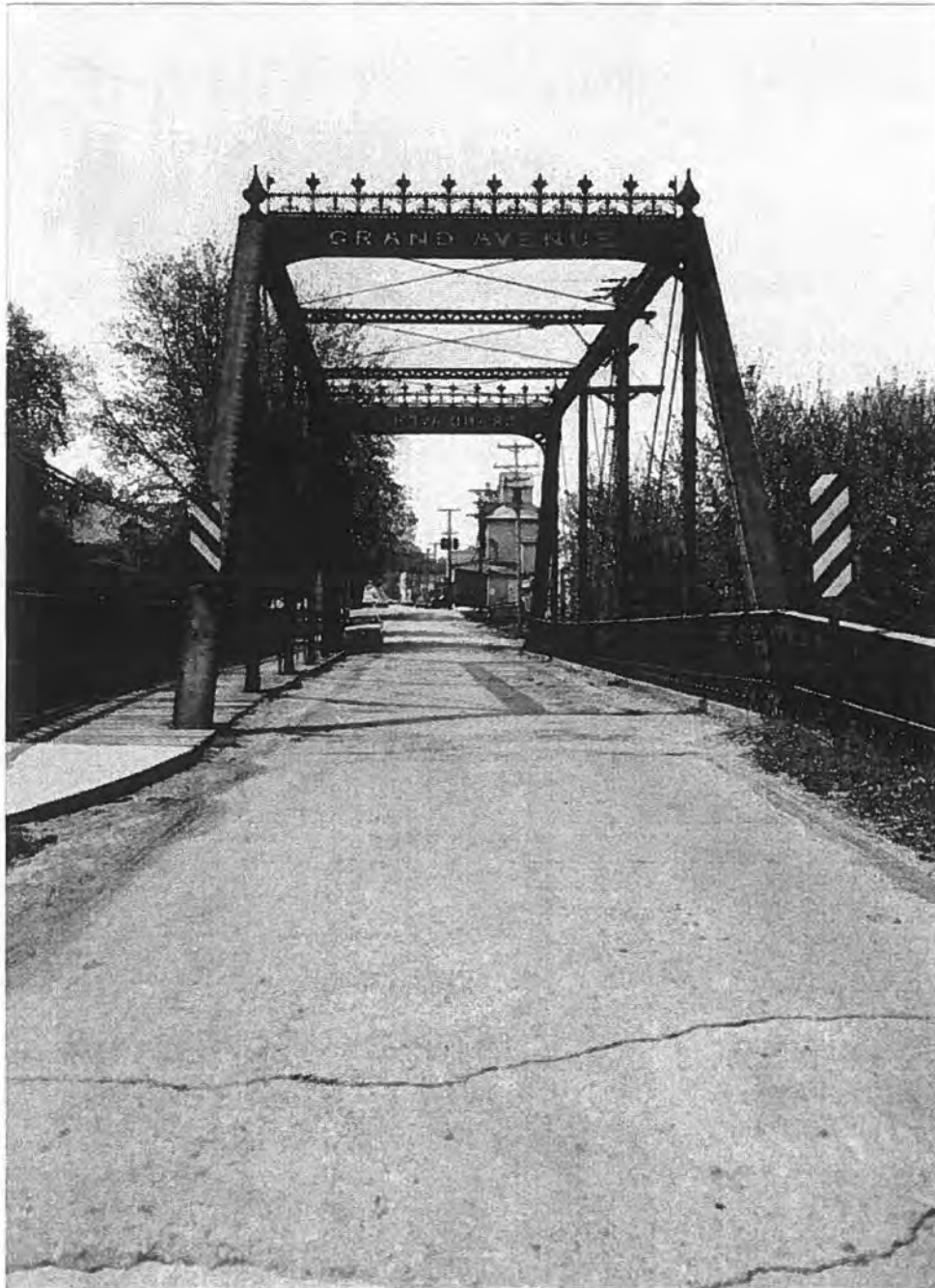
Figure 29: Grand Avenue Bridge, Neillsville, Clark County; overhead Pratt truss, erected 1894; replaced 1986. (Source: HAER No. WI-72).
