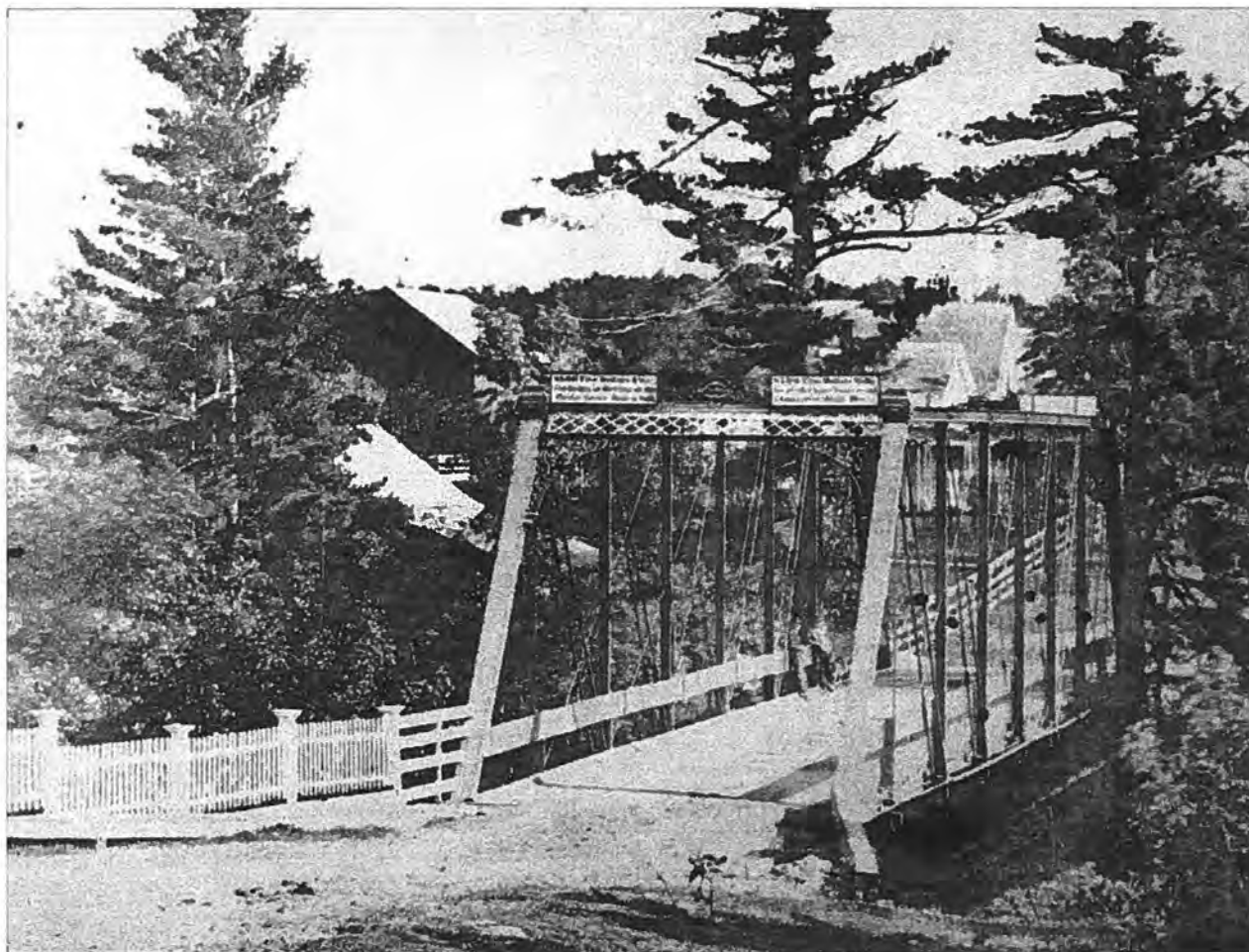
Figure 21: Overhead Pratt truss, River Falls, Pierce County; built in 1876 by Wrought Iron Bridge Company. The double-intersection counters are an unusual feature. (Source: Shepherd Collection, Area Research Center, University of Wisconsin -- River Falls).
