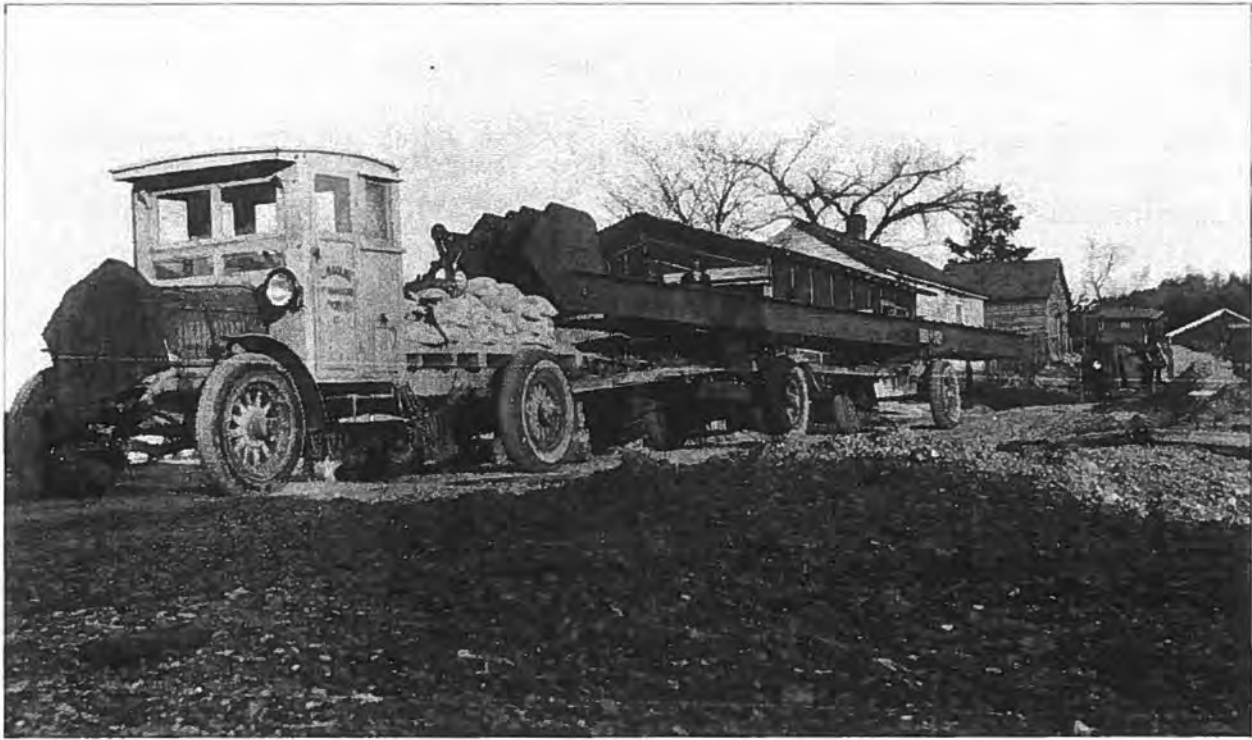
Figure 45: Transporting a bridge section to the site by truck. (Source: State Historical Society of Wisconsin, WHi(X3)43959).
