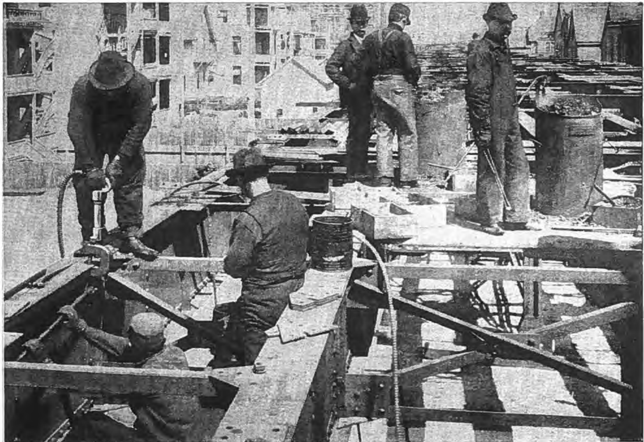
A PNEUMATIC HAMMER DRIVING \frac{3}{8} -INCH RIVETS ON CHICAGO ELEVATED RAILWAY. MADE BY THE CHICAGO PNEUMATIC TOOL COMPANY, CHICAGO
