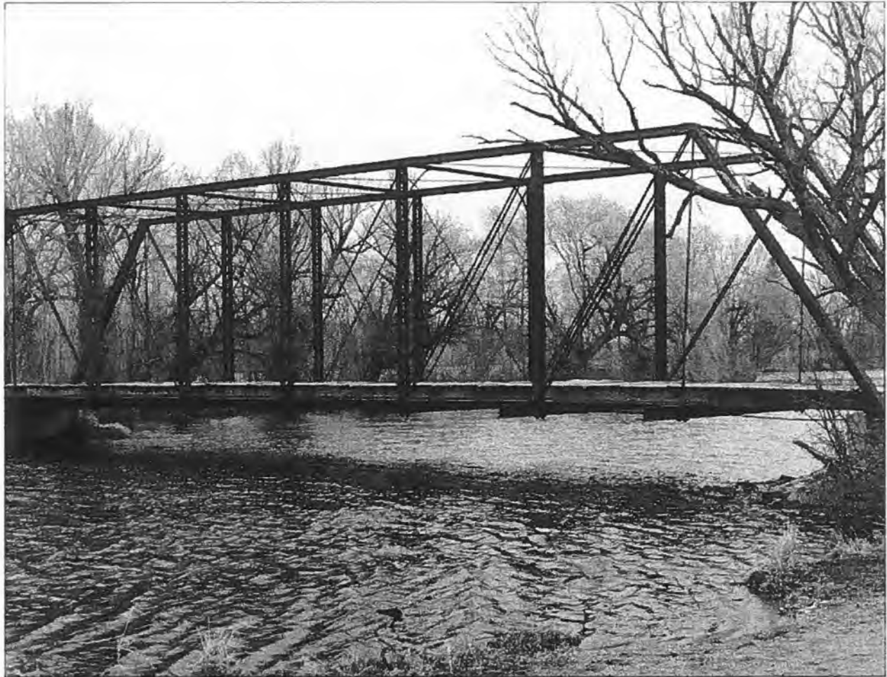
Figure 8: This wrought iron, overhead, Pratt truss was built in downtown Burlington in 1877 by the Milwaukee Bridge and Iron Company. It was moved to its current location on the edge of town over the White River in 1920. It is privately owned. (Source: HAER No. WI-16).
