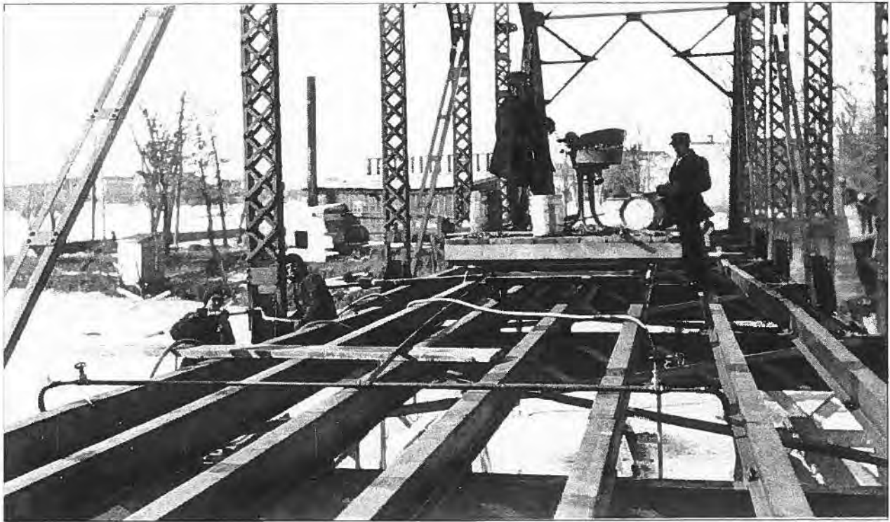
Figure 48: Field riveting a bridge. (Source: State Historical Society of Wisconsin, WHi(X3)43963).
