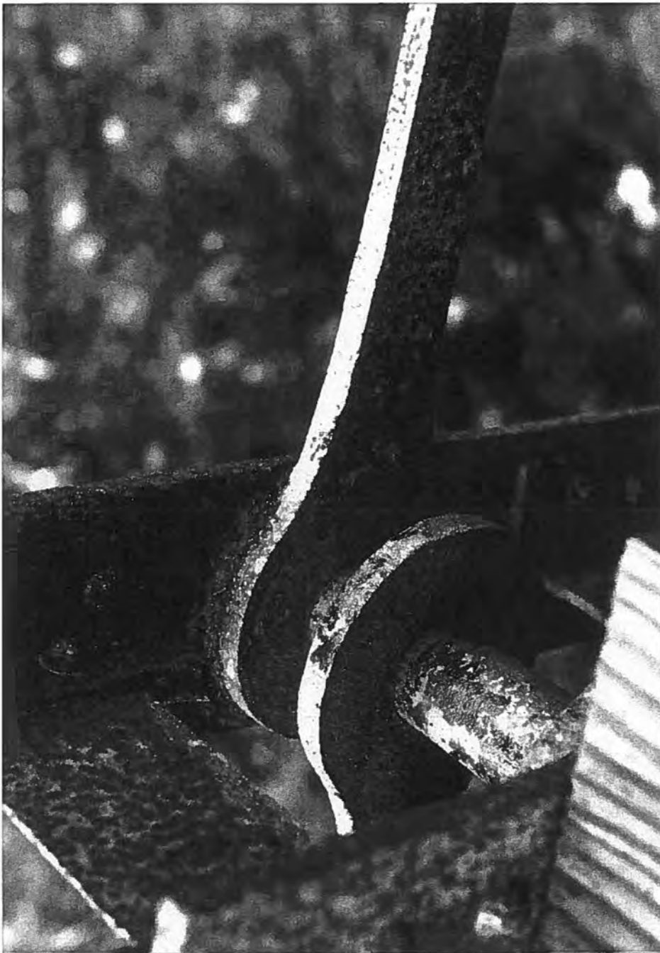
Figure 10: Kloman-type, punched eye-bars; bottom chord of Kelly Road Bridge (P-27-121), built in 1905 over Robinson Creek, Jackson County. (Source: WisDOT).
