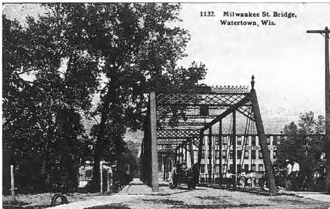
Figure 62: The Milwaukee Street Bridge in Watertown, Wisconsin, displays decorative bridge plates and portals. (Source: Collection of Robert Newbery).
