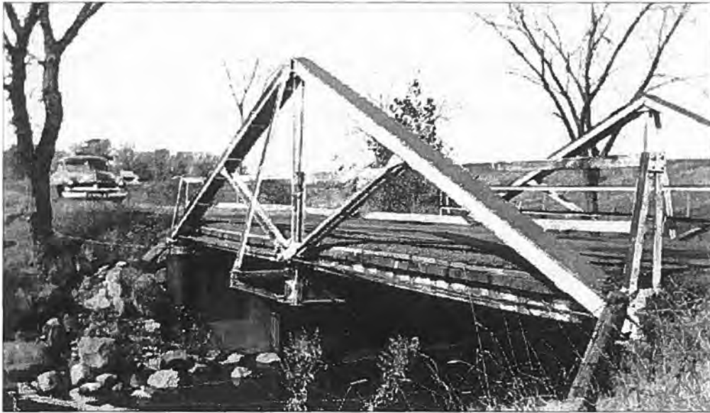
Figure 19: All-metal king post truss, Polk County, 1950; demolished. In this bridge, the traditional king post design has been modified with sub-diagonals, forming a variant known as a "Waddell A Truss." (Source: SHC files, WisDOT).
