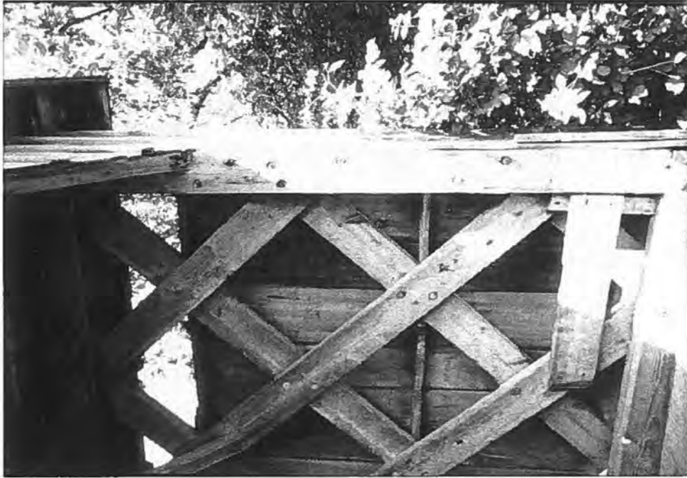
Figure 6: The tree nails are the small circular objects at the intersection of the lattice work; Cedarburg Covered Bridge, Ozaukee County; built in 1876; now closed to vehicular traffic. (Source: WisDOT).
