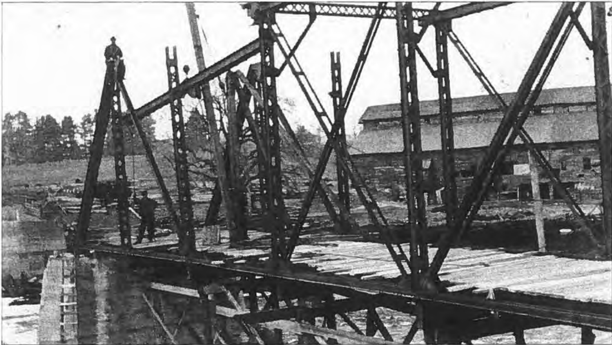
Figure 46: Lifting a top chord member into place by means of a gin pole. (Source: State Historical Society of Wisconsin, Whi(X3)43961).
