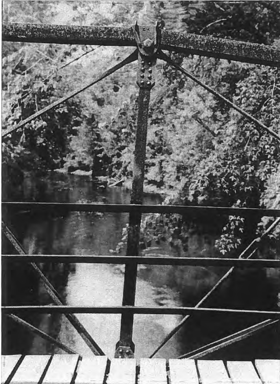
Figure 25: Detail of Charles M. Horton's patented, hanger hook-clip; McGilvray Road Bowstring Truss Bridge No. 1, Van Loon Wildlife Area, La Crosse, Wisconsin. (Source: HAER No. WI-22).
