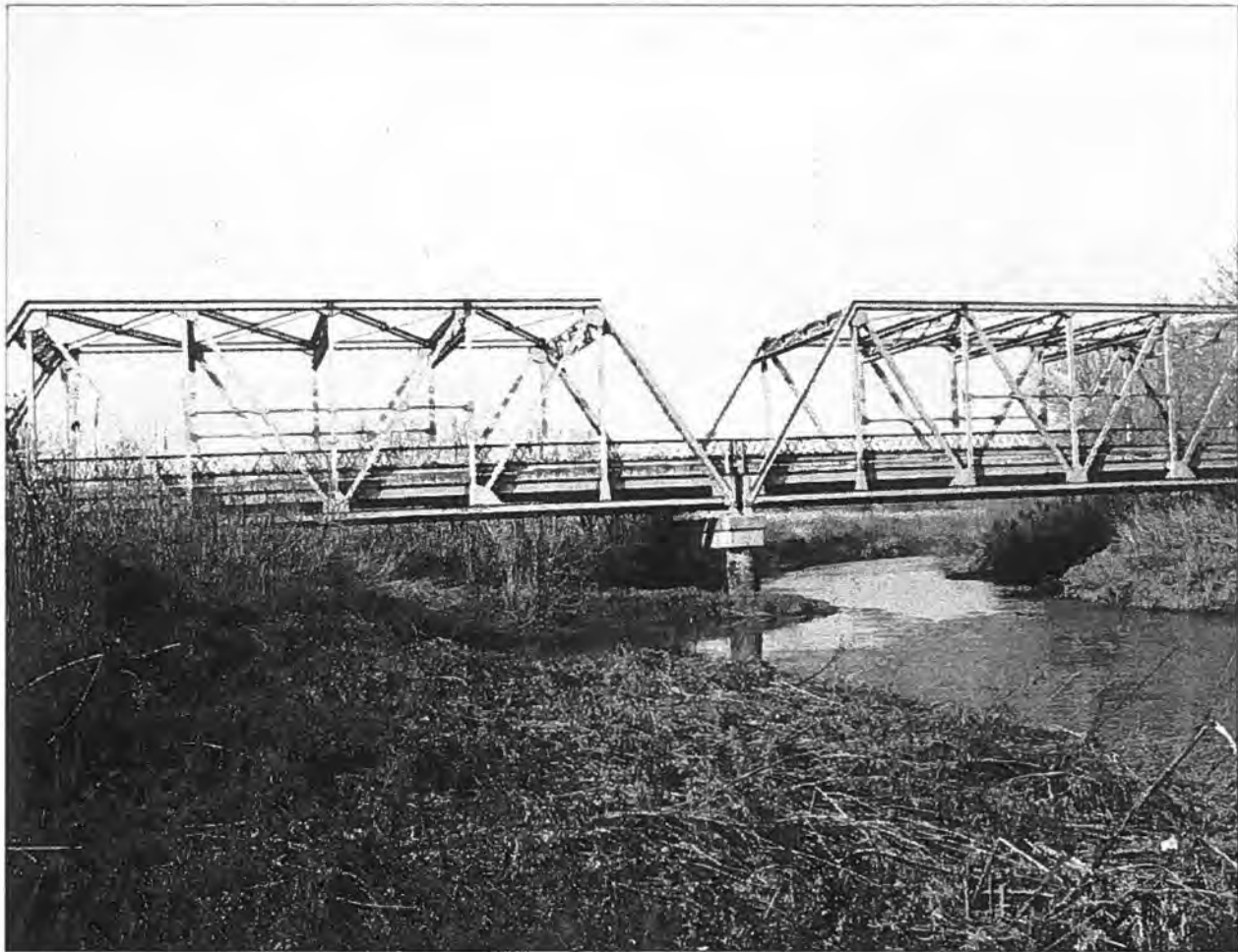
Figure 32: Coulthard Bridge (B-33-204), Town of New Diggings, Lafayette County; double-span overhead Pratt truss, erected 1935. (Source: Robert M. Frame, Field Inventory Photograph, 1986).
