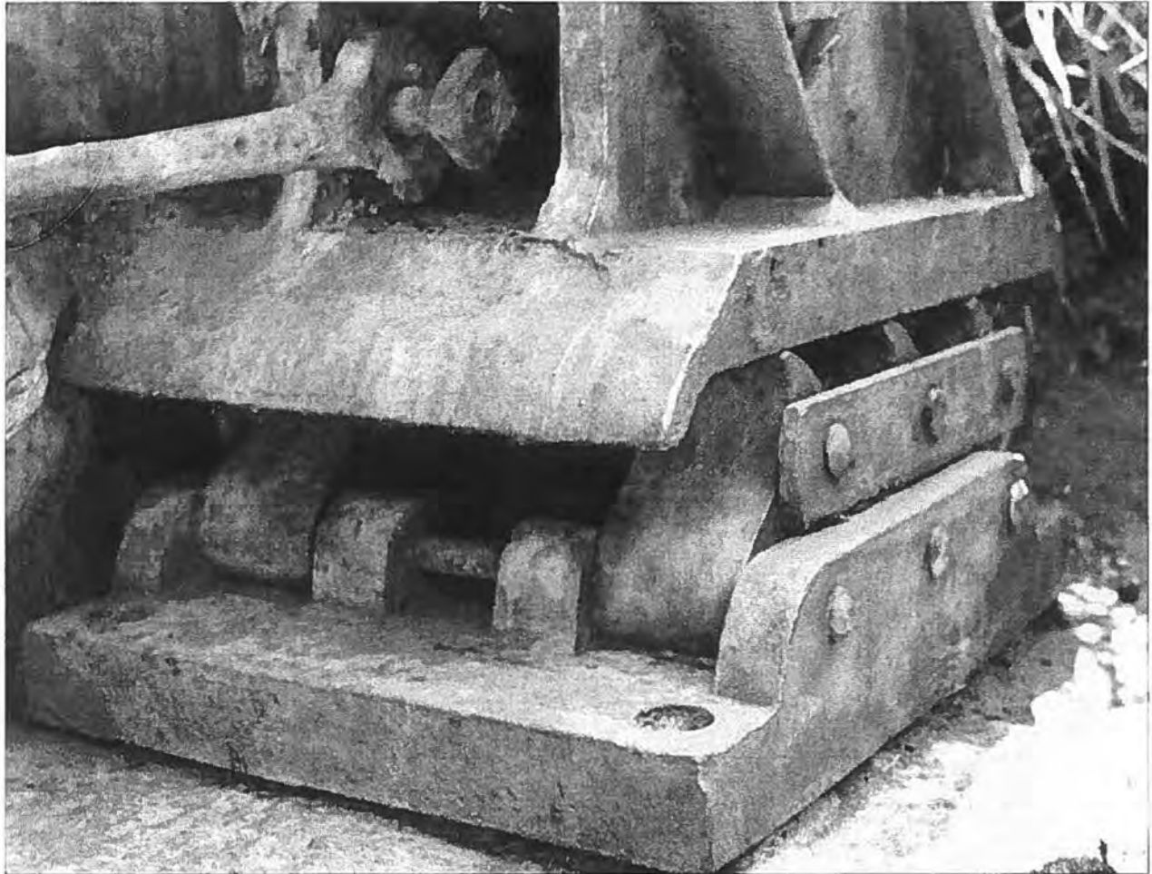
Figure 35: Rocker nest expansion bearing, Gill Road Bridge, Dodge County. This unusual bearing combines the attributes of the rocker and roller nest designs. (Source: SHC files, WisDOT).
