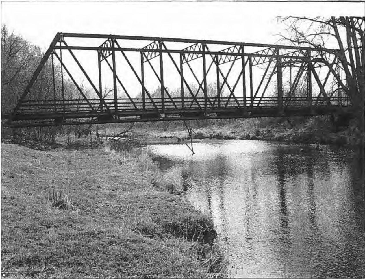
Figure 11: Riveted construction; Wagon Trail Road Bridge (B-47-006) built in 1909 over Eau Galle River, Pierce County. (Source: HAER No. WI-31).
