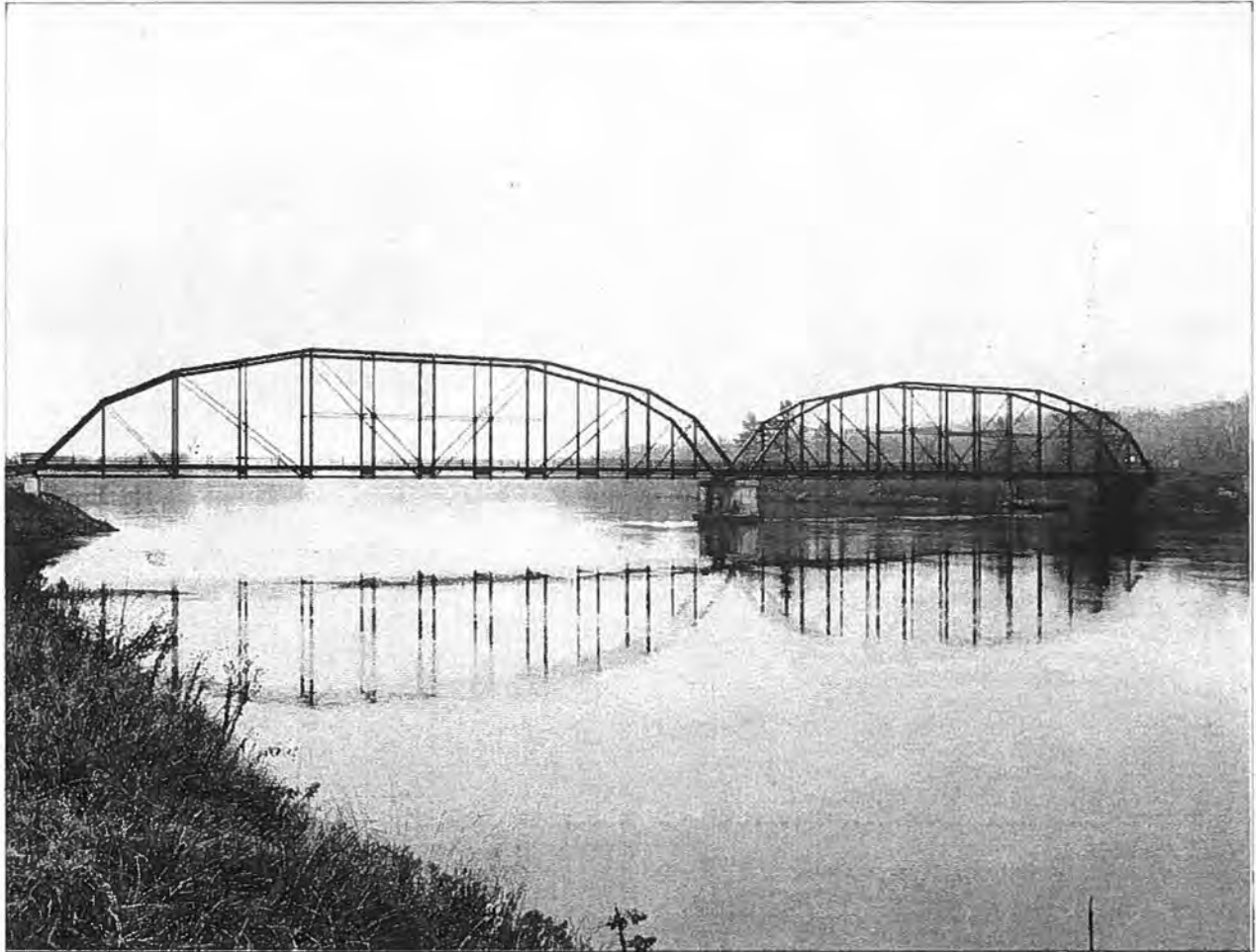
Figure 23: Cobban Bridge (B-09-965) over Chippewa River, Towns of Arthur and Eagle, Chippewa County. Originally erected in 1908 at a site about 15 miles downstream, this double-span Pennsylvania truss bridge was moved to its present location in 1919. (Source: Jeffrey A. Hess, Field Inventory Photograph, 1986).
