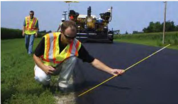
Edge improves the compaction of the pavement near the edge. Shoulders should still be pulled up flush with the pavement. The installation of a safety edge showed reductions of more than 5 percent of total crashes<sup>28</sup>.
