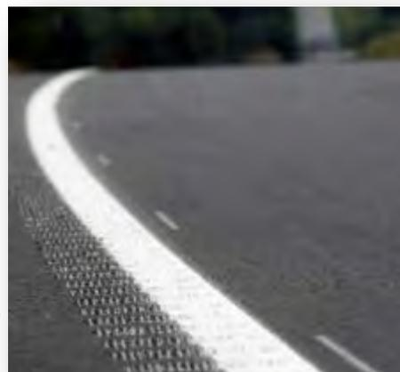
The installation of shoulder rumble strips is expected to result in a crash reduction of 36 percent for Run off Road crashes, excluding PDO crashes. If edgeline rumble stripes are installed the crash reduction increases to 39 percent for Run off Road crashes, excluding PDO crashes.
