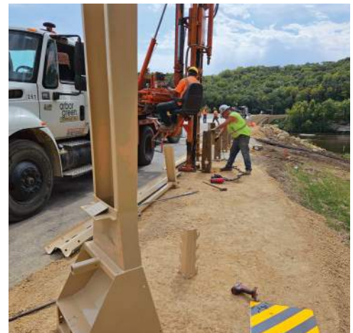
Arbor Green, Inc. : Guardrail install
