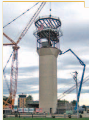
Wittman Regional Airport Air traffic control tower under construction
