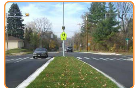
Mineral Point Road and South Owen Drive after the addition of a median, pedestrian signal, and painted crosswalk. Photo by WisDOT SRTS
