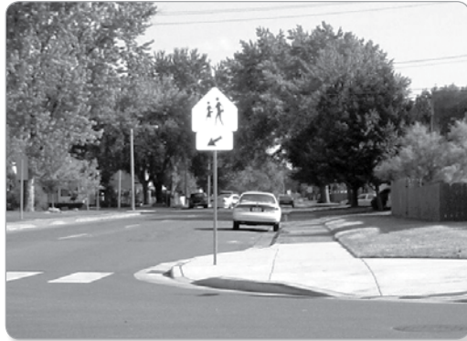
Responding to concerns about unsafe crossings, Eau Claire constructed curb extensions like the one pictured above. The new design reduces traffic speed, makes pedestrians more visible to cars and lessens the crossing distance, all of which increase pedestrian safety.
