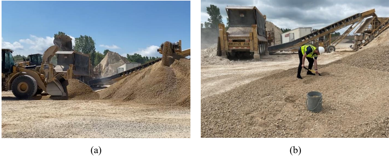
Figure 3.3 Typical aggregate sampling: (a) sampling pad preparation by loader, (b) sampling from the pad
