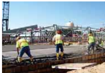
US HIGHWAY 41 WORK CREW
