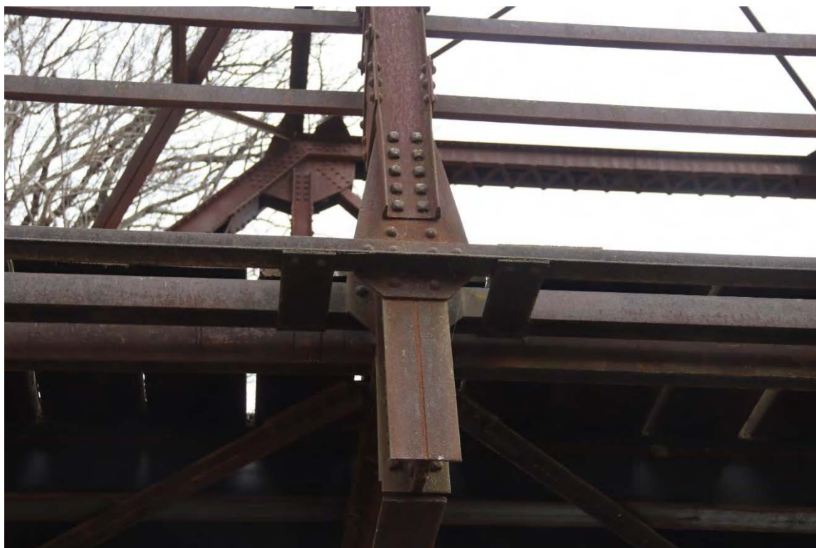
Figure 11. Bottom chord details, view facing northeast.
