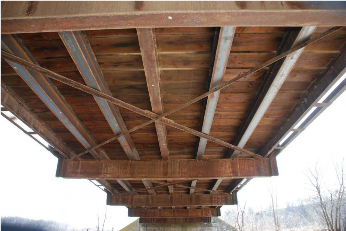
Figure 8. Steel floor beams and stringers, view facing southeast.
