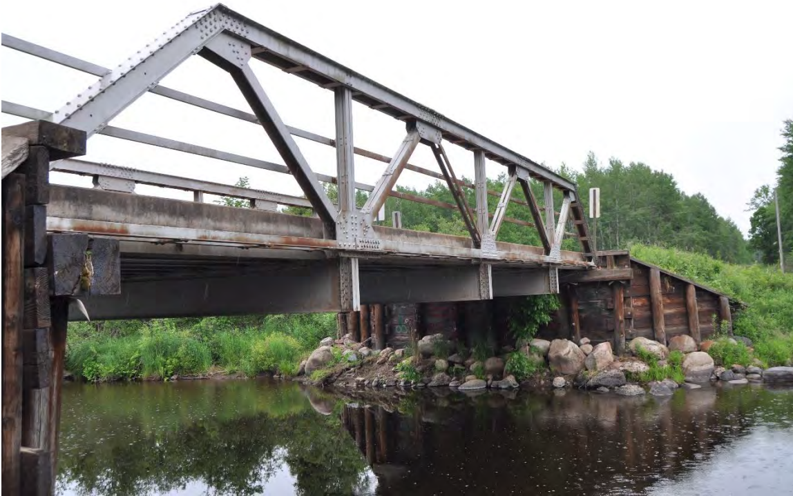
Photo 2 of 4. P-50-0091, P-50-0091, east elevation and substructure, looking northwest.
