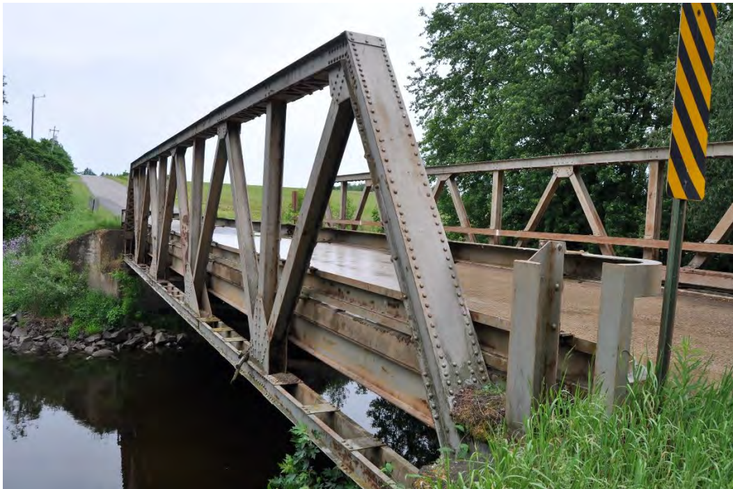
Photo 1 of 3: Meridian Road Bridge (P-37-0190), west elevation, looking northeast.
