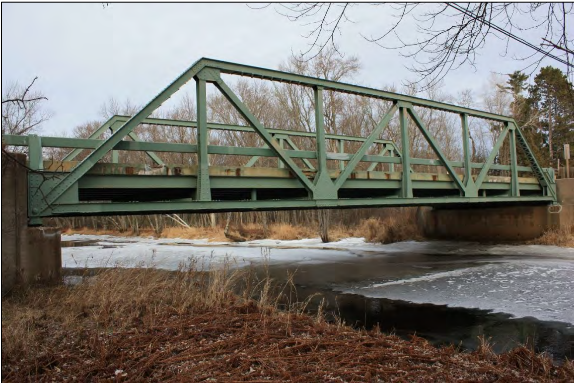
B-19-509, Overview of north span, facing southwest.
