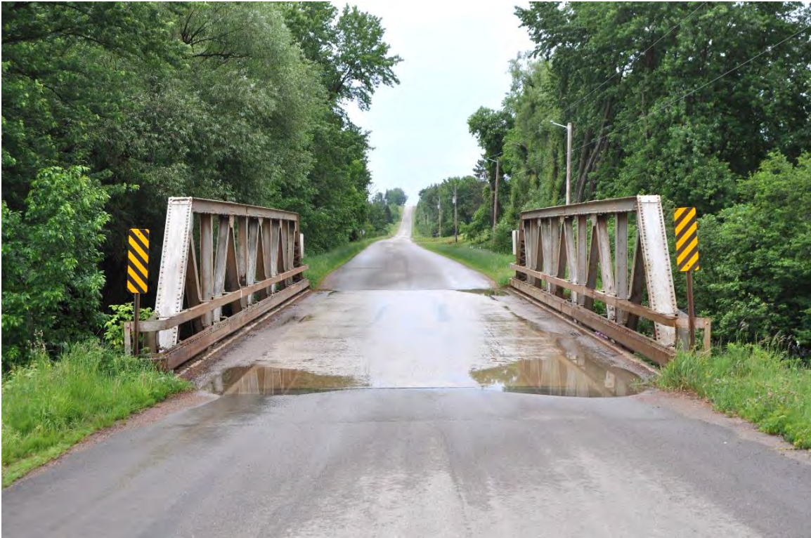
Figure 4. Approach to the Meridian Road Bridge, view facing south.
