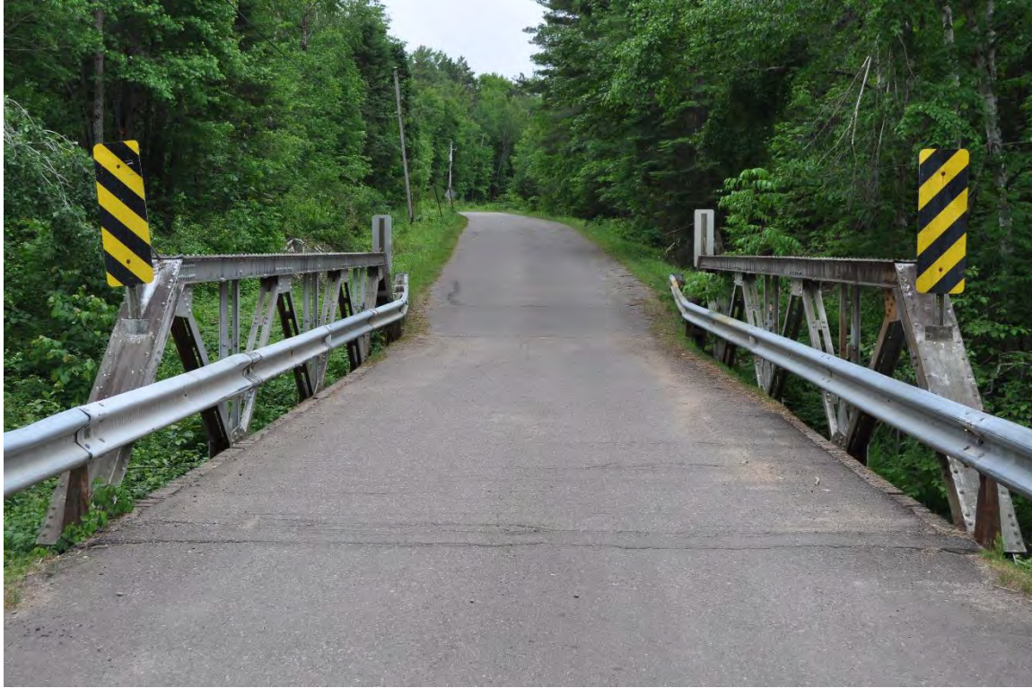
Photo 1 of 4. P-54-0906, overview of bridge from north approach, looking south.
