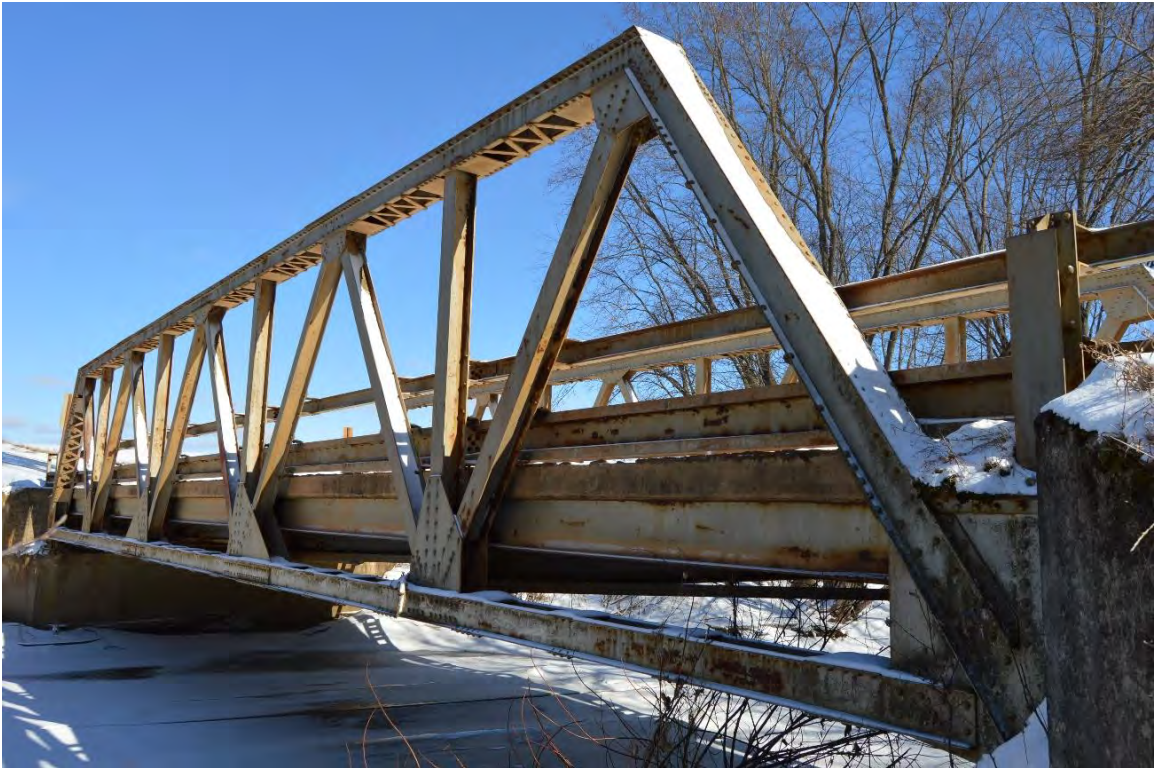
Figure 6. East side of the Meridian Road Bridge, view facing southwest.
