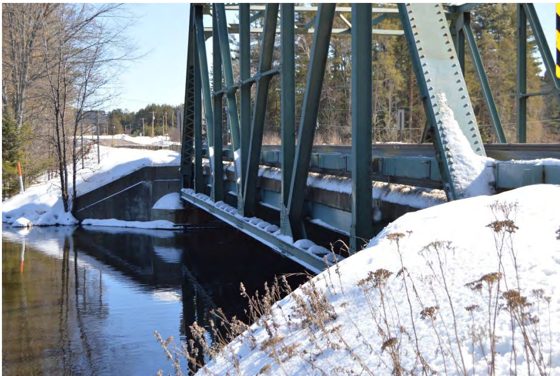
B-35-0067, looking SE
