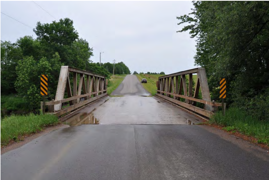
Photo 3 of 3: Meridian Road Bridge (P-37-0190), south approach, looking north.
