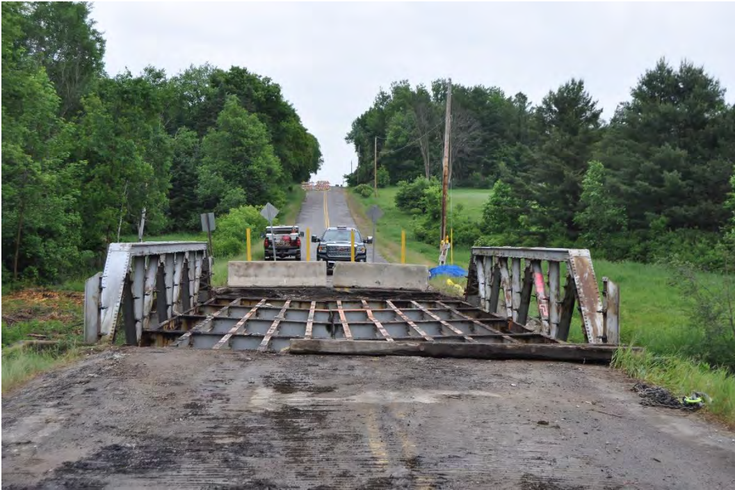
Stettin Drive Bridge (P-37-0203), west approach, looking east.
