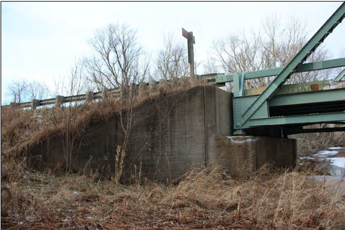
B-19-509, Concrete abutment and wingwall, facing south from Pine River.
