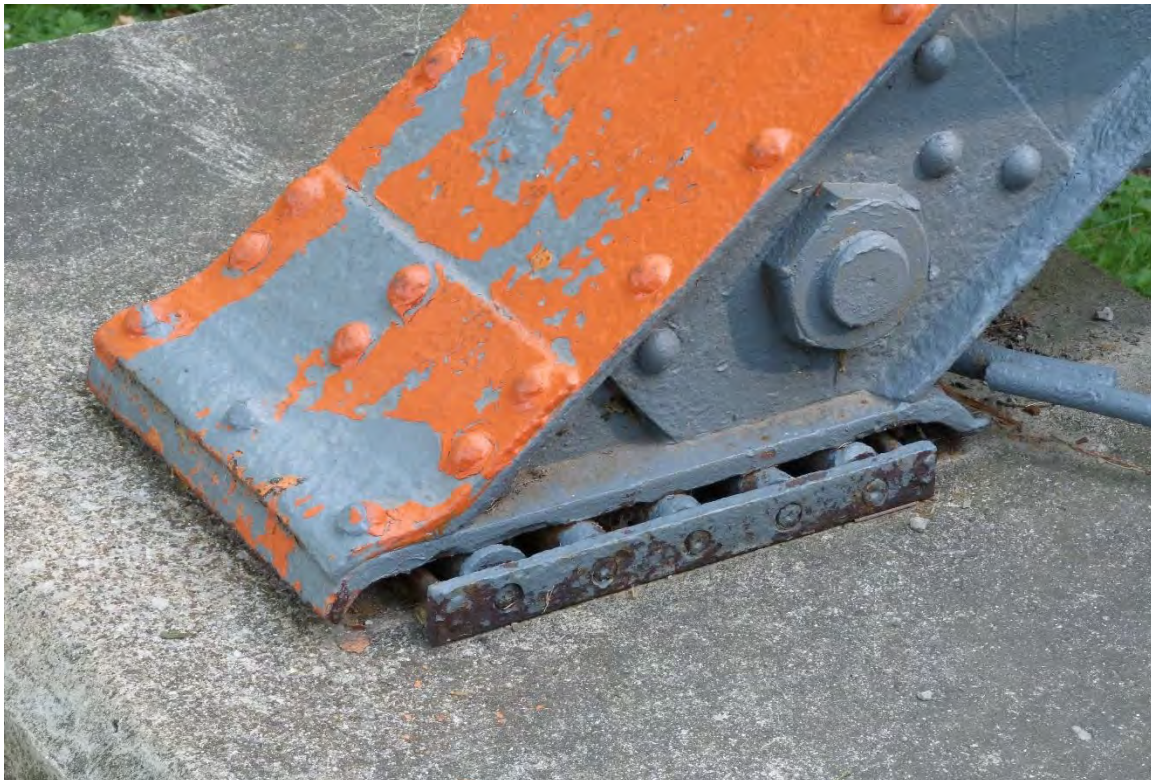
Figure 15. Roller-nest expansion bearing. Photo courtesy of Historic Bridges.
