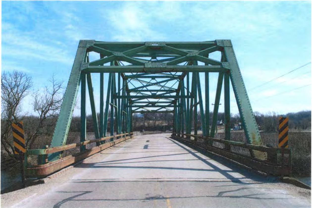
B-33-625 View facing West
