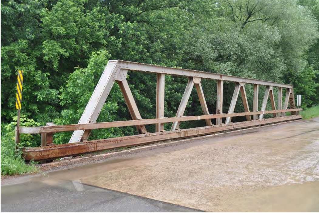
Photo 2 of 3: Meridian Road Bridge (P-37-0190), interior of east truss, looking east.
