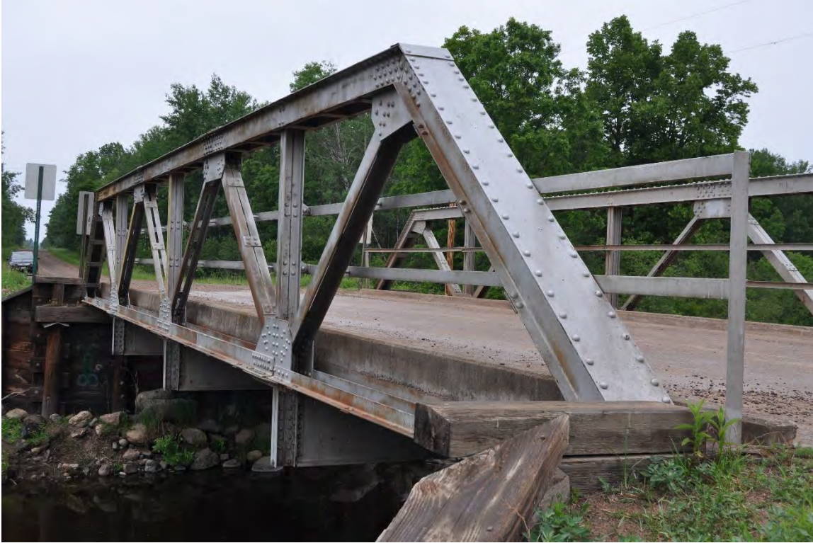
Photo 3 of 4. P-50-0091, east elevation, looking northeast.
