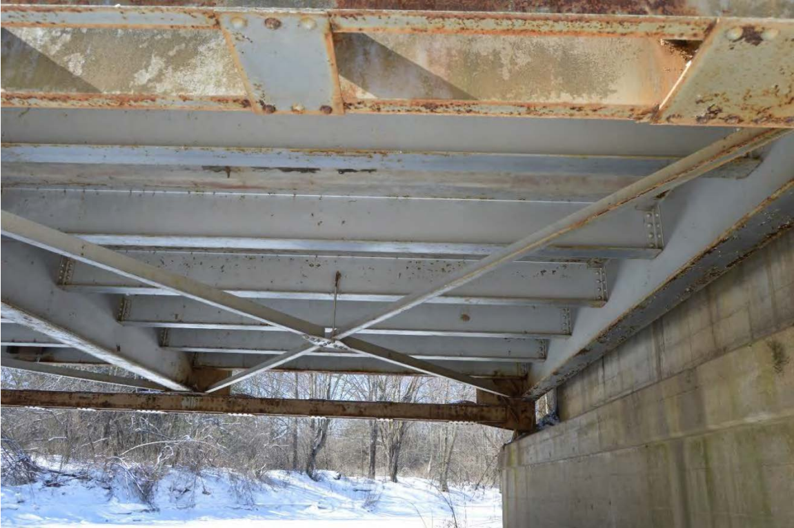
Figure 9. Floor beams and stringers, view facing west.
