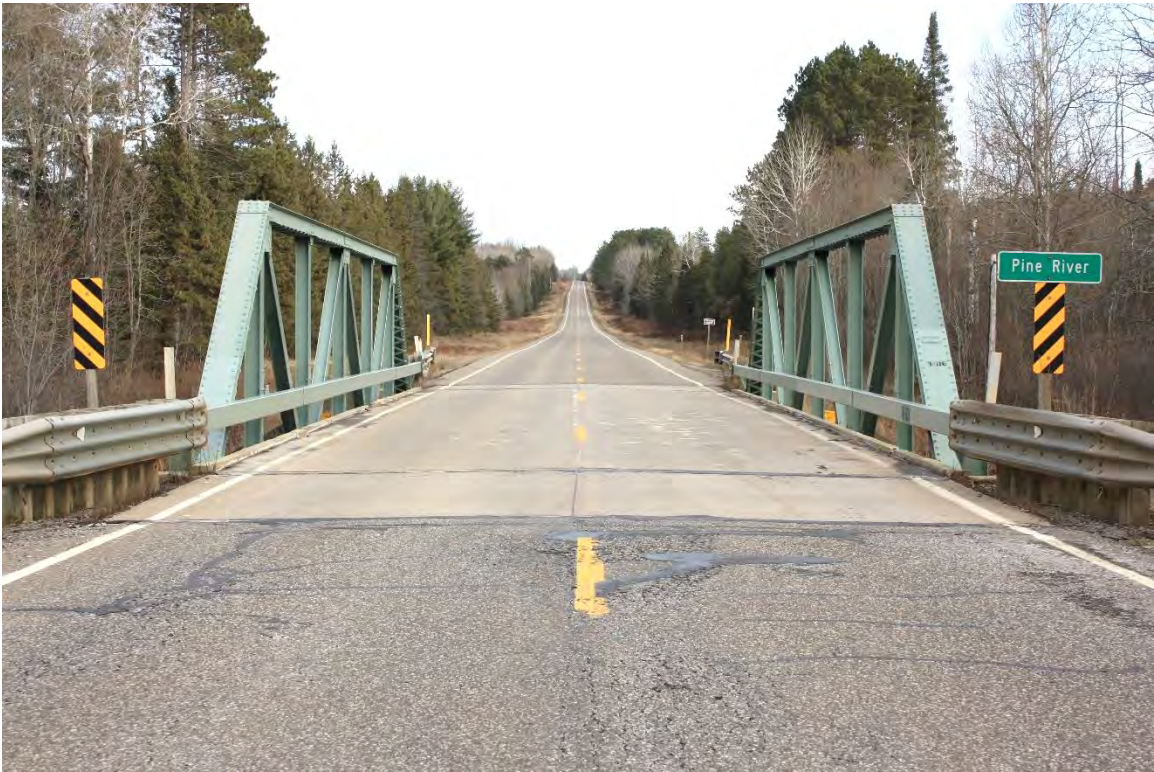
Figure 19. Replacement concrete deck on the Pine River Bridge (AHI No. 245691, B-19-0509), 1939.
