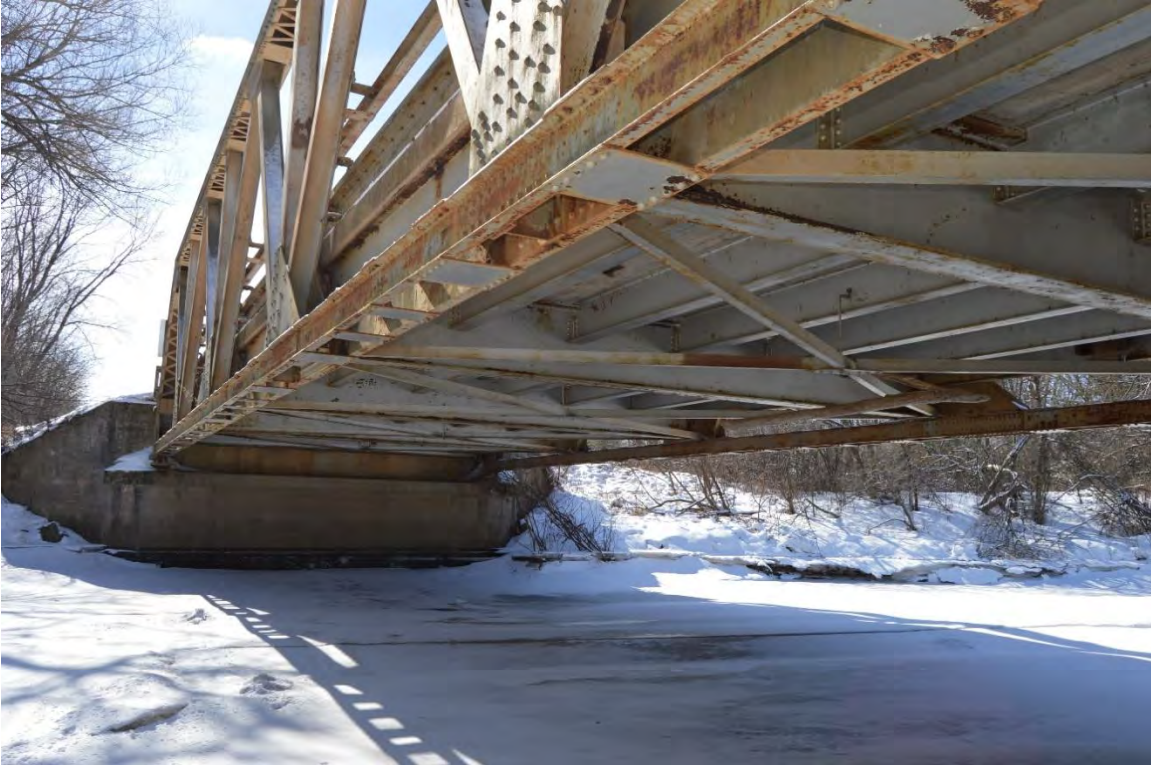
Figure 8. Bottom chord details and concrete abutment, view facing southwest.
