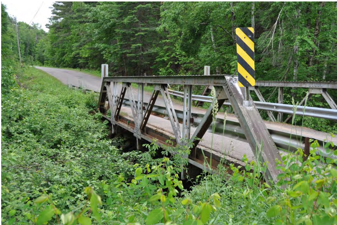
Photo 2 of 4. P-54-0906, east elevation, looking southwest.
