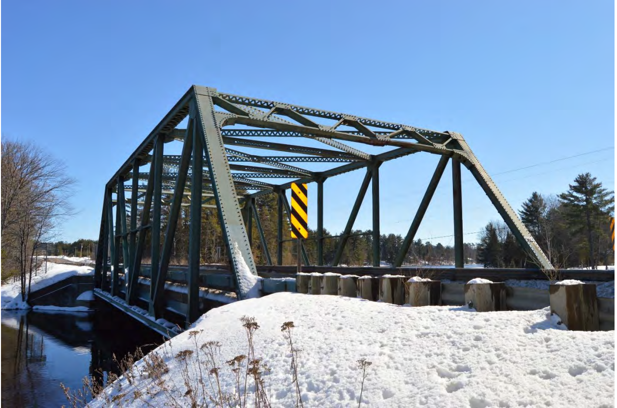
B-35-0067, looking SE
