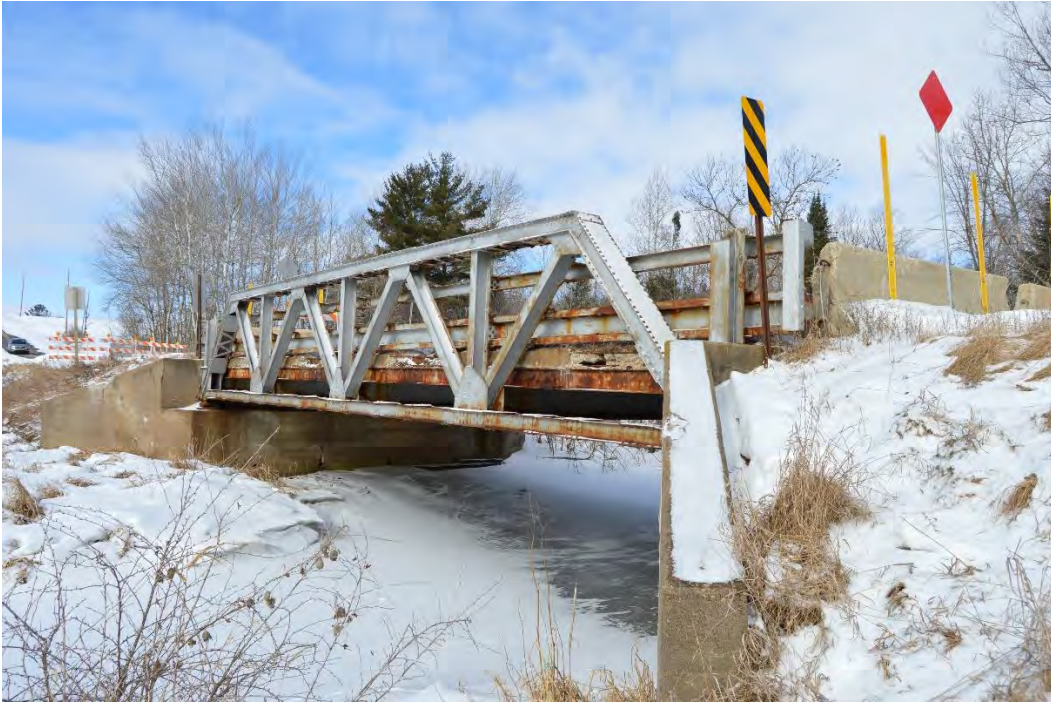
Stettin Drive Bridge (P-37-0203), south elevation and concrete substructure, looking northwest.
