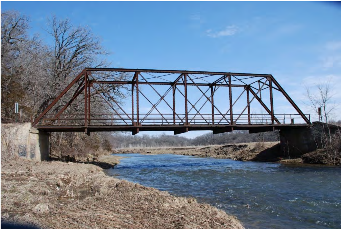
Figure 6. The Richardson Bridge, view facing northeast.
