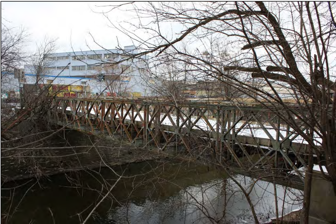
P-40-0658, Overview of west span, facing northeast.
