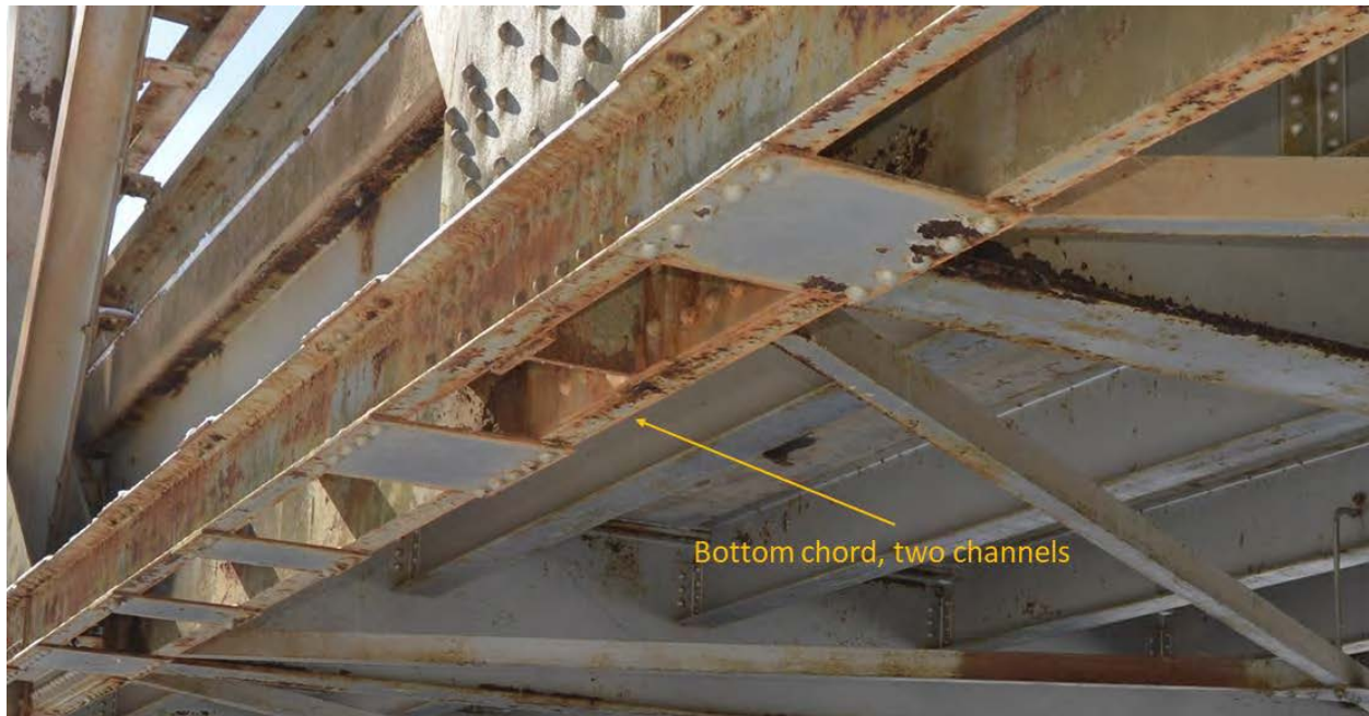
Figure 2. Meridian Road Bridge bottom chord details.
