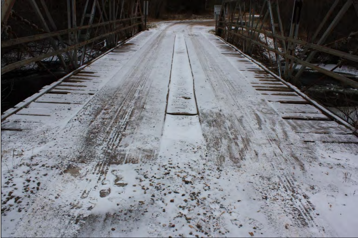
P-19-0013, Timber stringer and wood plank decking, facing east.
