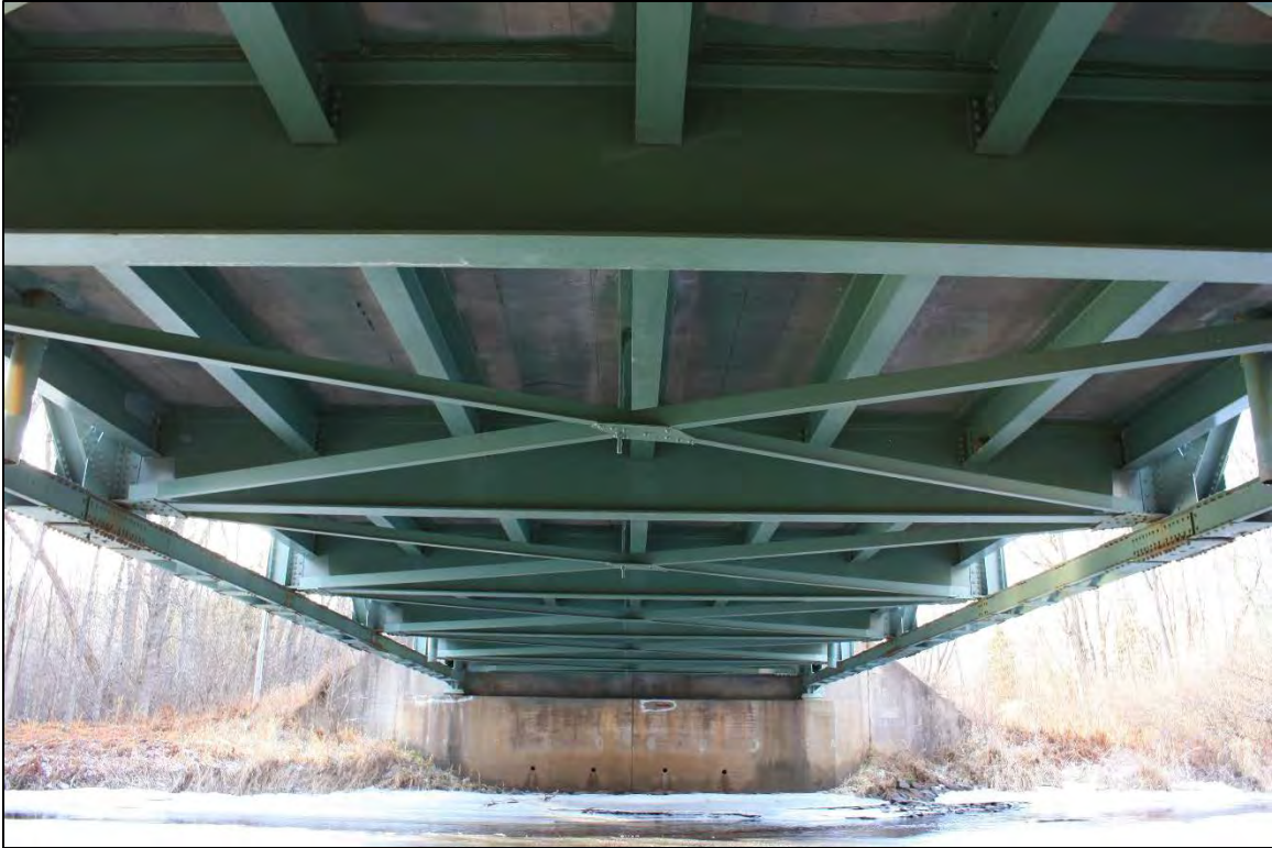
B-19-509, Underside of superstructure, facing east.
