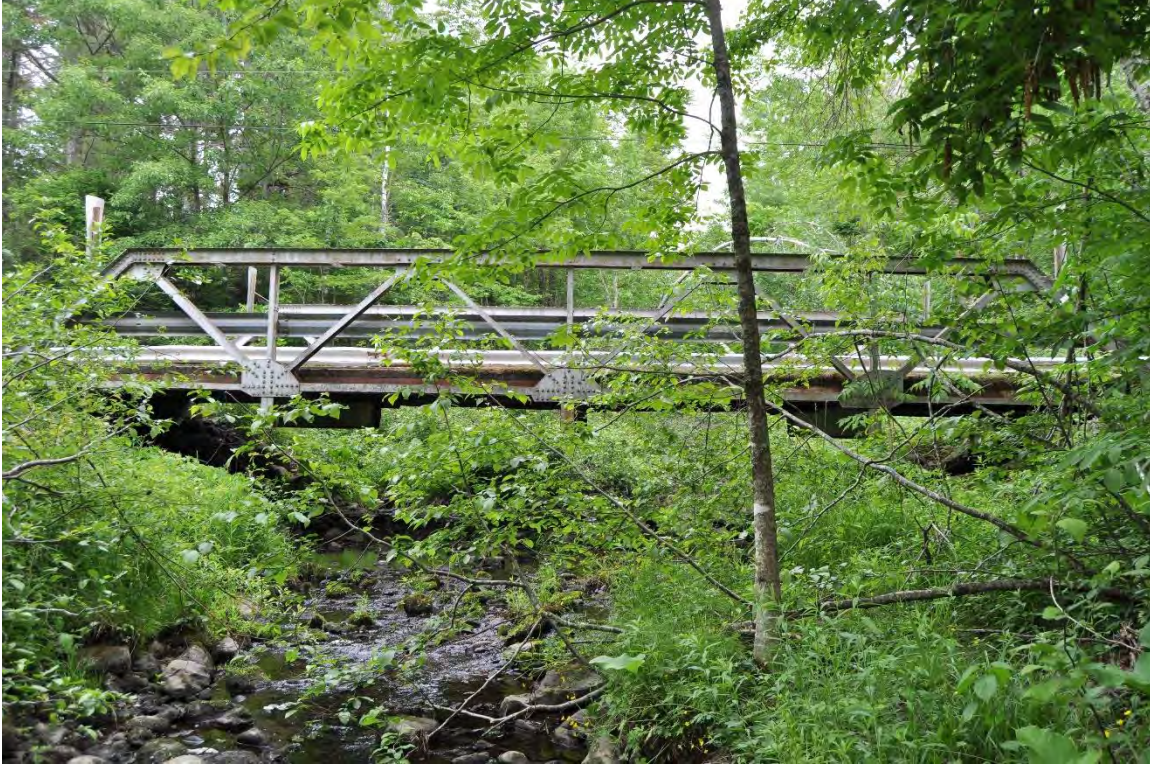
Photo 3 of 4. P-54-0906, west truss, facing east.
