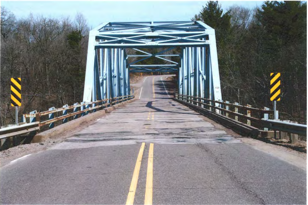
B-18-001 View Looking South
