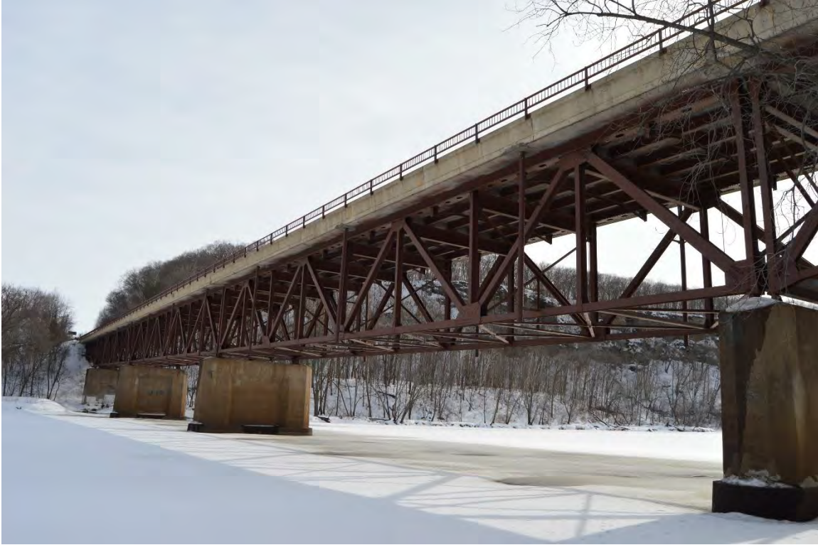
B-48-0224, looking SE
