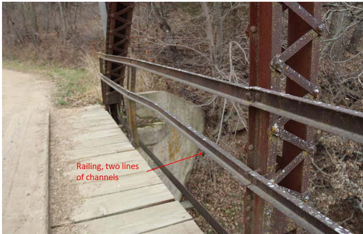
Figure 4. Richardson Bridge railing details.
