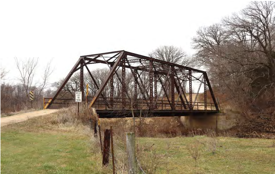
Figure 5. The Richardson Bridge, view facing west.
