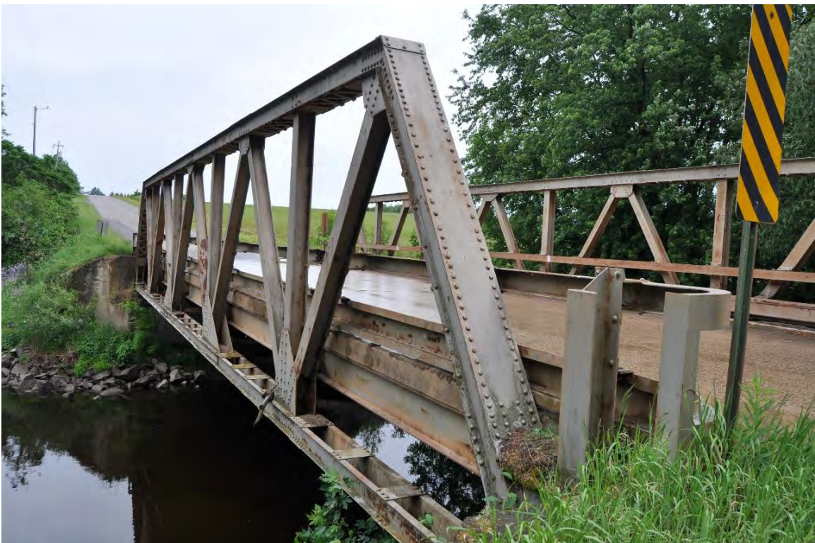
Figure 5. West side of the Meridian Road Bridge, view facing northeast.
