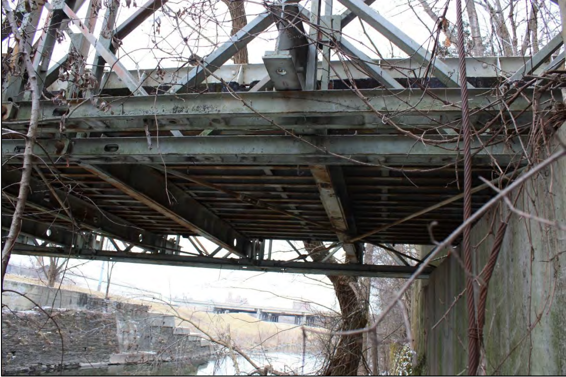
P-40-0658, Underside of superstructure, facing east.
