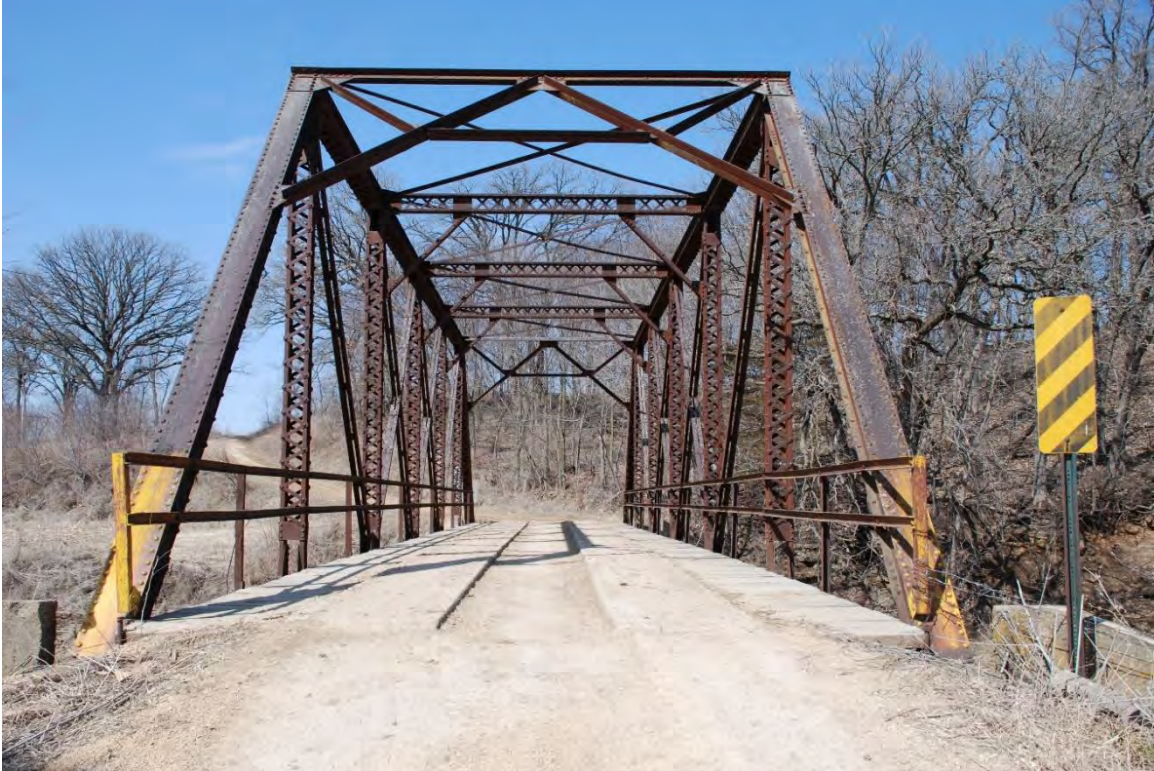
Figure 7. Approach to the Richardson Bridge and portal bracing, view facing northwest.
