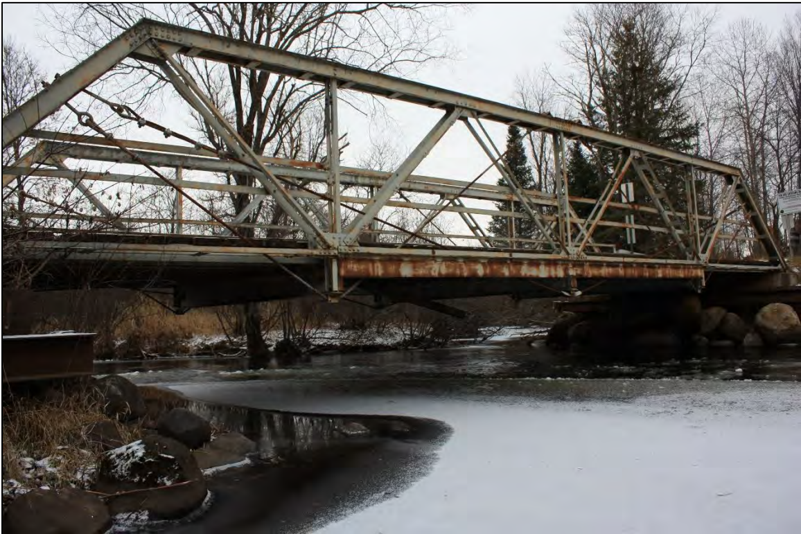
P-19-0013, Overview of south span, facing northeast.
