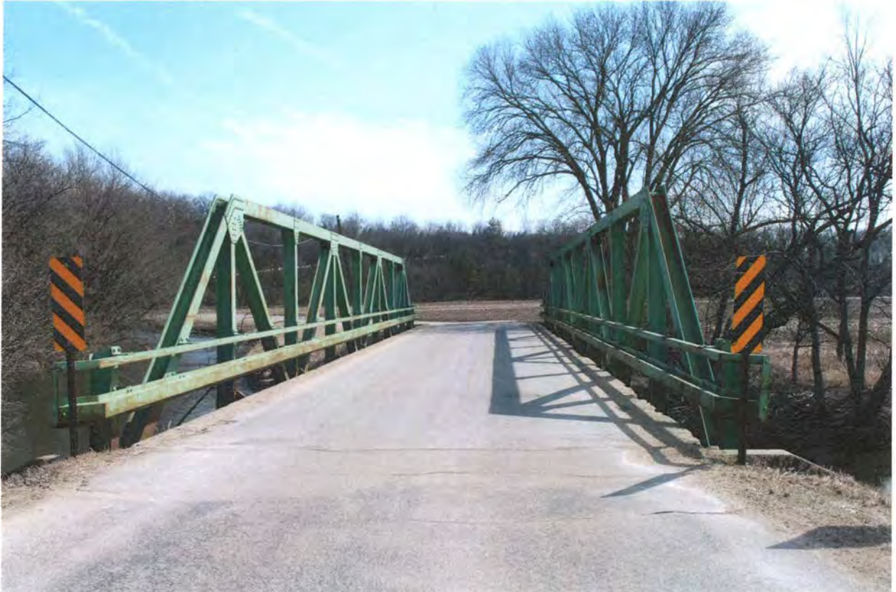
B-33-002 View Facing East
