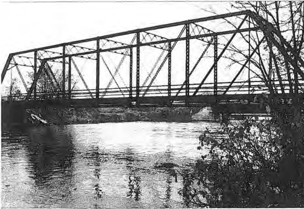
Van Laenen Road Bridge (P-42-081), Town of Stiles, Oconto County West elevation - Source: J.A. Hess, 1986
