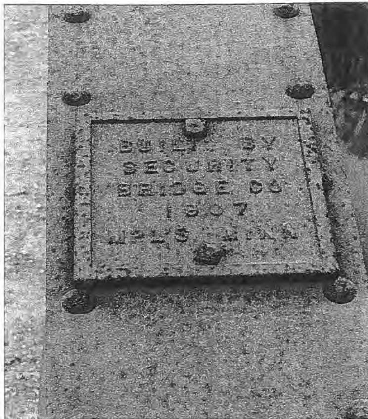
Broken Arrow Road Bridge (P-54-125), Town of Willard, Rusk County Detail of bridge plate on inclined endpost - Source: J.A. Hess, 1986
