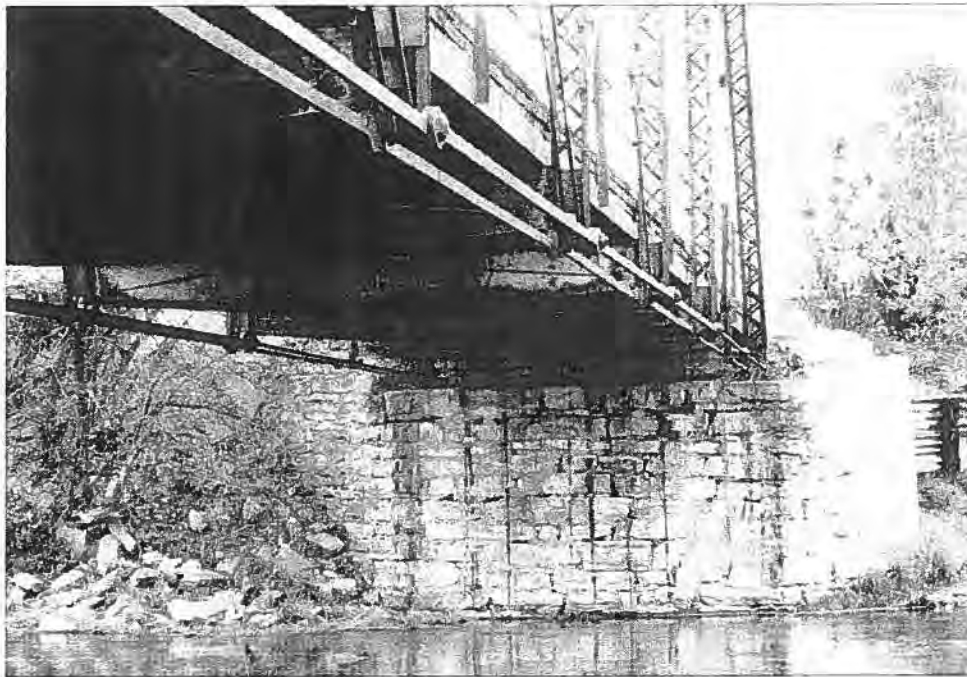
Mill Road Bridge (P-36-022), Town of Manitowoc Rapids, Manitowoc County North abutment - Source: J.A. Hess, 1986
