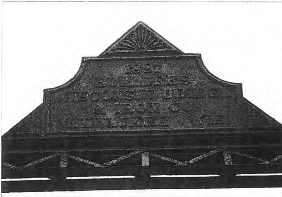
Mill Road Bridge (P-36-022), Town of Manitowoc Rapids, Manitowoc County Top: South approach - Source: J.A. Hess, 1986 Bottom: Detail of builder's plate - Source: J.A. Hess, 1986
