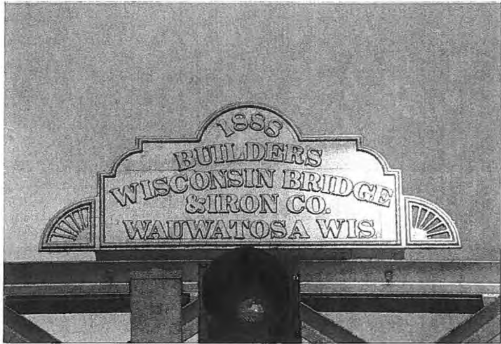
Bridge Street Bridge (P-45-700), Village of Grafton, Ozaukee County Bridge plate, west portal - Source: J.A. Hess, 1986
