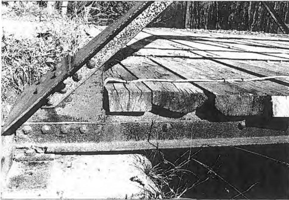
Iron Bridge Road Bridge (P-42-901), Town of Armstrong, Oconto County Detail of northeast endpost connection - Source: J.A. Hess, 1986
