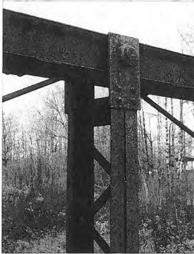
Broken Arrow Road Bridge (P-54-125), Town of Willard, Rusk County Detail of top chord and northeast pin, south side of north elevation - Source: J.A. Hess, 1986
