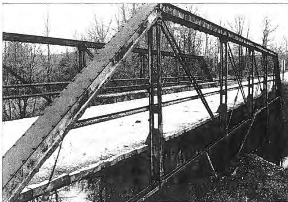
Branch River Bridge (P-36-116), Town of Franklin, Manitowoc County
