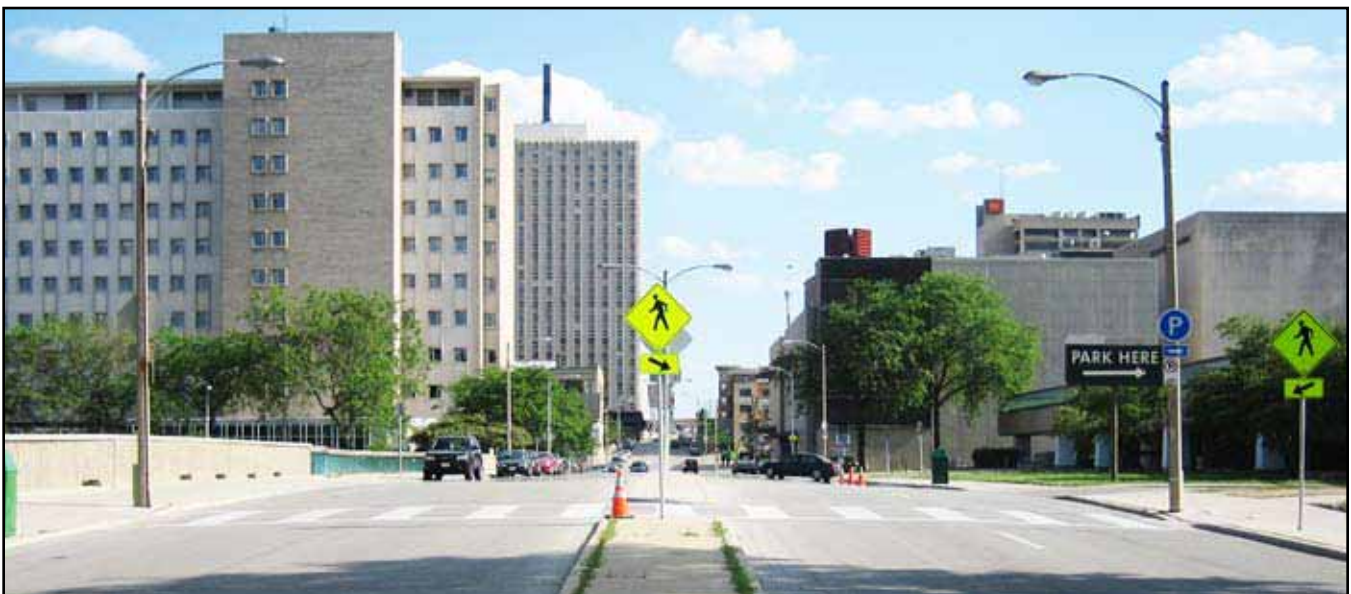
Exhibit 5-59: Mid-block crosswalks should have highly visible pavement markings and appropriate signage to alert motorists.
