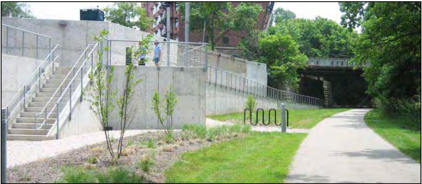
Exhibit 5-79: An accessible ramp is required to connect the grade-separated pedestrian facility to the sidewalk, but stairs may also be constructed to provide more direct access.
