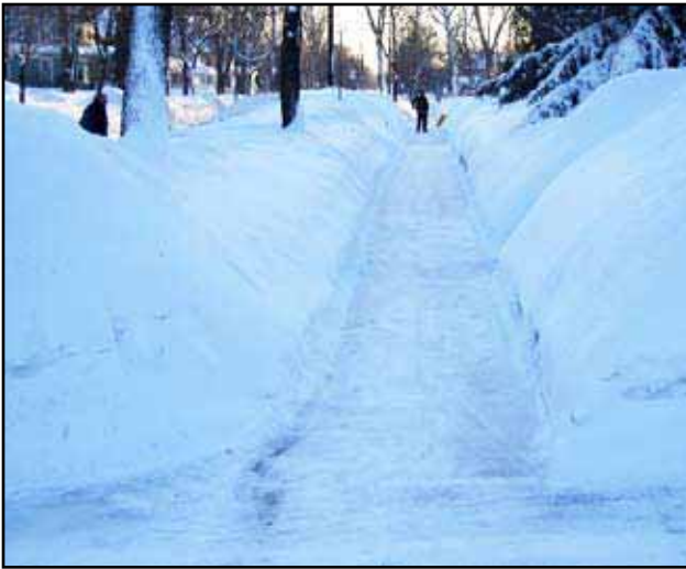
Exhibit 5-10: In Wisconsin, horizontal separation between the sidewalk and the roadway provides needed space for snow storage.
