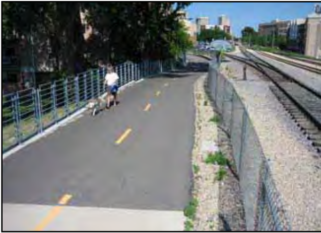
Exhibit 5-92: Some communities have had success incorporating pedestrian pathways alongside rail corridors, although considerable coordination with the rail company is necessary.
