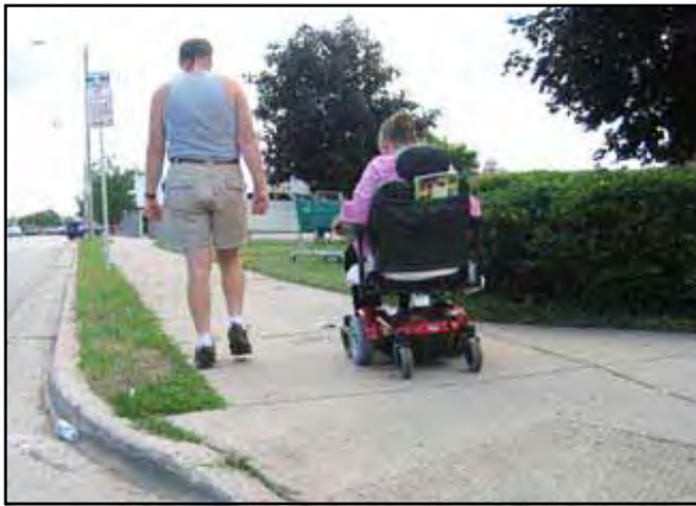
Exhibit 5-25: Side flares and cross slopes can be problematic for some pedestrians. In this example, an easement is provided for pedestrians to maneuver around the flare.
