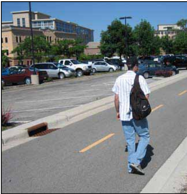
Exhibit 88-5 t: Well-placed drainage grates are located outside of the walking area so they do not interfere with pedestrian travel.
