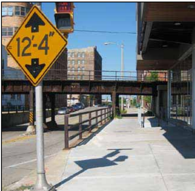
Exhibit 5-77: Where the sidewalk is located above the roadway grade, a railing must be provided.
