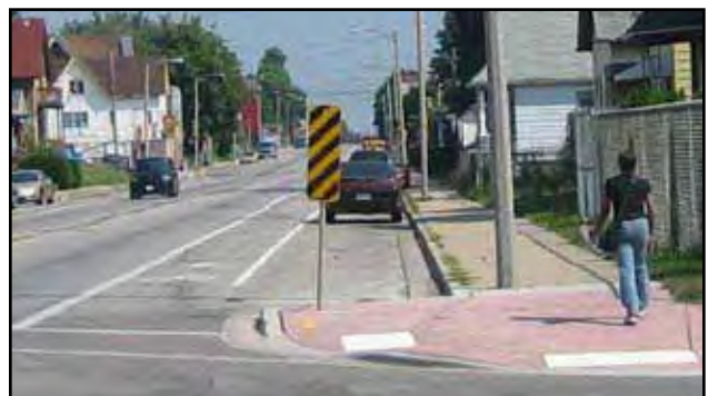
Exhibit 5-70: Since curb extensions stretch the width of the parking lane, signage or street furniture must be placed on the curb extension to alert drivers and plows.
