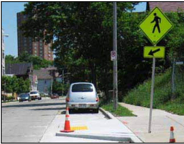
Exhibit 5-61: Curb extensions and parking restrictions should be incorporated into the design of a mid-block crosswalk in conjunction with on-street parking.
