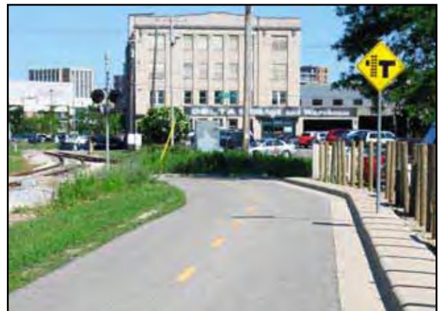
Exhibit 5-72: If necessary, the walking area should curve to avoid crossing railroad tracks at an angle less than perpendicular.
