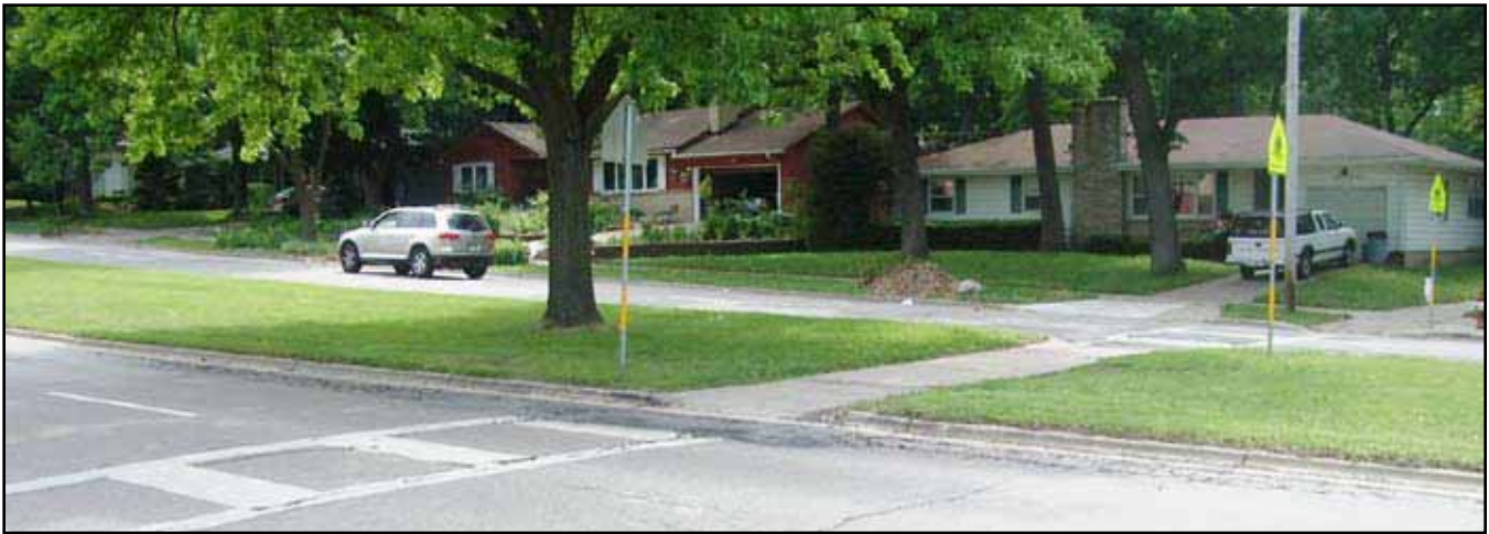
Exhibit 5-58: On busy roadways where pedestrians may have to complete a two-stage crossing, raised medians should be provided as a safe place to wait and check for traffic.
