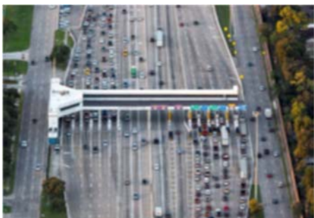
Toll Plaza with ORT Lanes and Cash Collection Lanes
