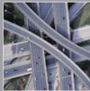
Toronto, Canada's 407 ETR The world's first all-electronic, barrier-free toll highway opens.
