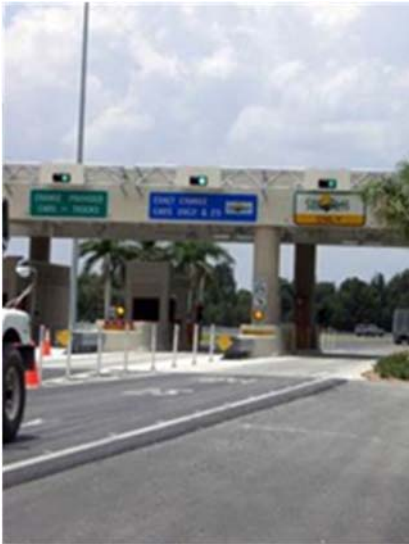
Toll Plaza with ETC Lanes and Cash Collection Lanes
