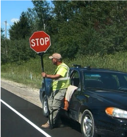
Flagger leaning on car without an escape route
