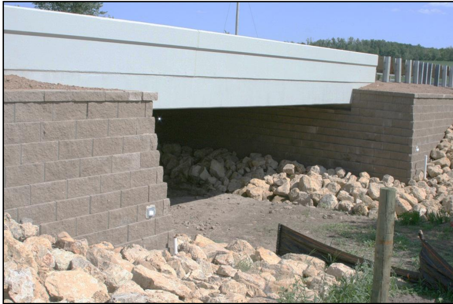
Figure 7.1-4 GRS-IBS Structure
