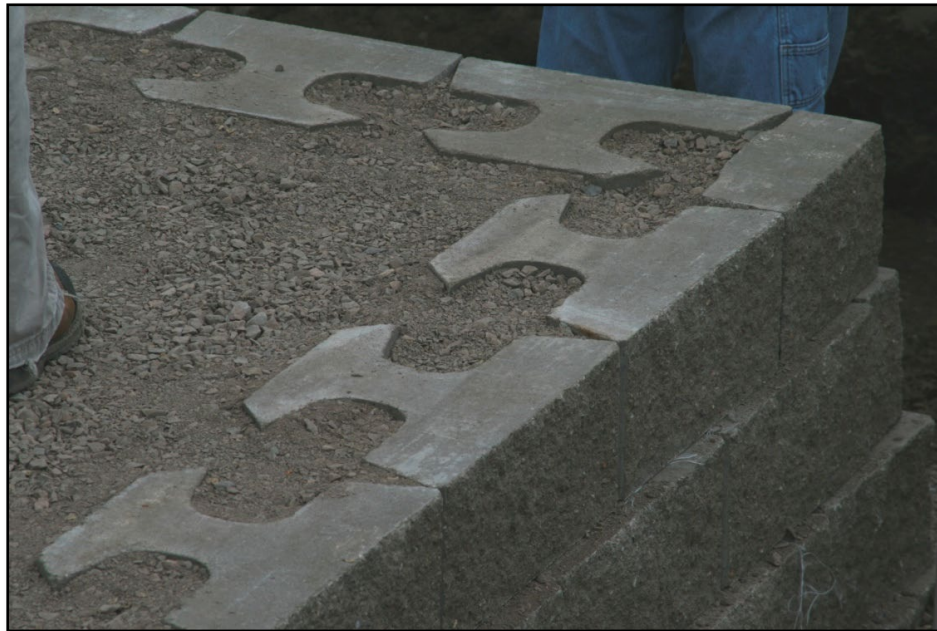
Figure 7.1-5 GRS Abutment Layer During Construction
