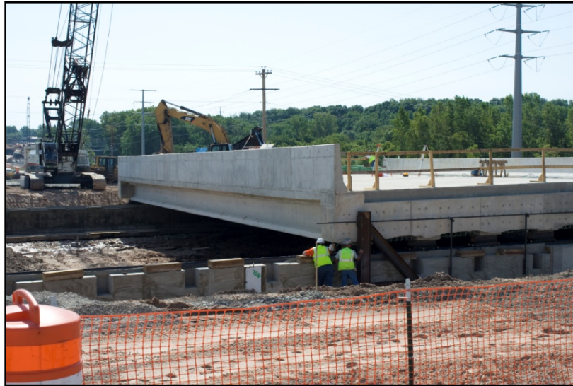
Figure 7.1-6 Lateral Sliding
