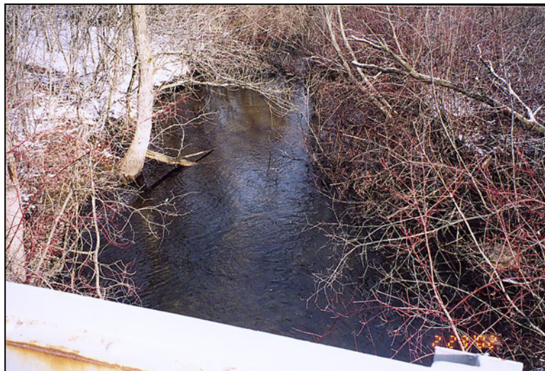
Figure 2.8.2.2-3: Heavily Vegetated Downstream Channel.
