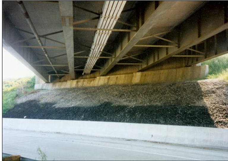
Figure 2.5.1.1-2: Reinforced Concrete Sill Abutment
