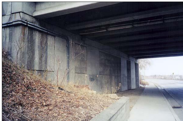
Figure 2.5.3.3-3: Reinforced Concrete Abutment - Condition State 1
