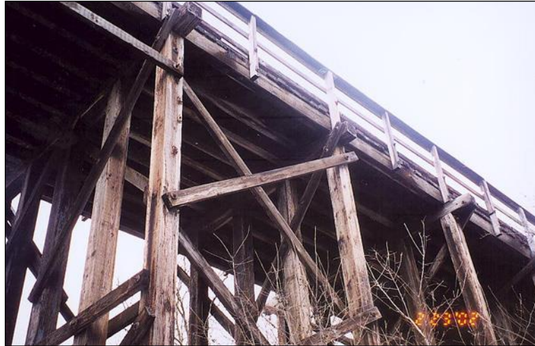
Figure 2.5.5.1-1: Timber Pier Columns
