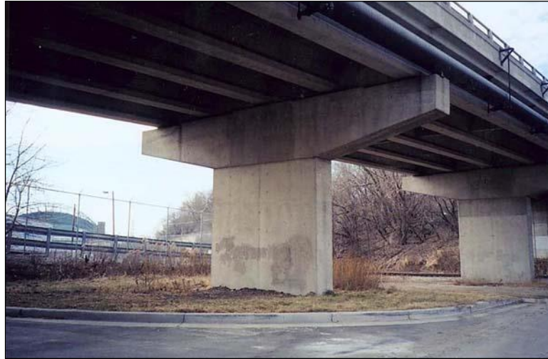
Figure 2.5.1.2-4: Hammerhead Pier
