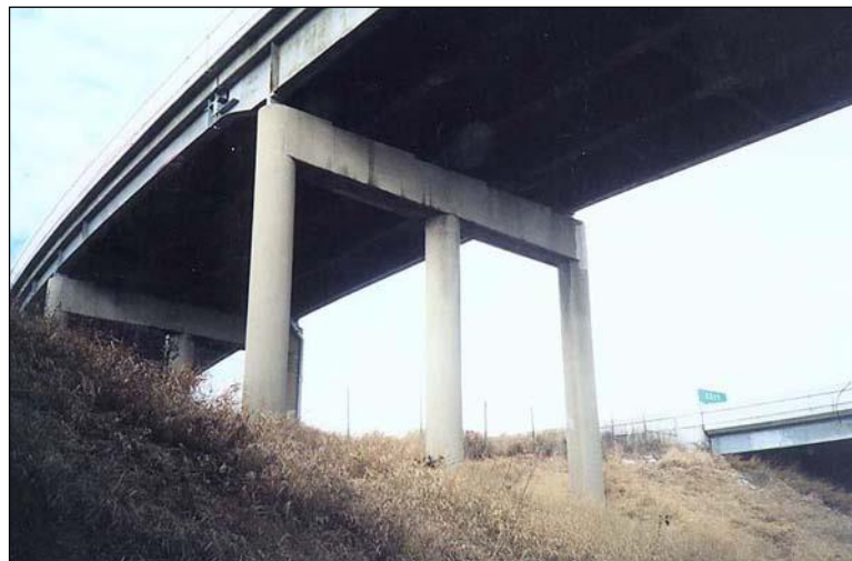
Figure 2.5.1.2-3: Reinforced Concrete Columns and Pier Cap
