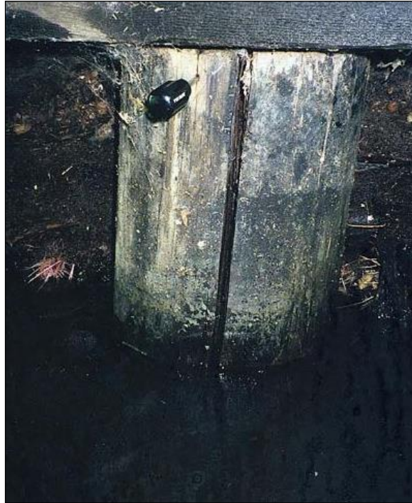
Figure 2.5.5.5-3: Split Timber Pile - Condition State 3
