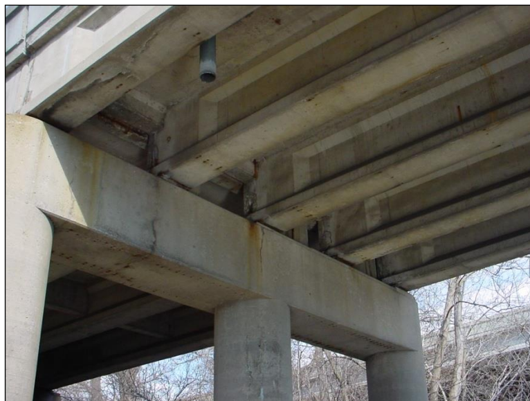
Figure 2.5.3.6-1: Reinforced Concrete Pier Cap
