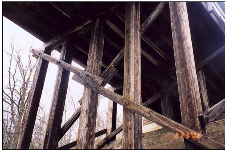
Figure 2.5.5.1-2: Timber Columns, Cap, and Cross-Bracing – Condition State 1
