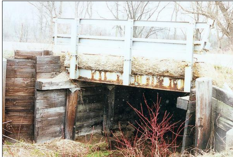
Figure 2.5.4.3-1: Timber Abutment and Wingwalls
