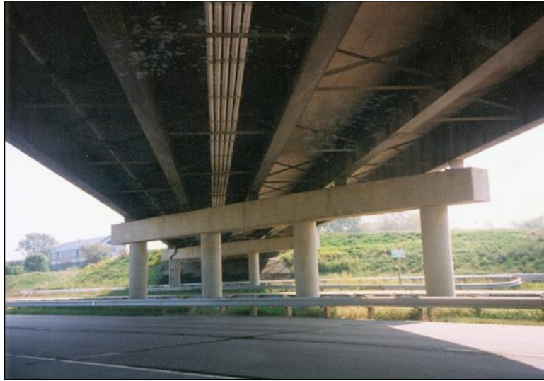
Figure 2.5.3.6-2: Reinforced Concrete Pier Cap - Condition State 1
