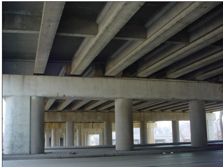
Figure 2.5.3.1-1: Reinforced Concrete Multi Column Piers
