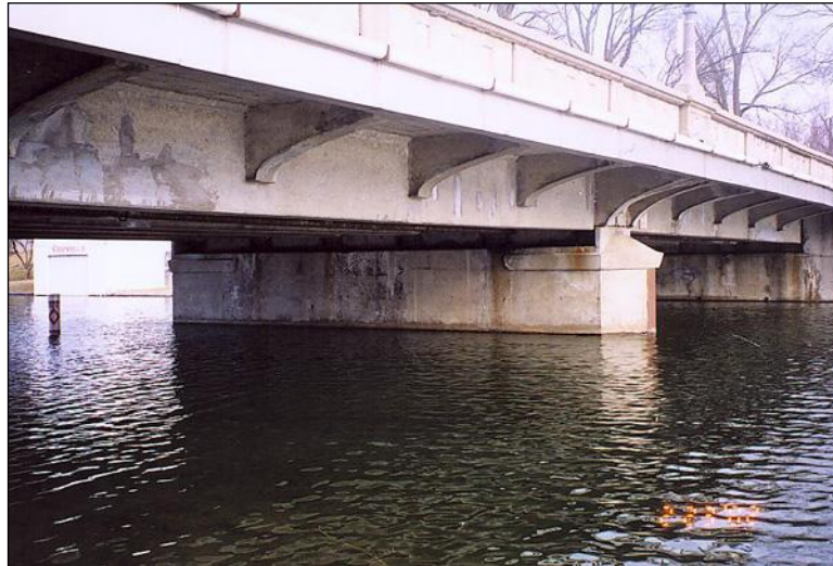
Figure 2.5.3.2-1: Reinforced Concrete Pier Wall
