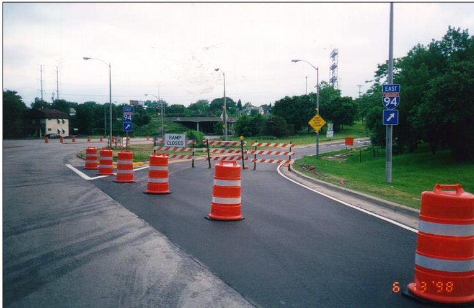
Figure 1.4.8.1-1: Barrels Channel Traffic Away From Work Zone.
