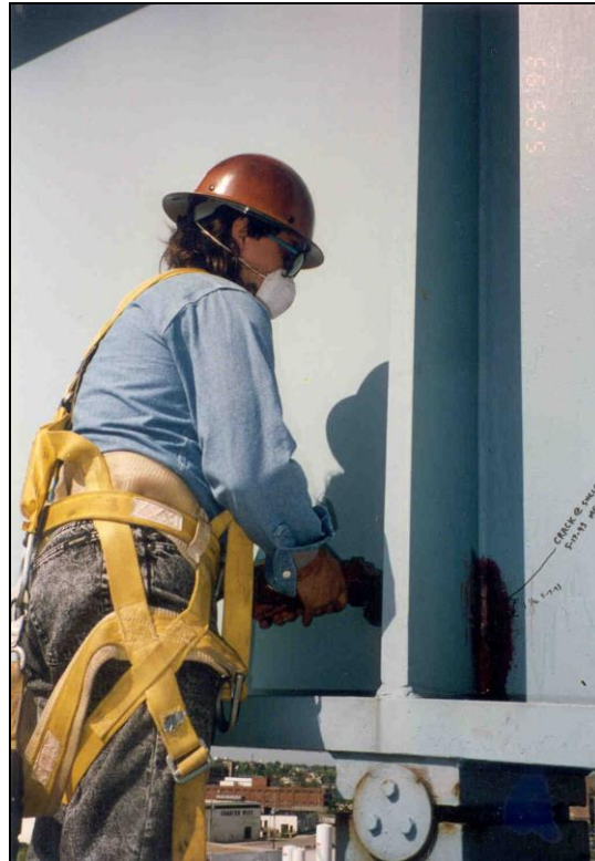
Figure 1.4.4.6-1: Body Harness/Tie-Off.
